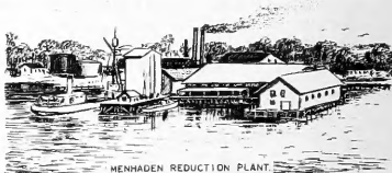
MENHADEN REDUCTION PLANT
