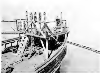
Fig. 10 - Mounting of the harpoon gun on the Dennis Gayle .
