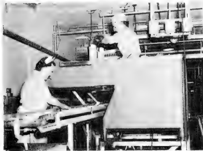
Fig. 7 - Frozen fish slabs fed into the guillotine cutter are sliced into individual fish sticks, which drop on to the conveyor belt for processing.
