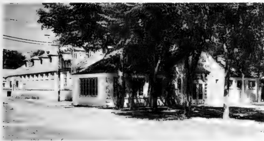
Fig. 1 - Main building Hormel Institute of University of Minnesota, Austin, Minn.
