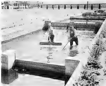
FIG. 2 - TROUT PONDS AND HATCHERY BUILDINGS AT FISH CULTURAL STATION. THE PONDS ARE BEING CLEANED.
