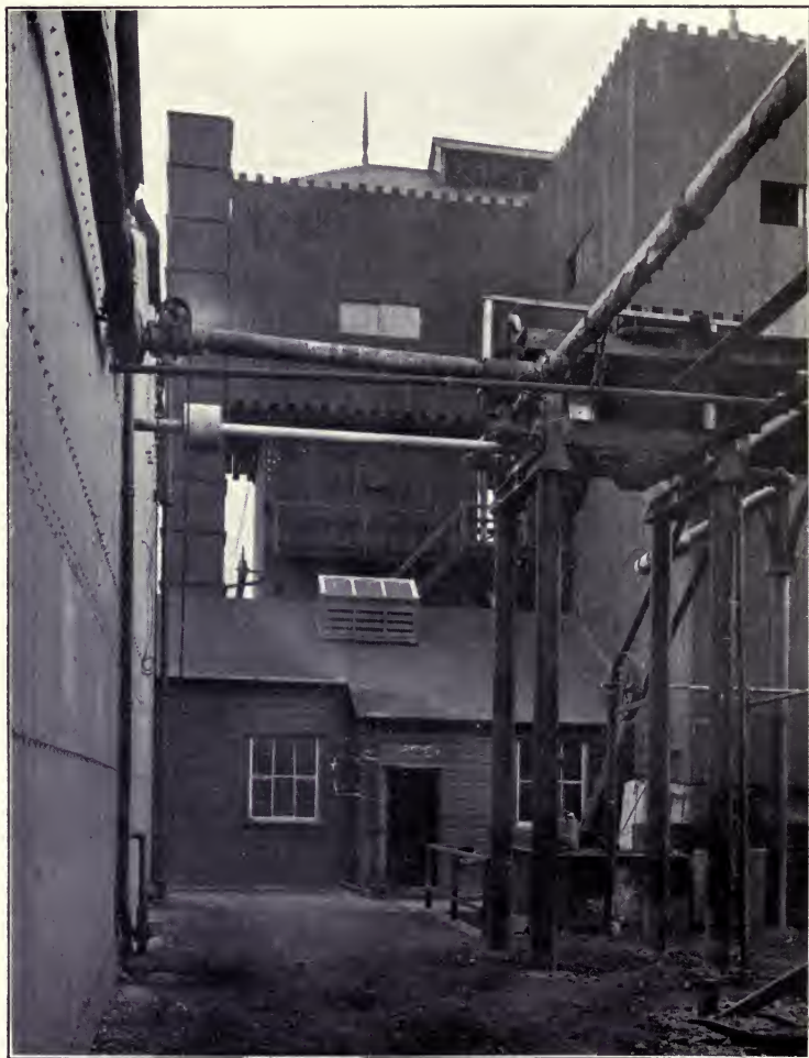
FIG. 4.—View of the Acid Towers.
