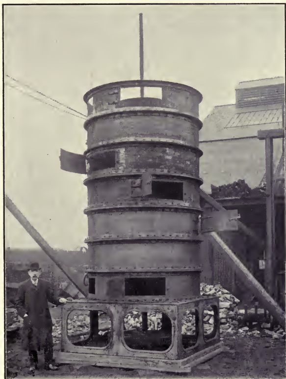
FIG. 50.—Lennox's Patent Continuous Automatic Peat-drying Machine.
