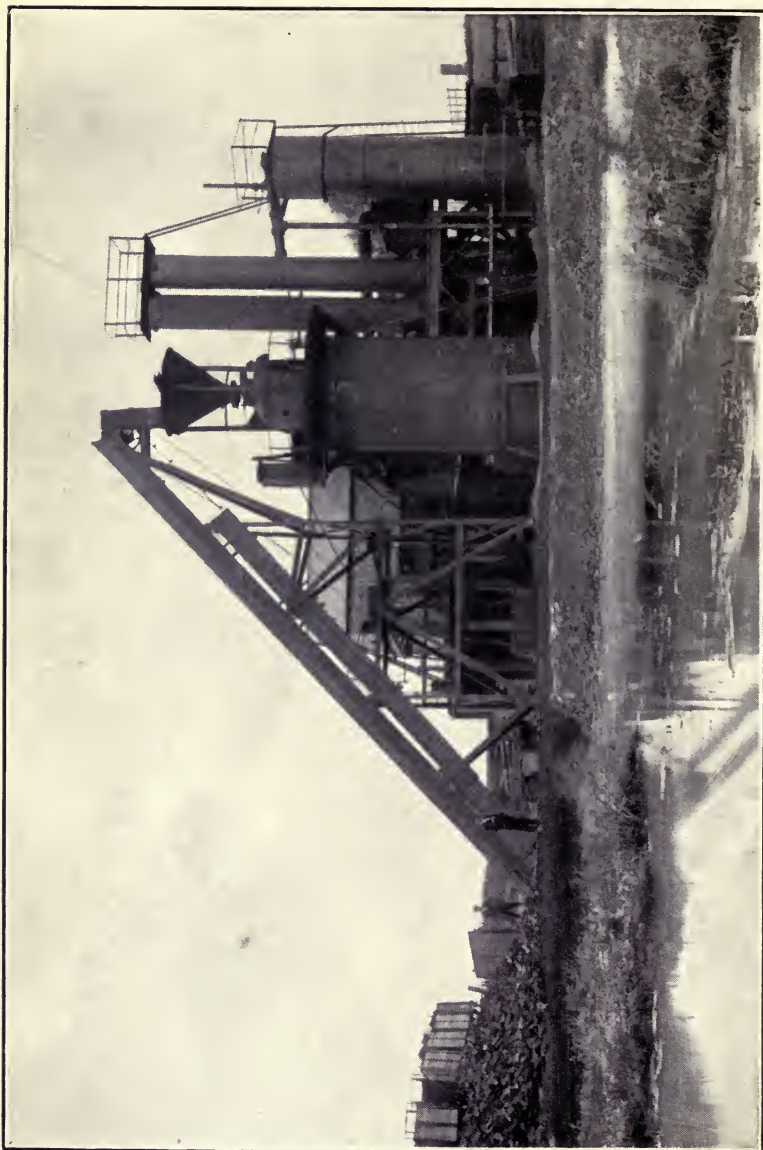
The first producer plant in the world making regularly sulphate of ammonia and producer gas from wet peat. N.B. —Peat may be used containing up to 75 per cent. water. (See page 156.)
