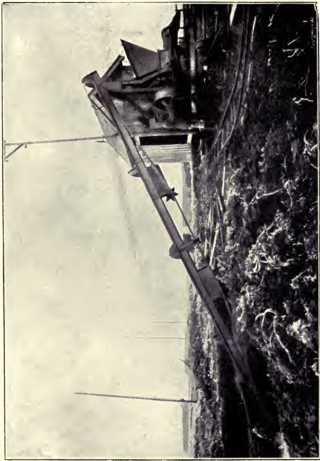
FIG. 12. — Electrically-driven Elevator and Peat-Press.
