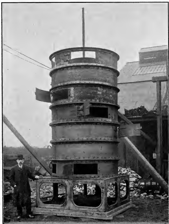
FIG. 50.—Lennox's Patent Continuous Automatic Peat-drying Machine.
