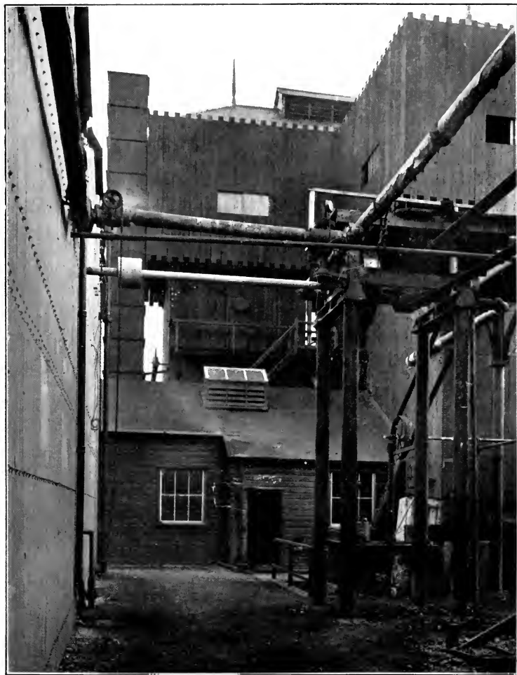
FIG. 4.—View of the Acid Towers.
