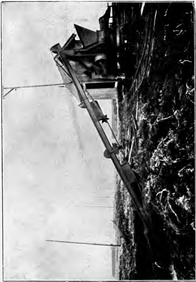
FIG. 12.—Electrically-driven Elevator and Peat-Press.
