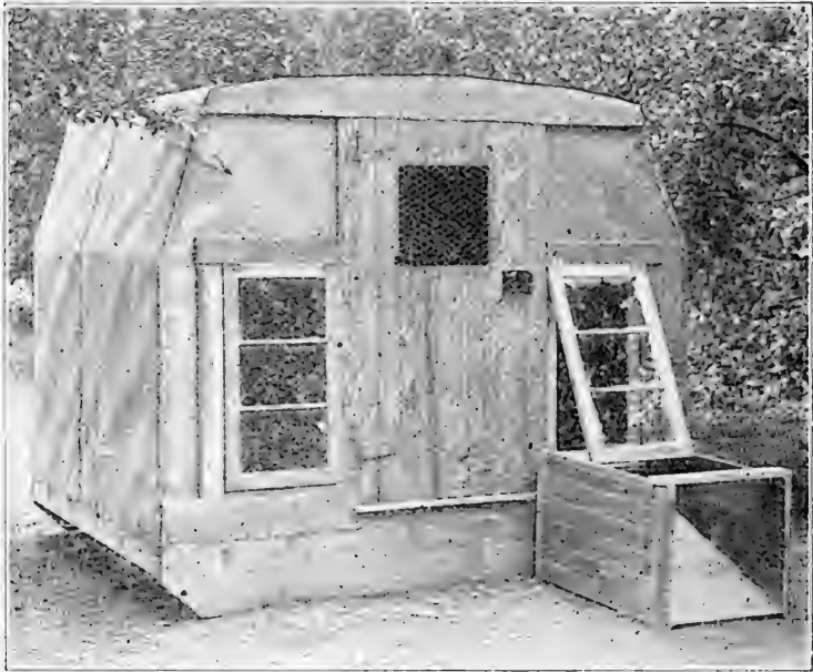
Fig. 217.—Growing coop for young stock constructed from piano cases covered with tar paper. Note runway in front of right-hand window.
