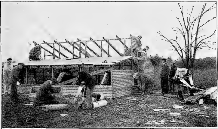
Fig. 78.—Poultry house under construction by students at Purdue University.
