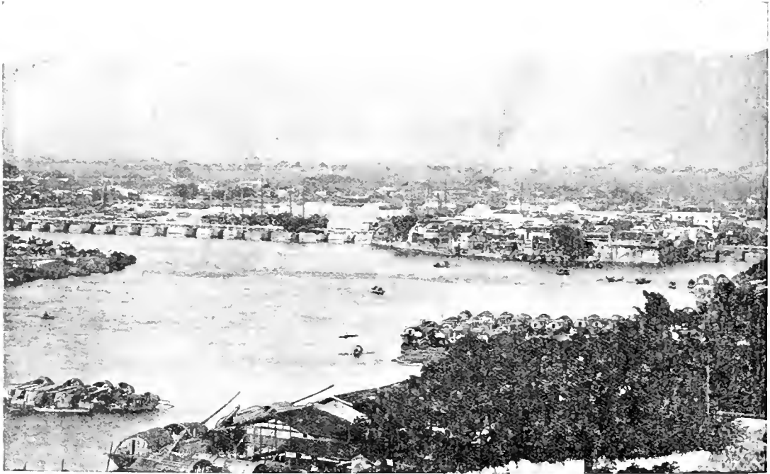
WAN SHUO BRIDGE, FOOCHOW
