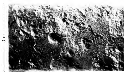
MILD STEEL (F 8) EXPOSED TO COMPLETE IMMERSION IN SEA-WATER AT AUCKLAND FOR 10 YEARS, SHOWING PITTING.
