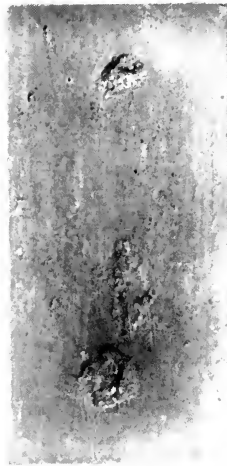
3 in. 13·5 PER CENT. CHROMIUM STEEL (J 8) EXPOSED TO COMPLETE IMMERSION IN SEA-WATER AT AUCKLAND FOR 10 YEARS, SHOWING LOCALIZED CORROSION.
