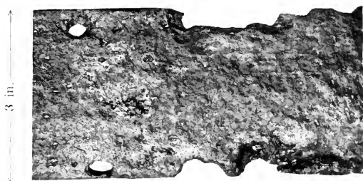
INGOT IRON (M 11) EXPOSED TO AERIAL CORROSION AT COLOMBO FOR 10 YEARS.
