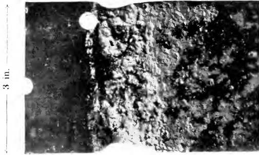
3.75 PER CENT. NICKEL STEEL (K 23) EXPOSED TO HALF-TIDE CONDITIONS AT HALIFAX FOR 10 YEARS, SHOWING DEEP CORROSION AT CONCRETE LEVEL.
