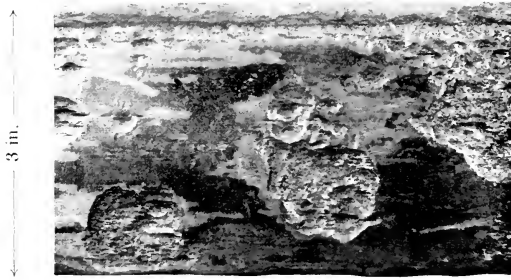
MILD STEEL (F 38) EXPOSED TO COMPLETE IMMERSION IN FRESH WATER AT PLYMOUTH FOR 10 YEARS, SHOWING OYSTER-LIKE PITTING AND CHANNELLING NEAR TOP EDGE.
