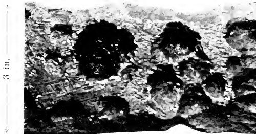
0.635 PER CENT. COPPER STEEL (G 14) EXPOSED TO HALF-TIDE CONDITIONS AT COLOMBO FOR 10 YEARS, SHOWING FACE.
