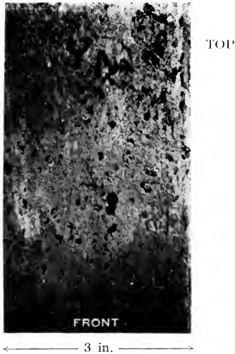
13·5 PER CENT. CHROMIUM STEEL (J 25) AFTER COMPLETE IMMERSION IN SEA-WATER AT HALIFAX FOR 5 YEARS, SHOWING PIN-HOLE PITTING.
