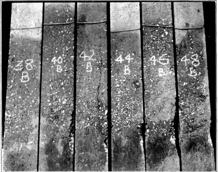
LEAN MIXTURE OF HIGH ALUMINA CEMENT (1 : 3 : 6), NORMAL CONSISTENCY, AFTER 4 YEARS IN SEA-WATER AT SHEERNESS.
