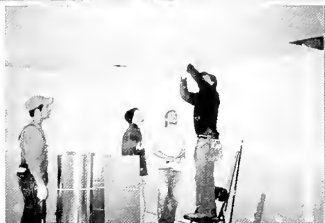
Jesse, Dr. Dan, David, and our facilitator Jeff work on the walls and ceilings, getting them ready to finish and paint.
