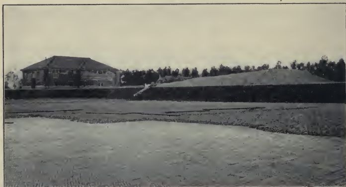
FILTER BED OF THE INDIANAPOLIS WATER WORKS.
