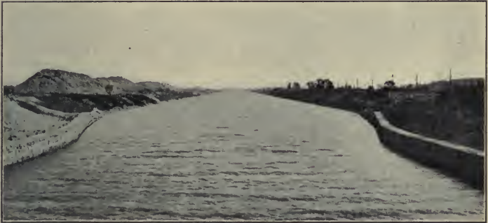
2. A section of the canal where it passes from the solid rock to the soft earth.
