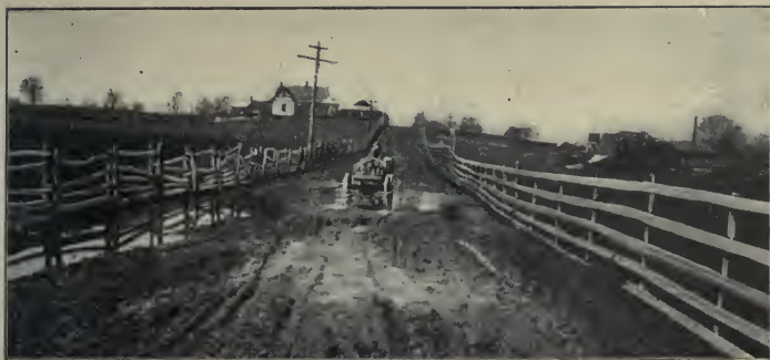
1. The road in its original condition.
