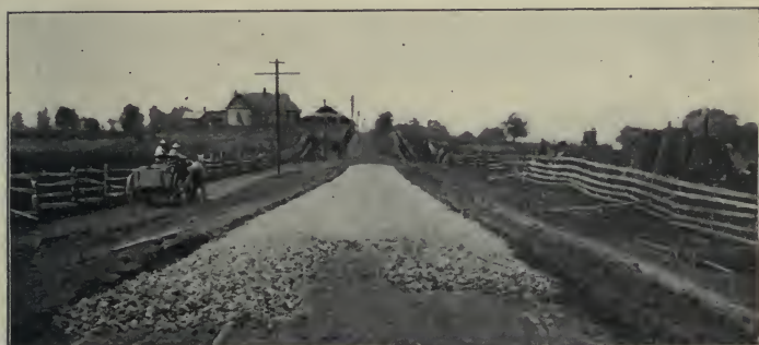
2. Laying the foundation course.
