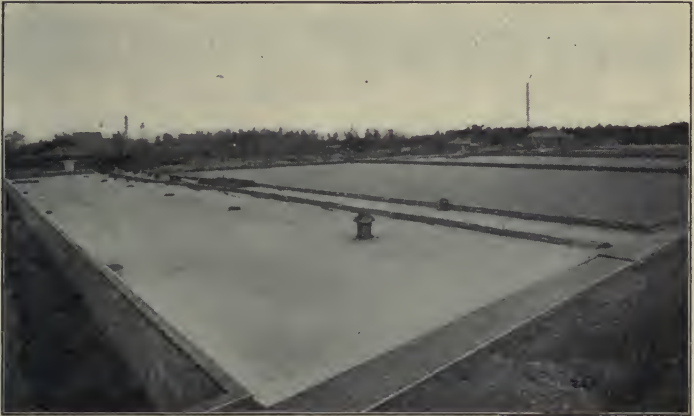
FILTER BEDS OF THE INDIANAPOLIS WATER WORKS.
