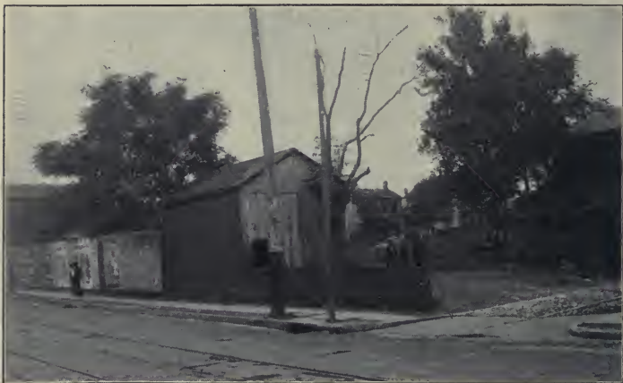
AN UNIMPROVED CORNER.
