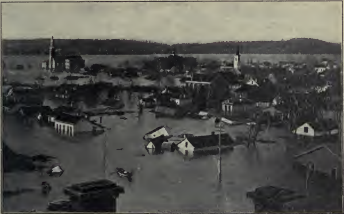
LAWRENCEBURG, IND., DURING THE FLOOD OF THE OHIO RIVER IN 1883.
