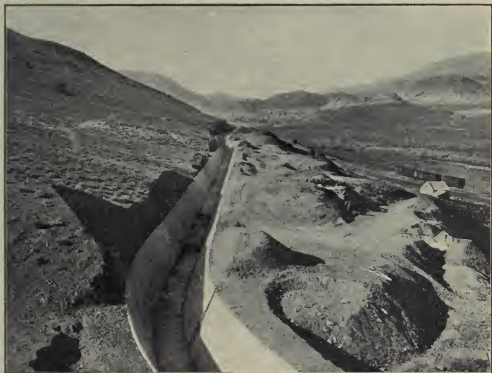
TRUCKEE IRRIGATION CANAL, NEVADA.
