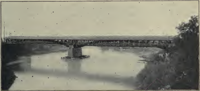
OLD WOODEN BRIDGE ON THE NATIONAL ROAD CROSSING WHITE RIVER, INDIANAPOLIS.
