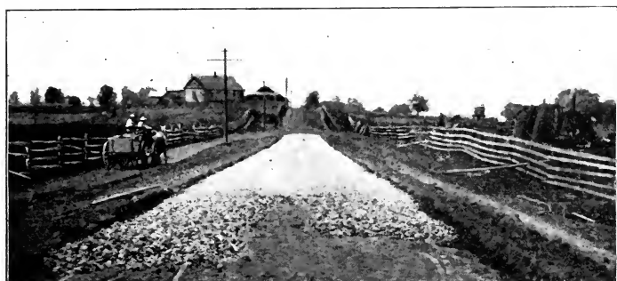
2. Laying the foundation course.
