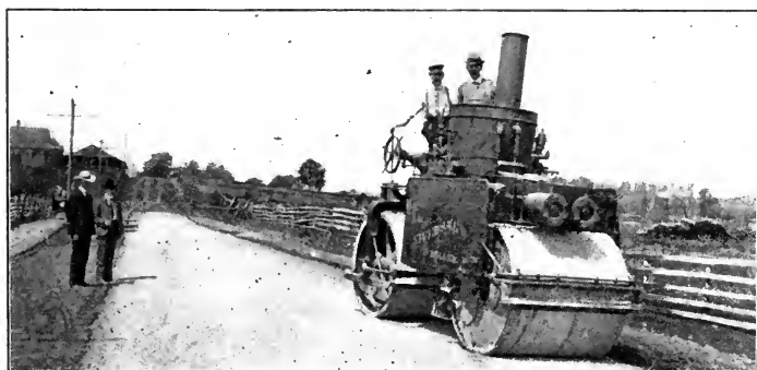
3. Finishing the road.
