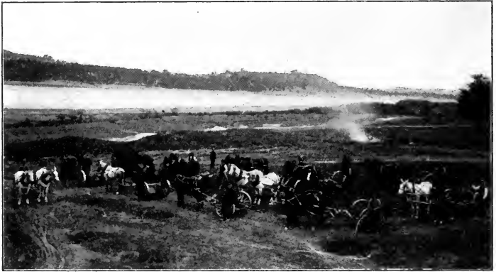
BUILDING THE LEVEE AT LAWRENCEBURG, IND., FOR THE PROTECTION OF THE CITY AGAINST FLOODS.
