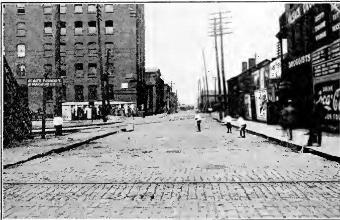
DANGEROUS GRADE CROSSING.
