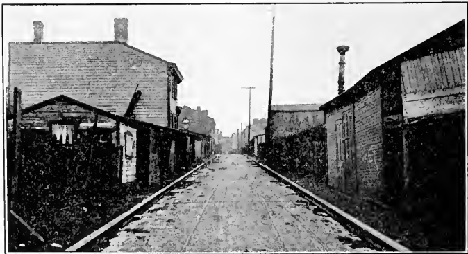
CONCRETE ALLEY PAVEMENT.
