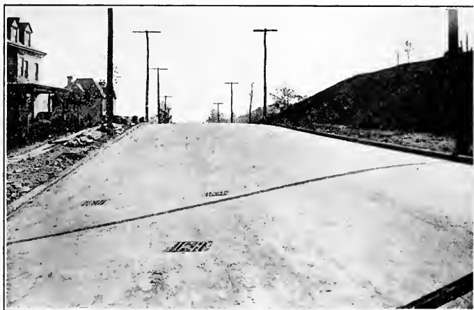
THE SAME STREET AFTER PAVING.
