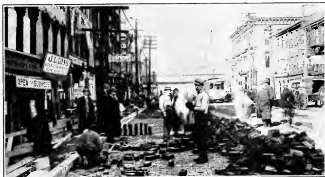
LAYING WOOD BLOCK PAVEMENT.
