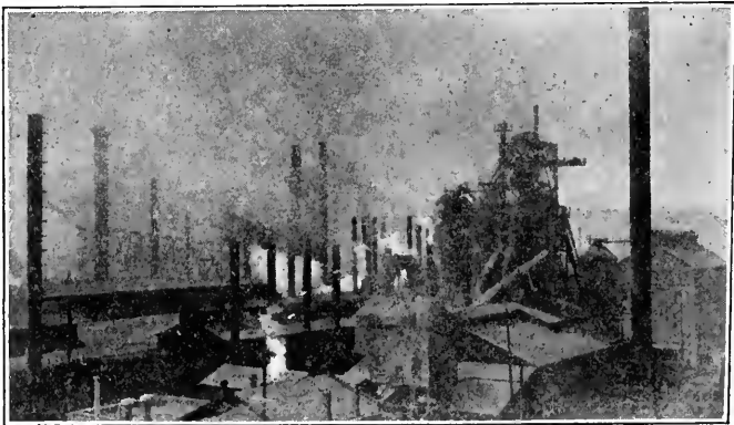
STEEL MILLS, PITTSBURGH.
