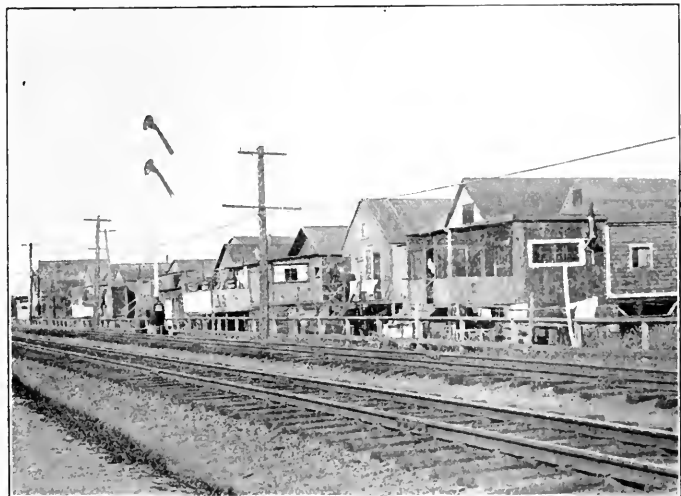
A DANGEROUS FIRE HAZARD.
