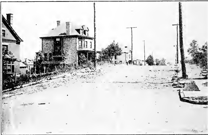
A CITY STREET BEFORE IMPROVEMENT.
