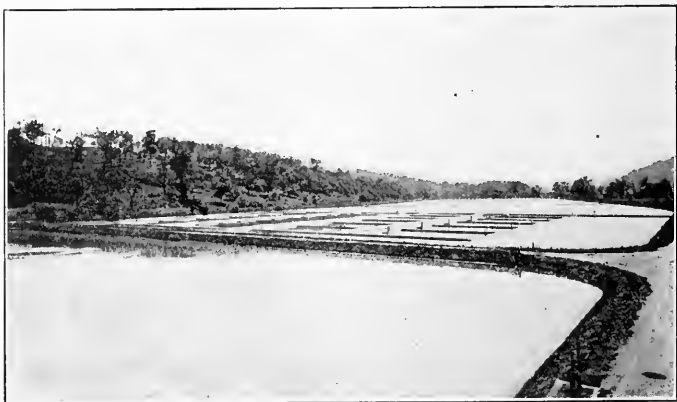
SETTLING BASINS AT A FILTRATION PLANT.
