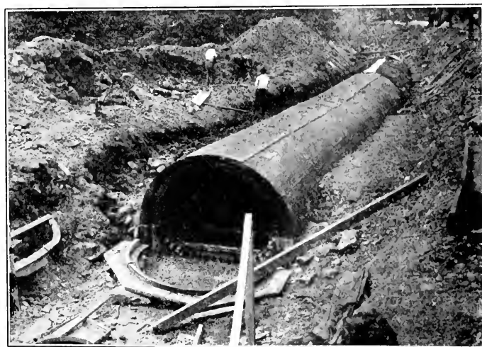
SEWERS UNDER CONSTRUCTION.
