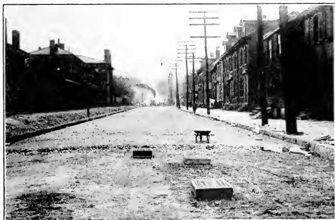
PREPARING THE STREET FOR PAVING.
