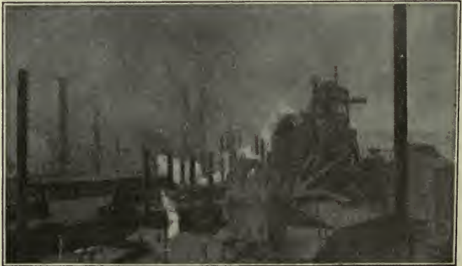
STEEL MILLS, PITTSBURGH.
