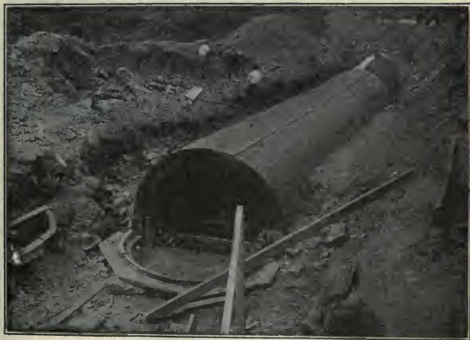
SEWERS UNDER CONSTRUCTION.
