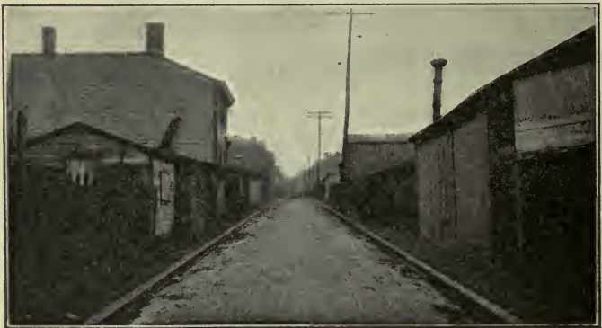
CONCRETE ALLEY PAVEMENT.
