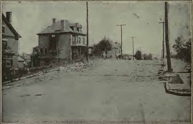
A CITY STREET BEFORE IMPROVEMENT.
