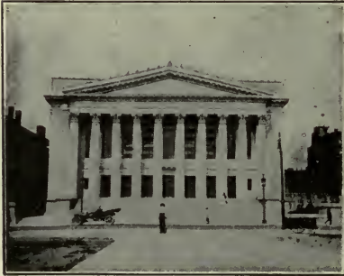
MUNICIPAL BUILDING, SPRINGFIELD, MASSACHUSETTS.
