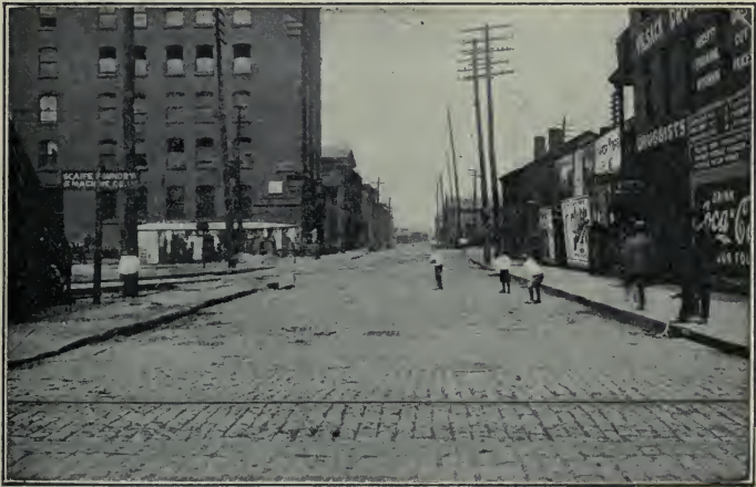
DANGEROUS GRADE CROSSING.
