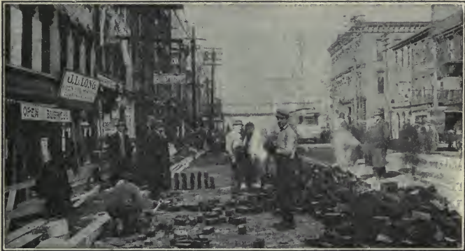
LAYING WOOD BLOCK PAVEMENT
