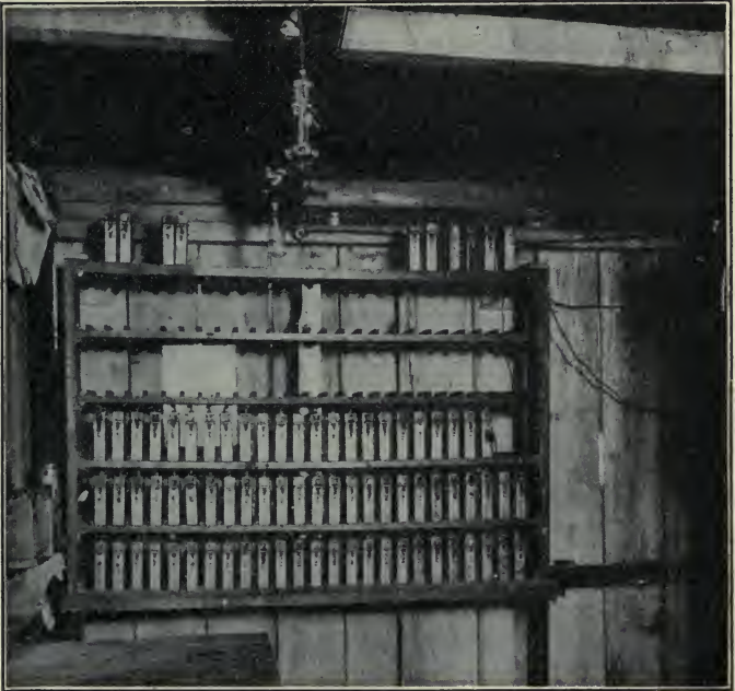
CHARGING BOARD FOR MINERS' LAMPS.
