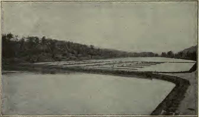
SETTLING BASINS AT A FILTRATION PLANT.
