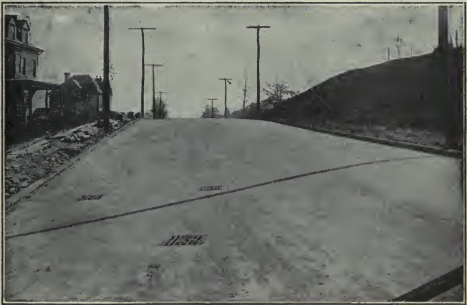
THE SAME STREET AFTER PAVING.
