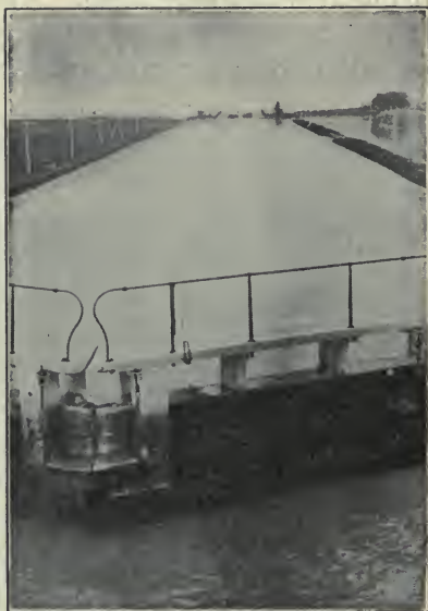
LOCKS IN CANAL AROUND RAPIDS IN THE ST. LAWRENCE RIVER.
