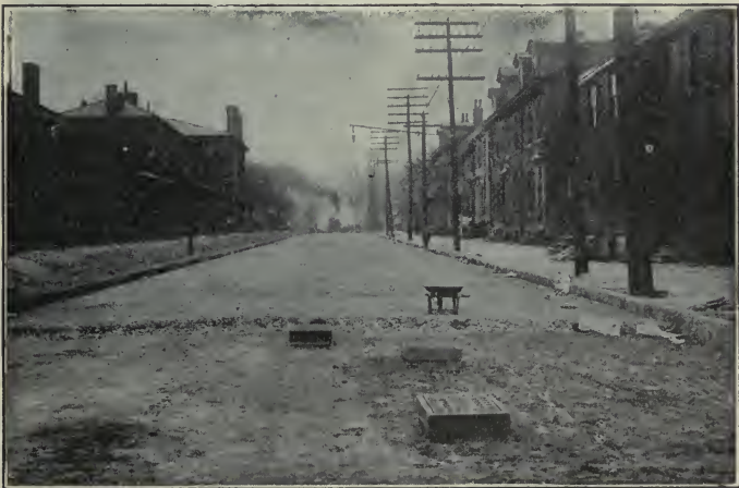
PREPARING THE STREET FOR PAVING.
