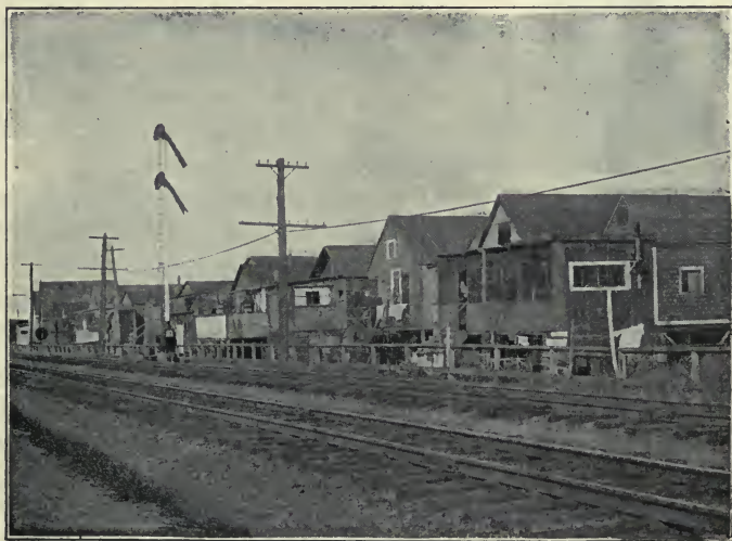
A DANGEROUS FIRE HAZARD.
