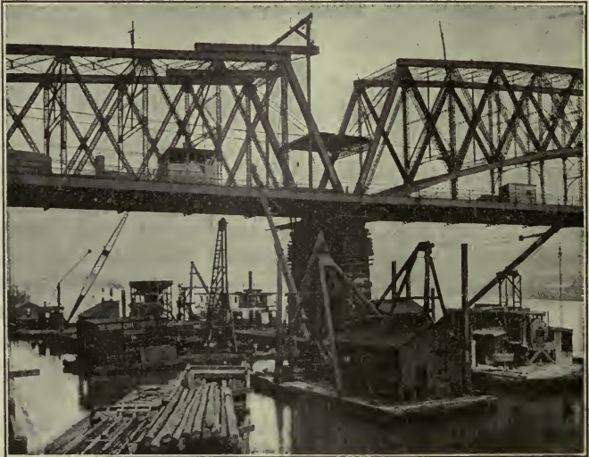
CONSTRUCTION WORK ON A GREAT BRIDGE.
