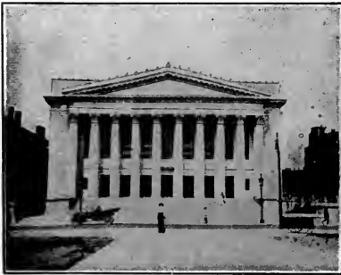
MUNICIPAL BUILDING, SPRINGFIELD, MASSACHUSETTS.
