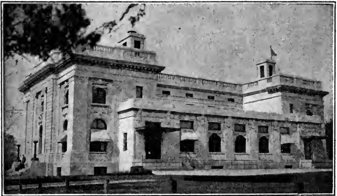
GOVERNMENT BUILDING, NEWPORT NEWS, VIRGINIA.
