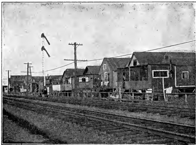
A DANGEROUS FIRE HAZARD.
