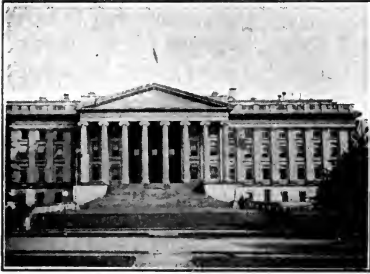
FRONT OF THE TREASURY BUILDING.
