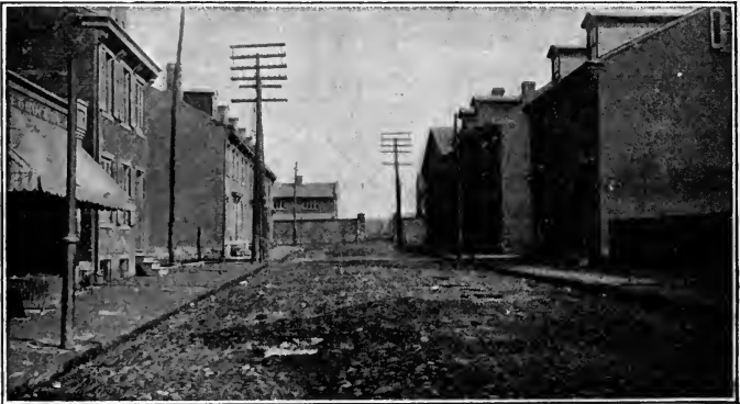
OLD STYLE COBBLESTONE STREET.
