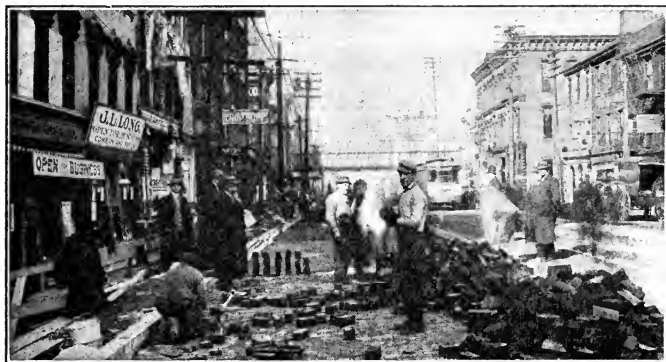
LAYING WOOD BLOCK PAVEMENT
