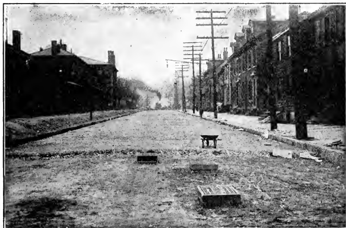
PREPARING THE STREET FOR PAVING.
