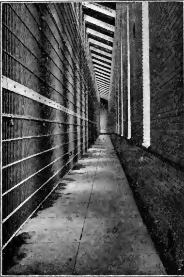
CELL CORRIDOR IN A COUNTY WORKHOUSE.
