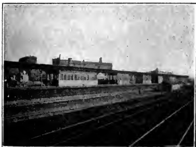
A SUBURBAN STATION PLATFORM AND TRACKS.
