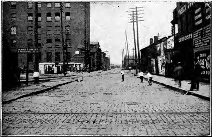
DANGEROUS GRADE CROSSING.
