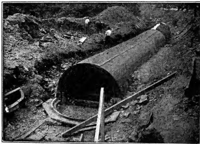
SEWERS UNDER CONSTRUCTION.
