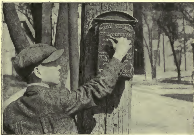
THESE BOXES ARE CONNECTED BY WIRE WITH A CENTRAL EXCHANGE, AND FROM THIS OFFICE THE ALARM IS SENT TO THE COMPANY WHICH IS TO RESPOND
