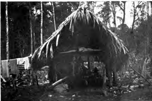
FIG. 3.— A typical shelter among the Lacandones, showing the open ends and the manner in which the sides are protected by the overhanging roof.
