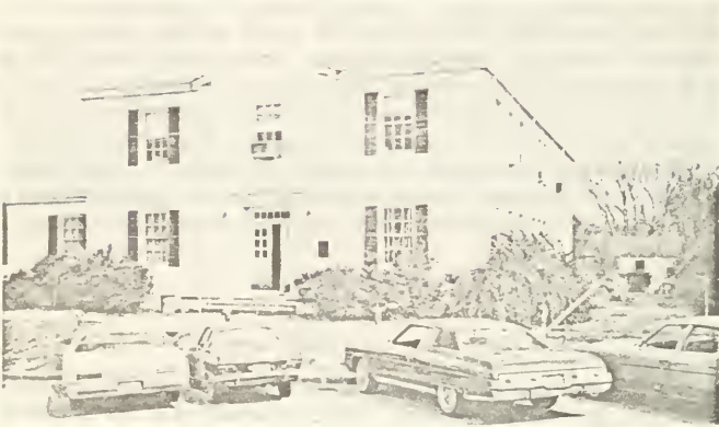
STRUCTURE VIEWED RIGHT-FRONT
