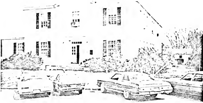
STRUCTURE VIEWED RIGHT-FRONT
