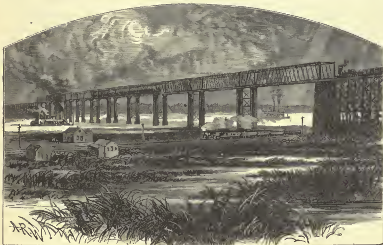
BRIDGE OVER THE MISSOURI AT COUNCIL BLUFFS.
