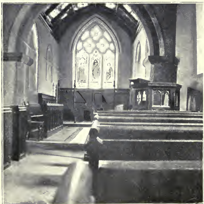
Sullington Church (interior).
