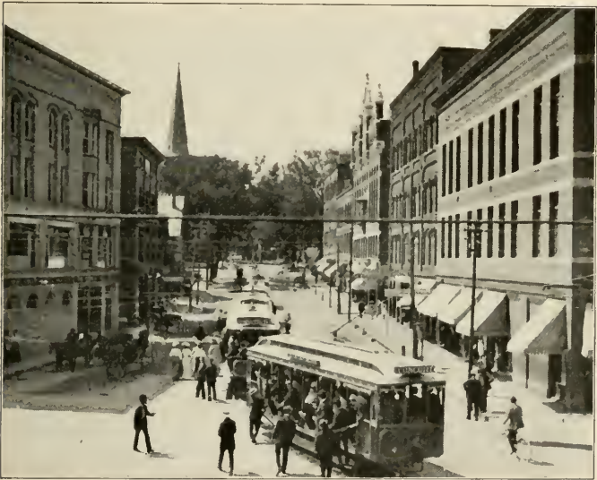
Looking Up Pleasant Street
