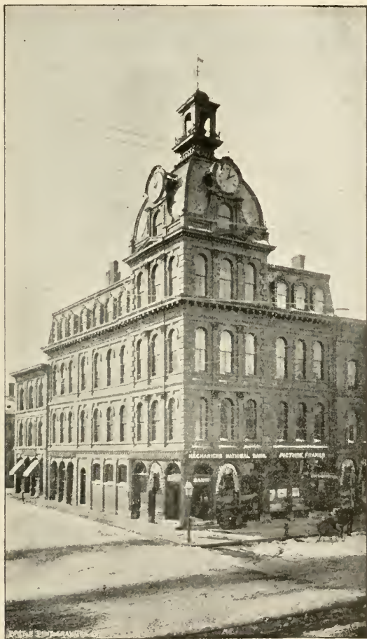
Mechanicks' National and Merrimack County Savings Bank
