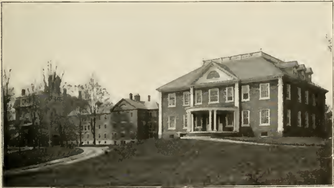
State Hospital Buildings
