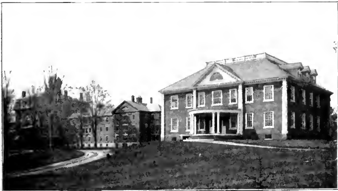
State Hospital Buildings
