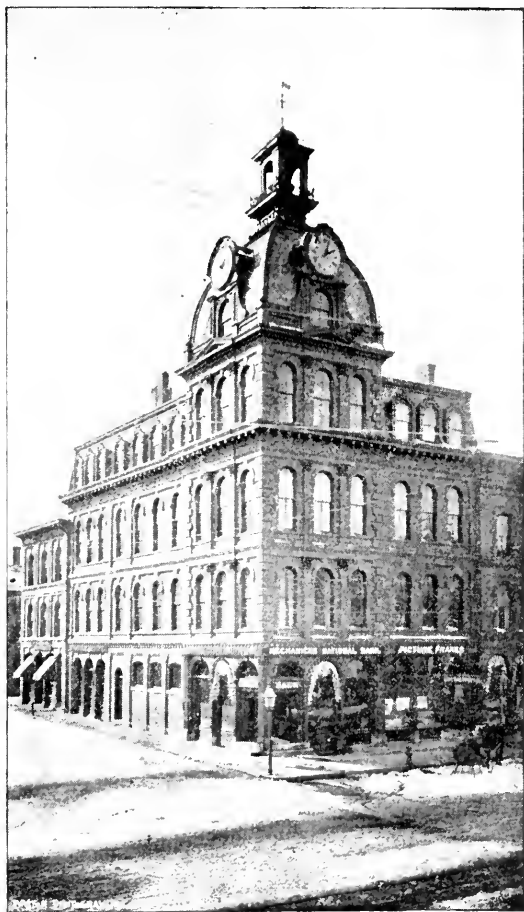
Mechanicks' National and Merrimack County Savings Bank
