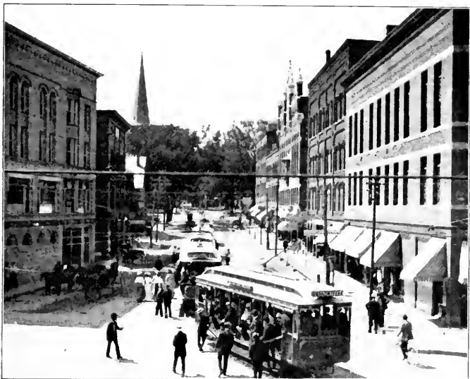
Looking Up Pleasant Street
