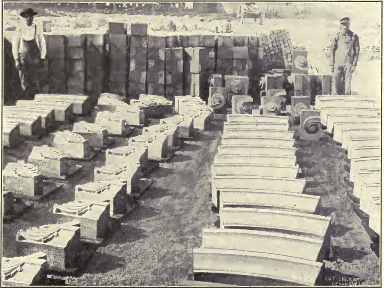
FIG. 12.—Ornamental Work for Chicago Drainage-canal Power-house.
