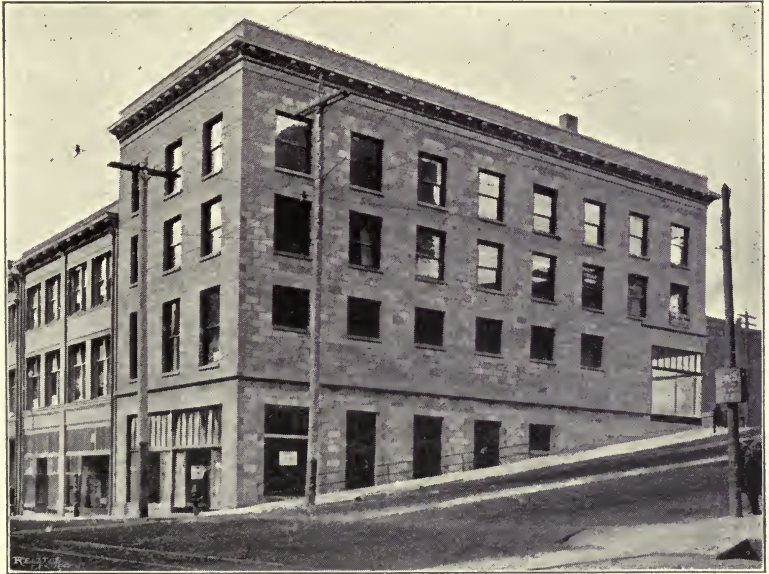
FIG. 33.—Warburton Building, Tacoma, Washington.
