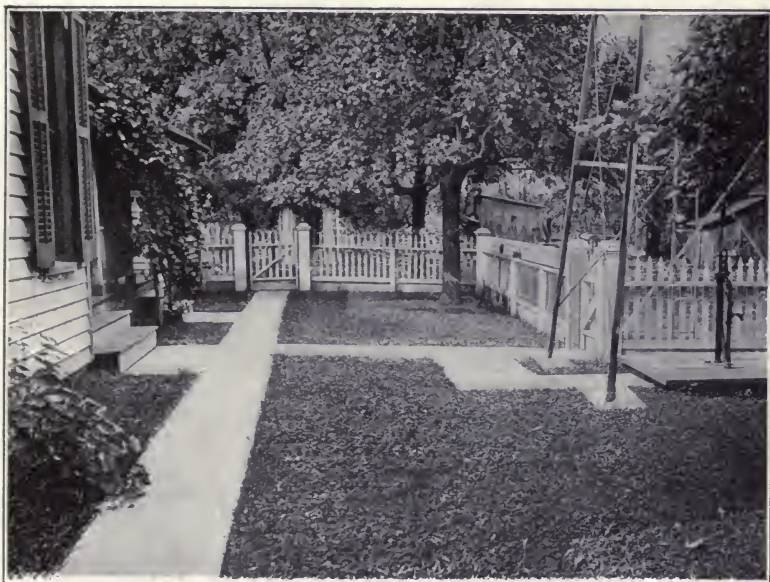
Photo No. 224. CONCRETE WALK AND WINDMILL FOUNDATION, CLINTON, IA.
