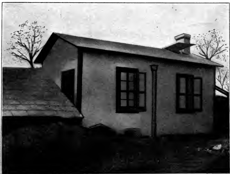
STUCCO KITCHEN ON THE ATLAS PORTLAND CEMENT CO.'S FARM, NORTHAMPTON, PA.
