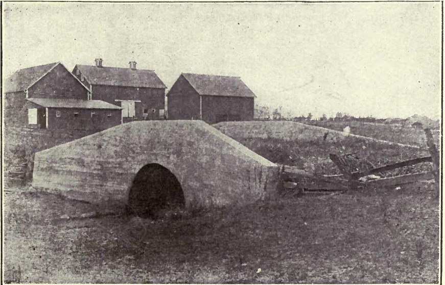
CULVERT AT MORTON, ILL.
