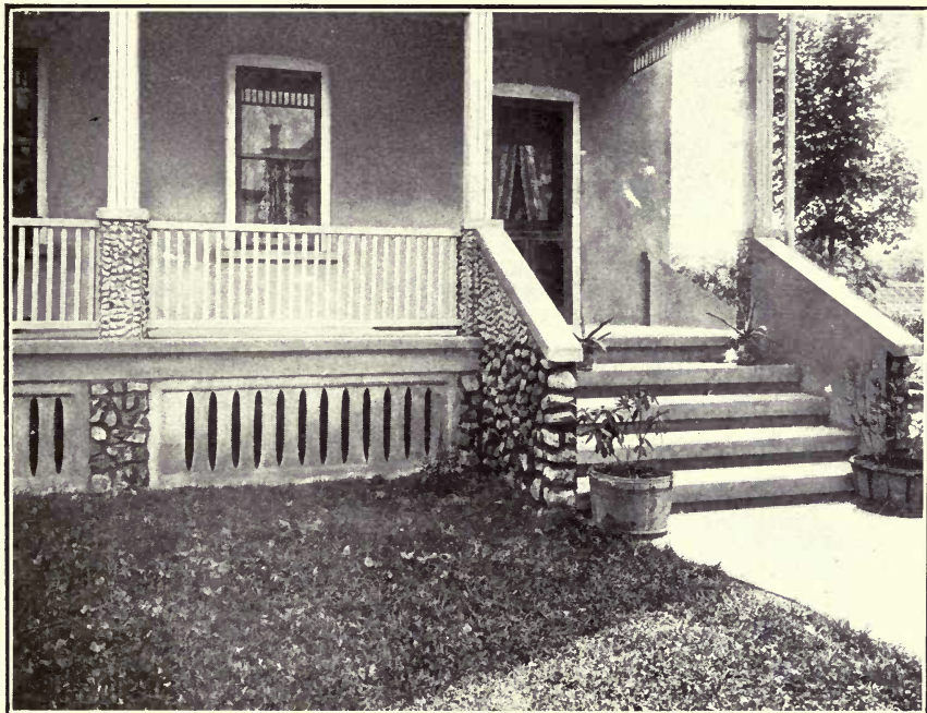
CONCRETE PORCH STEPS AND LATTICE AT WESTWOOD, N. J.
