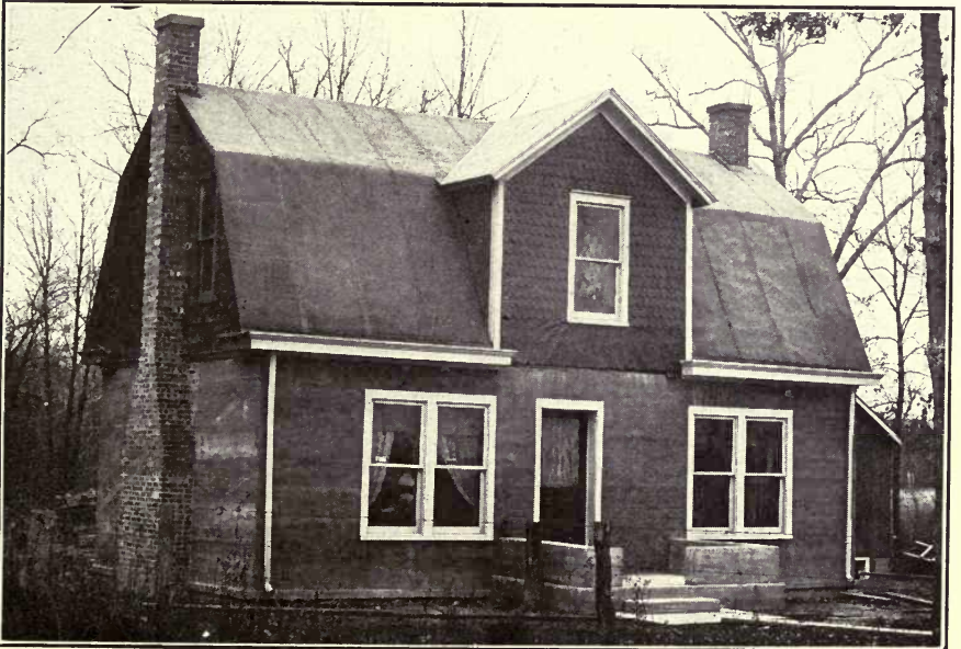
CONCRETE HOUSE NEAR MORTON, ILL.
