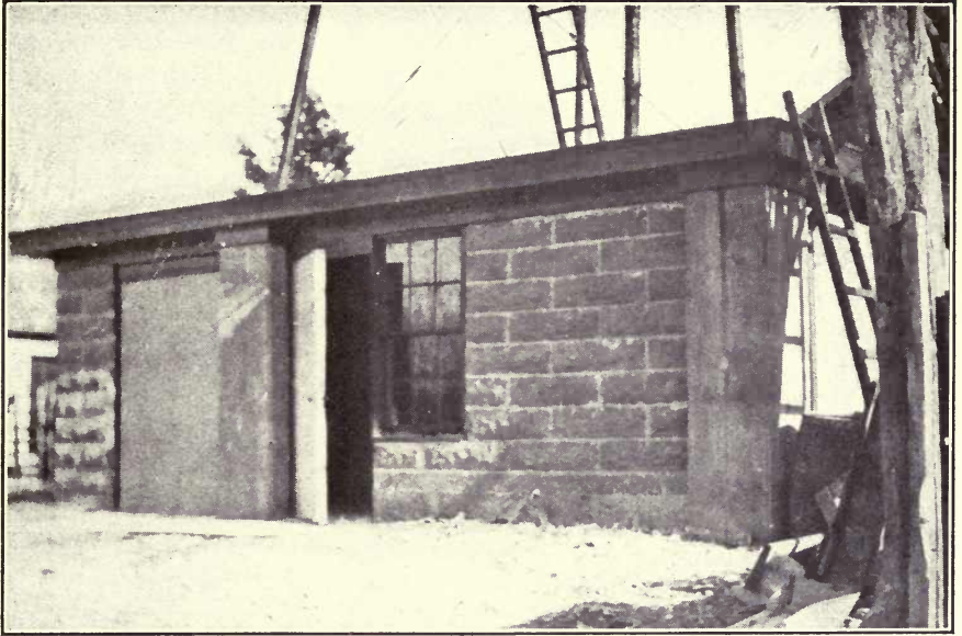
WELL HOUSE WITH HEAVY CONCRETE COLUMNS FOR SUPPORTING STEEL FRAME OF HIGH WATER TANK AT COLUMBIA, MO.
