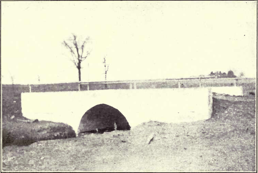
CULVERT AT HARRISTOWN, ILL.
