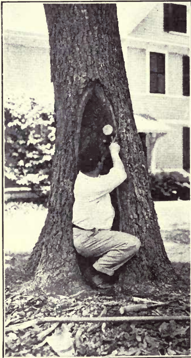
REMOVING DECAYED MATTER FROM TREE BEFORE FILLING
