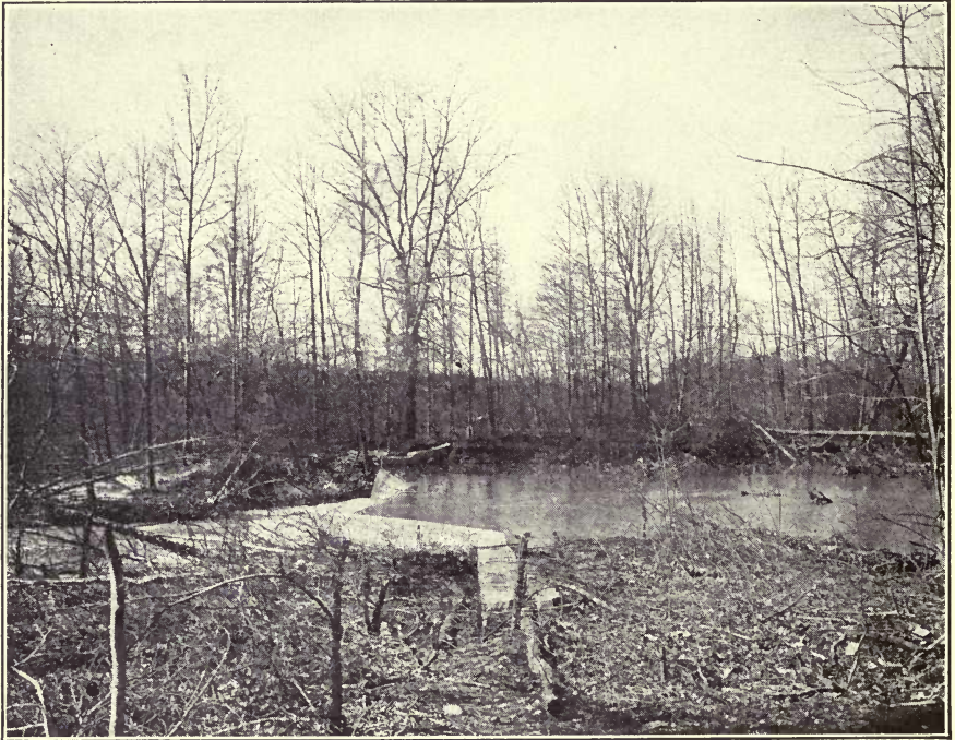
DAM AT ARLINGTON, VA.
