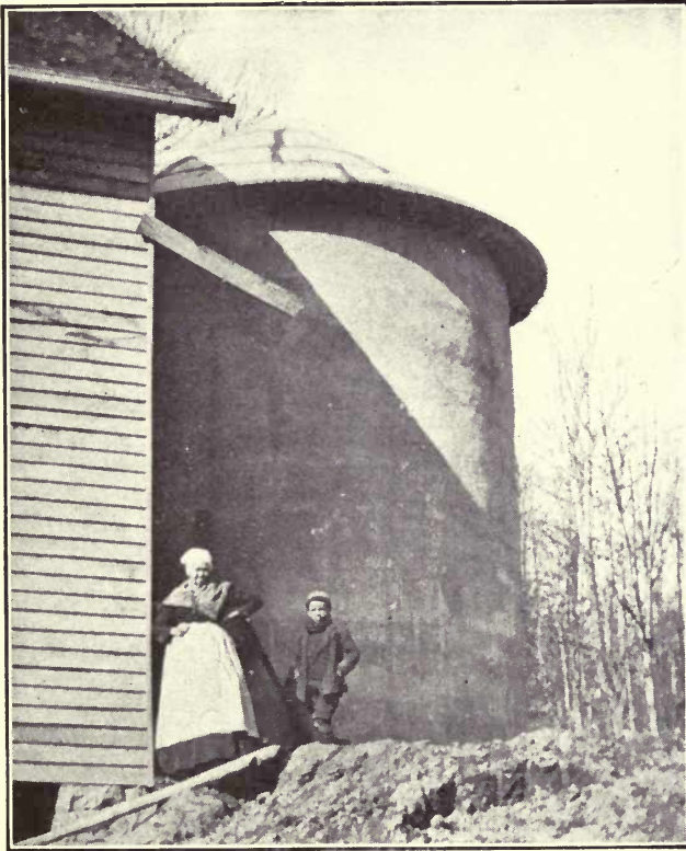
CONCRETE SILO AT CHARLOTTESVILLE. VA.
