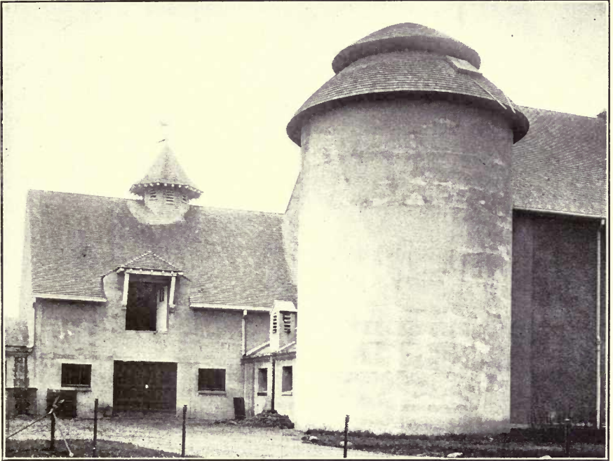
ONE OF THE SILOS AT GEDNEY FARMS, WHITE PLAINS, N. Y.
