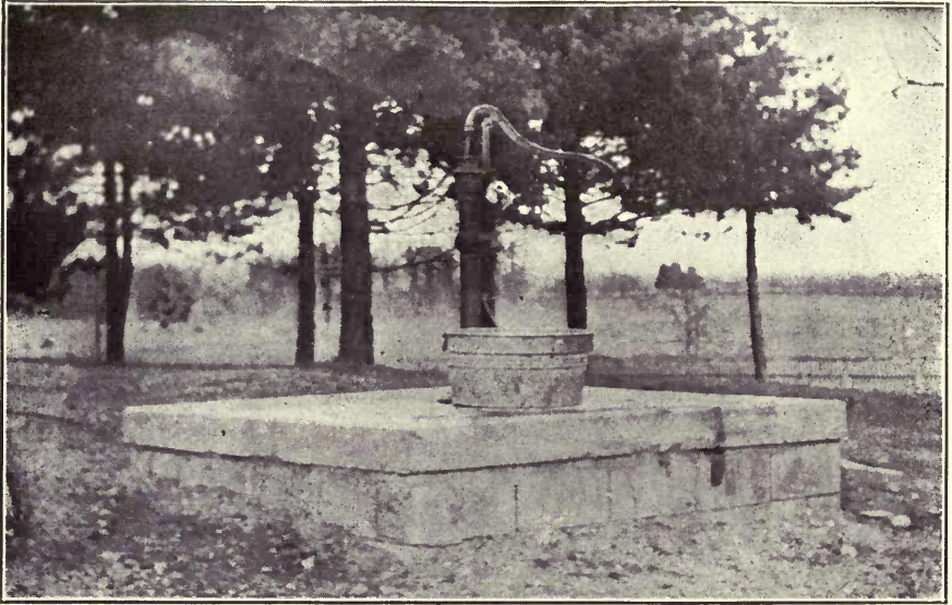
CONCRETE CISTERN COVER, HARRISTOWN, ILL.
