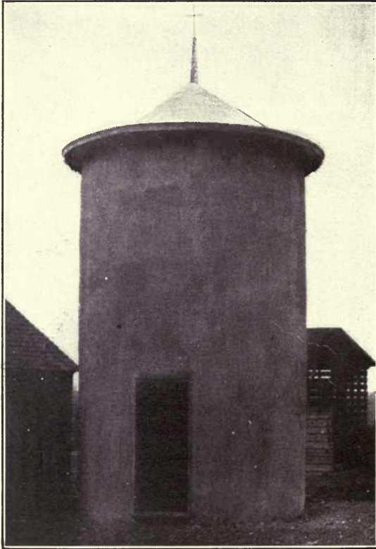
WATER TANK AT MORTON, ILL.
