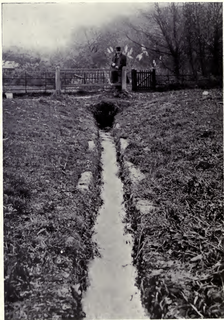
Fig. 37.—STONE DITCH EDGED WITH CONCRETE.
