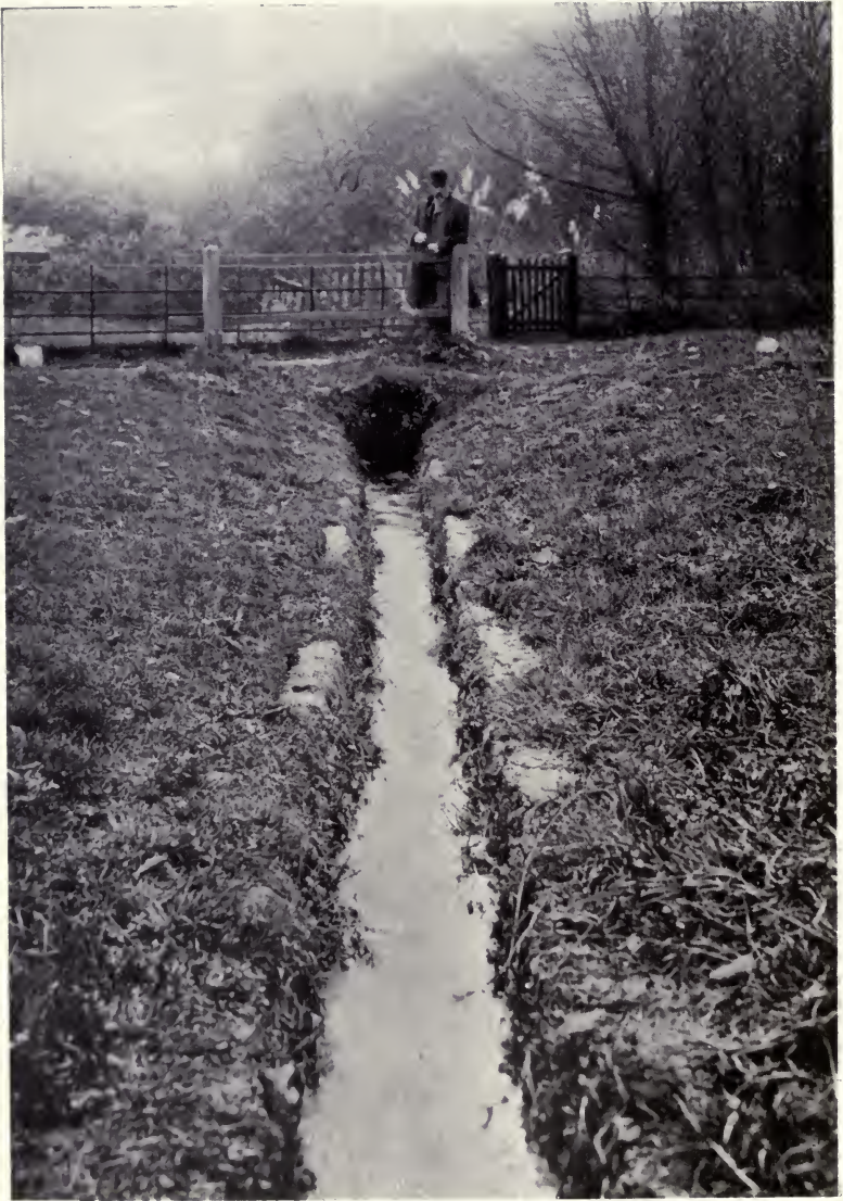
Fig. 37.—STONE DITCH EDGED WITH CONCRETE.
