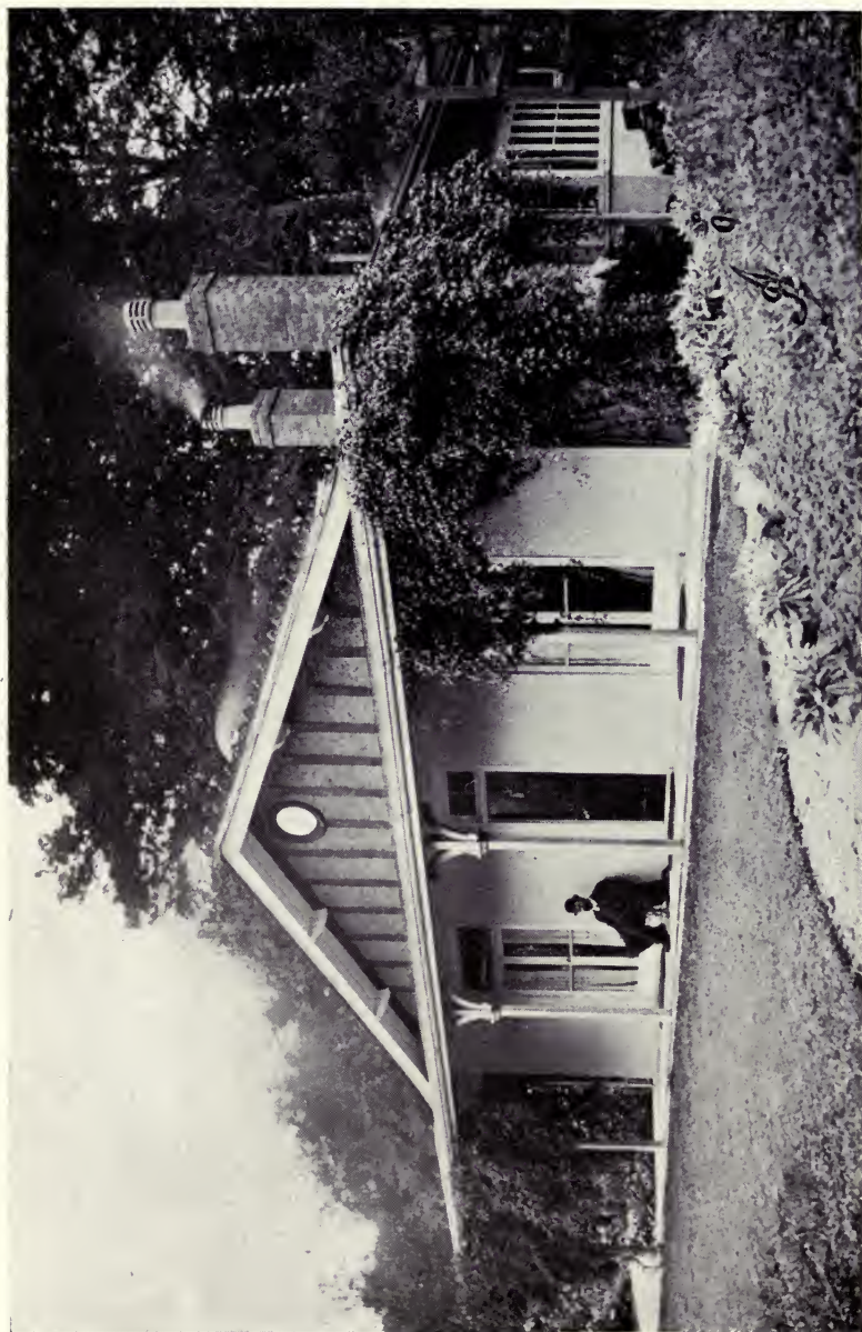
Fig. 48.—A Bungalow, the walls of which are all solid concrete 5" thick. A considerable quantity of barbed wire was used in reinforcing this building. Designed and constructed by Fred Ballard in 1904.
