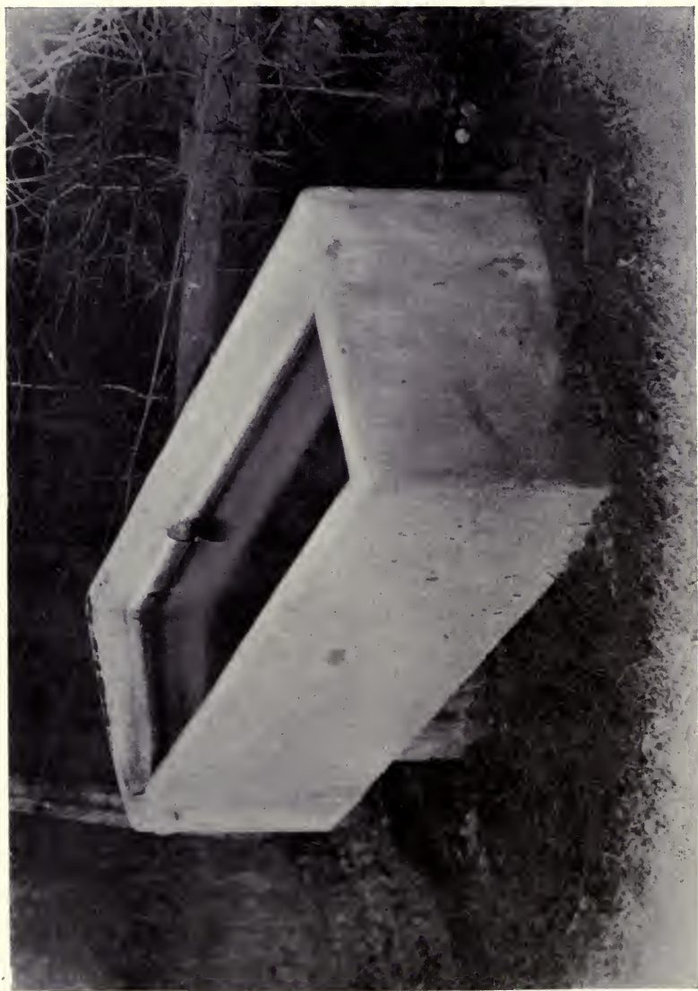
Fig. 38.—CONCRETE DRINKING TANK.
