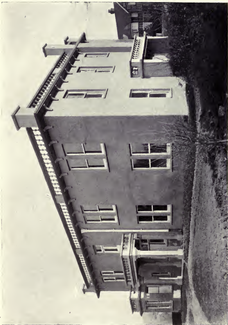
Fig. 44.—House designed by Fred and Beatrice Ballard. Built at Colwall for Miss Kissel. Concrete roof on brick walls.
