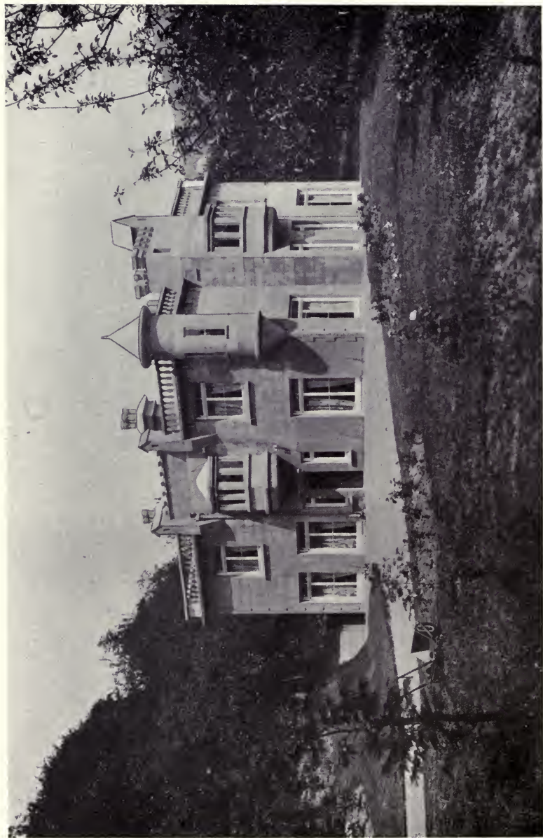
Fig. 45.—House built with brick, covered with cement plaster. Floors and roof of reinforced concrete. \frac{1}{8} " square indented bar used in spans up to 15'. The bay windows extend 4' beyond the perpendicular of the walls. Designed and built by F. and B. Ballard in 1909.
