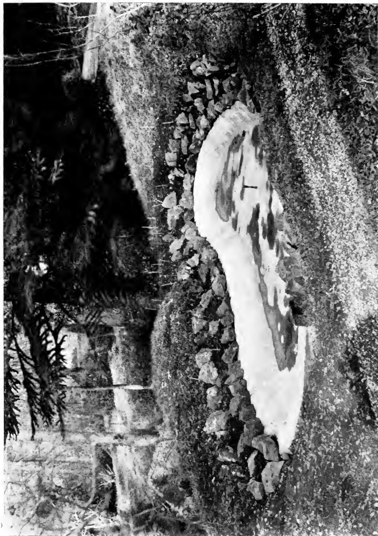
Fig. 14.—A sound 'concrete basin,' bottom and sides reinforced with old iron. (This pond is on a very bad foundation.)
