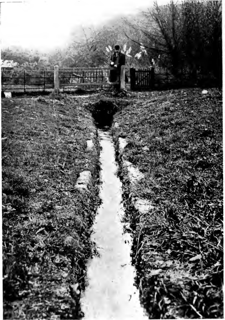
Fig. 37.—STONE DITCH EDGED WITH CONCRETE.
