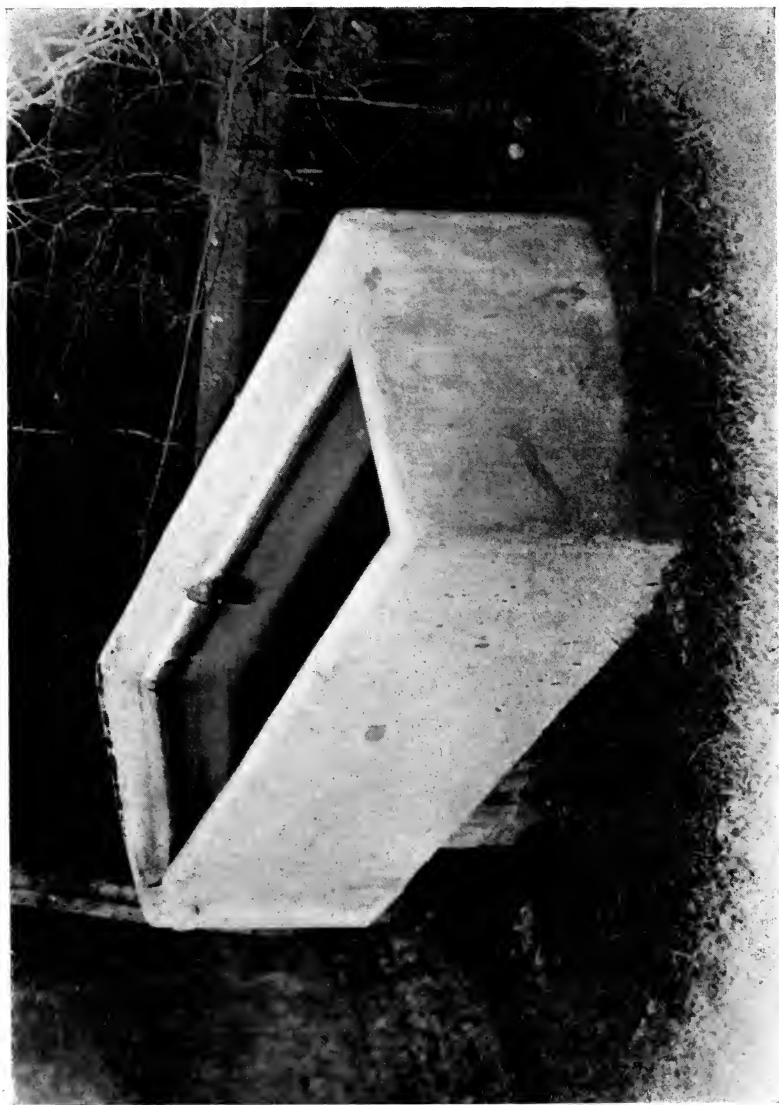
Fig. 38.—CONCRETE DRINKING TANK.
