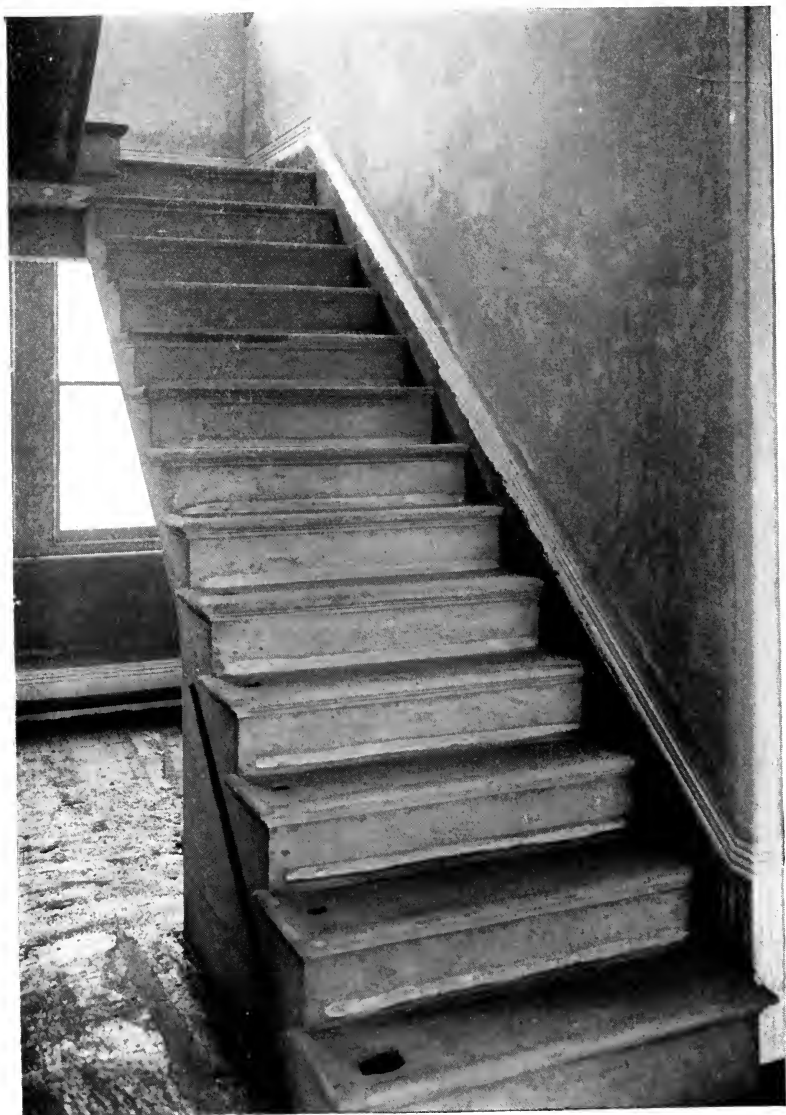
Fig. 17.—Illustration of Stairs, showing holes left for newel and balustrade. The wood insertion for fixing stair-rod eyelets can be seen.
