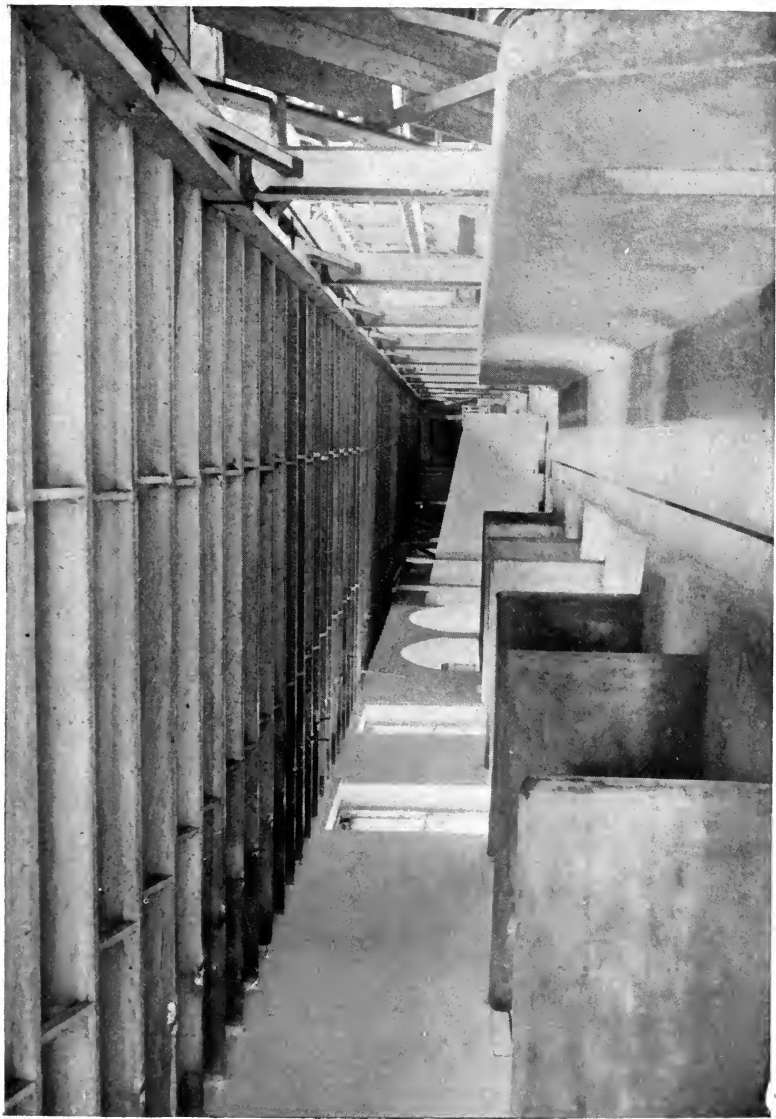
Fig. 23.—CONCRETE COW STALLS : WINNINGS FARM, COLWALL.
