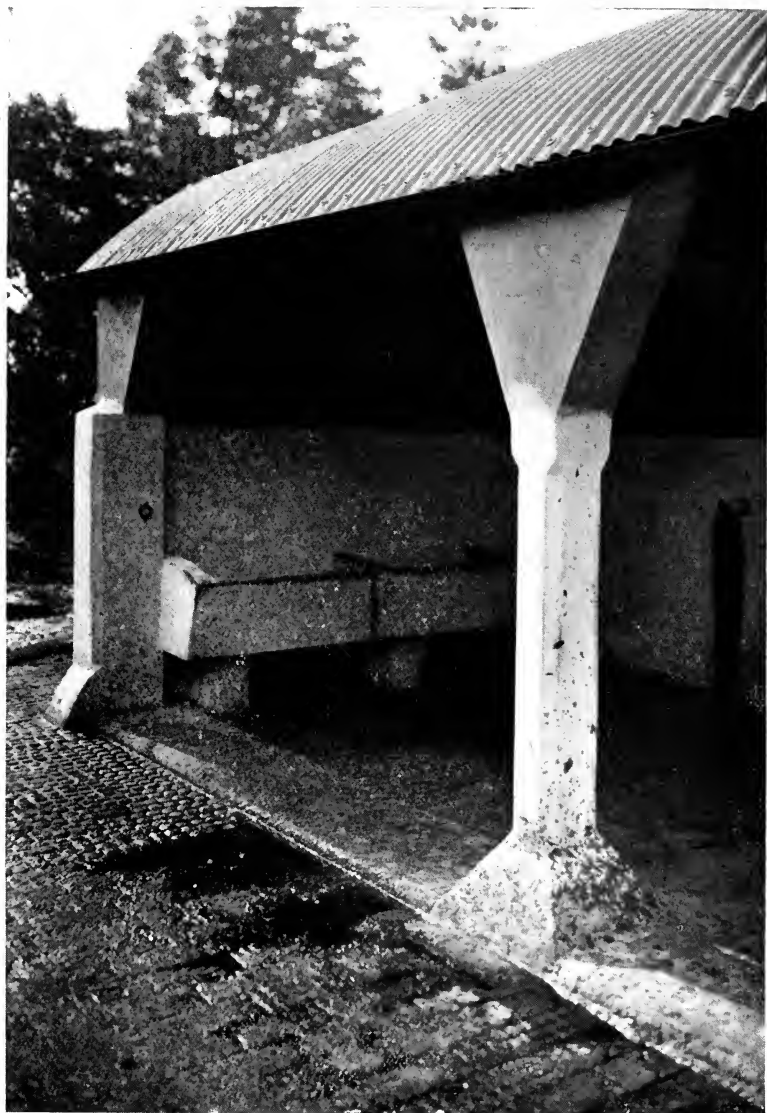
Fig. 22.—CONCRETE PILLARS.
