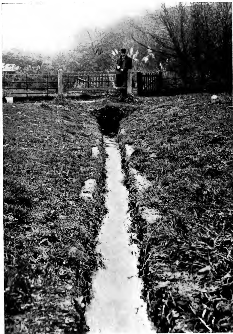
Fig. 37.—STONE DITCH EDGED WITH CONCRETE.
