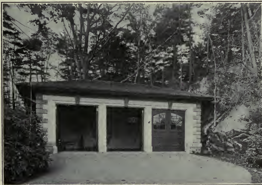
Garage at Beverly Farms, Mass. Solid Concrete.
