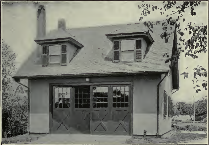
Garage at Far Rockaway, L. I. Stucco on Wood Stud and Metal Lath.
