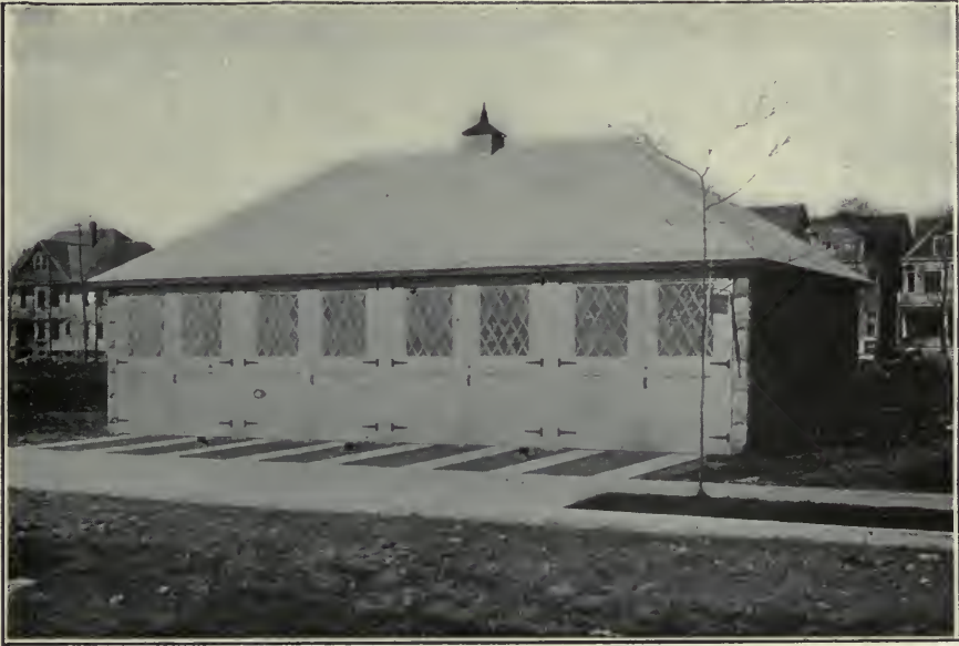
Garage at Paterson, N. J. Concrete Block.
