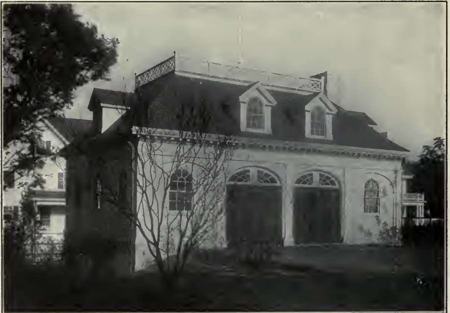
Solid Concrete Garage, Newton, Mass.
