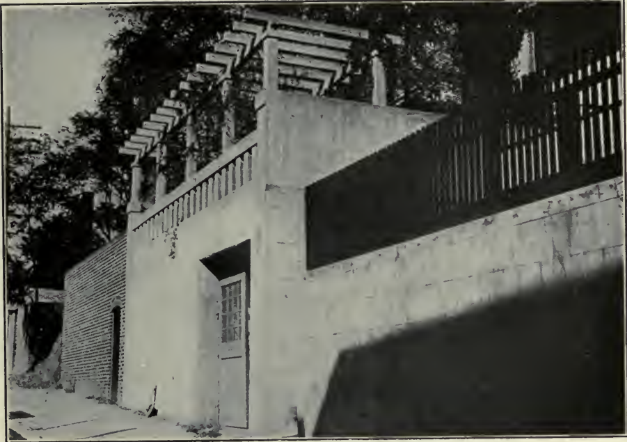
Solid Concrete Garage Built in Wall, Washington, D. C.
