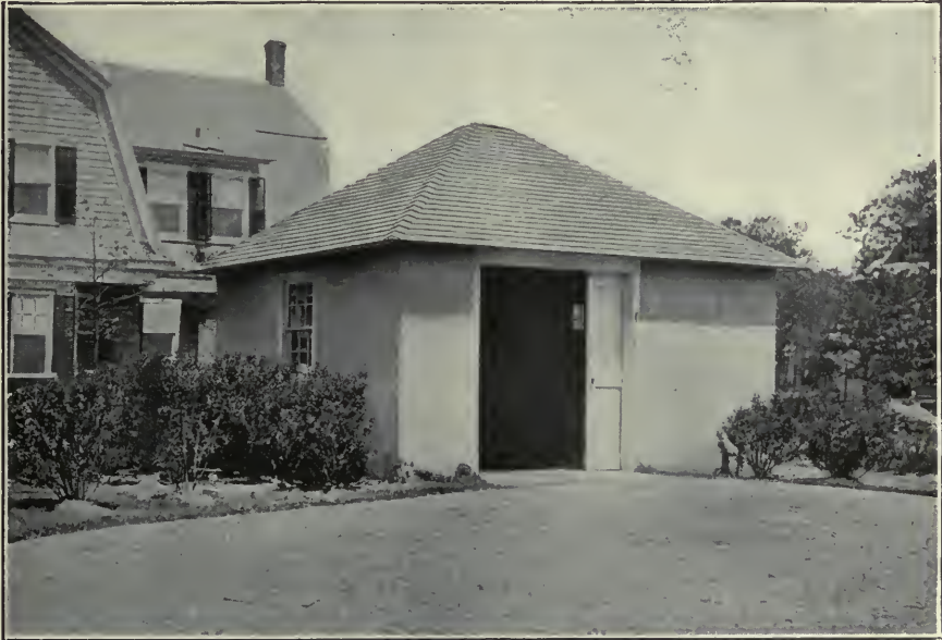
Garage at Woodmere, L. I. Stucco on Wood Frame and Metal Lath.
