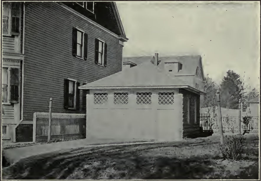
Garage at Paterson, N. J. Concrete Block.
