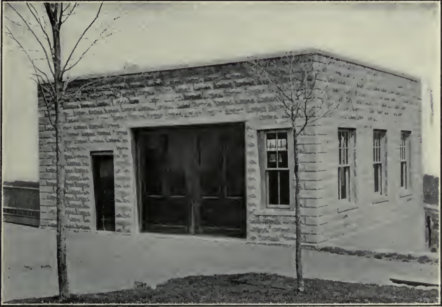
Garage at Scarsdale, N. Y. Concrete Block.
