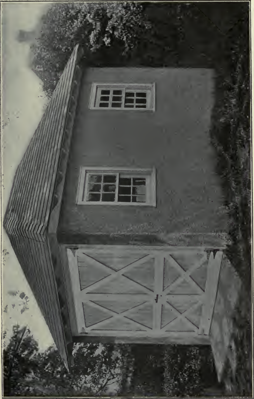
Garage at Far Rockaway, L. I., N. Y. Stucco on Wood Frame and Metal Lath.
