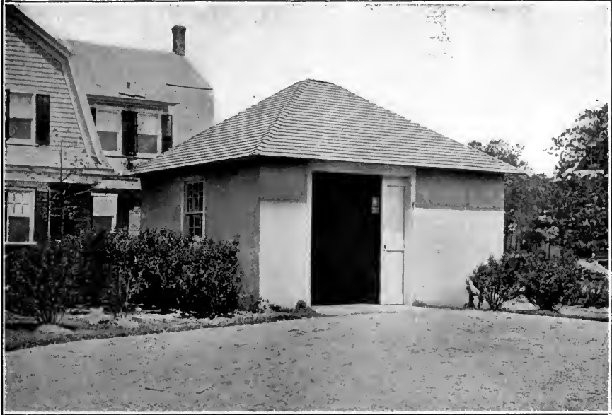
Garage at Woodmere, L. I. Stucco on Wood Frame and Metal Lath.
