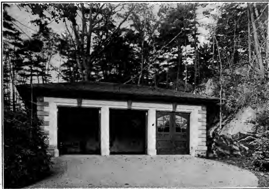
Garage at Beverly Farms, Mass. Solid Concrete.
