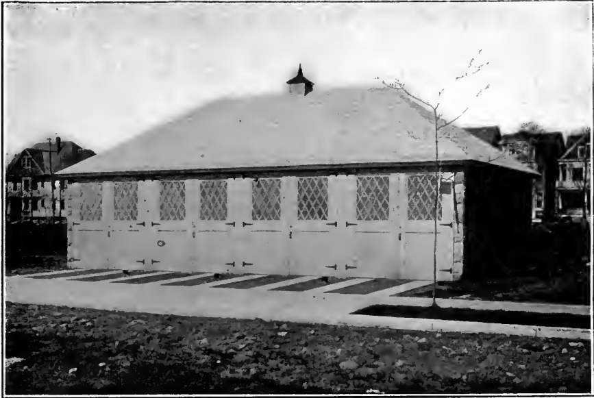
Garage at Paterson, N. J. Concrete Block.
