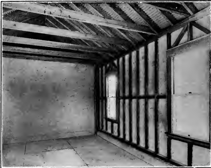
Interior of Garage at Allentown, Showing Wood Frame with Stucco on Both Sides of Metal Lath.
