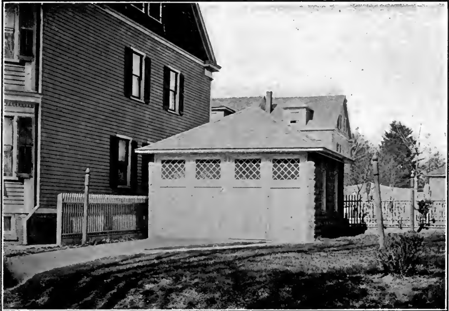
Garage at Paterson, N. J. Concrete Block.
