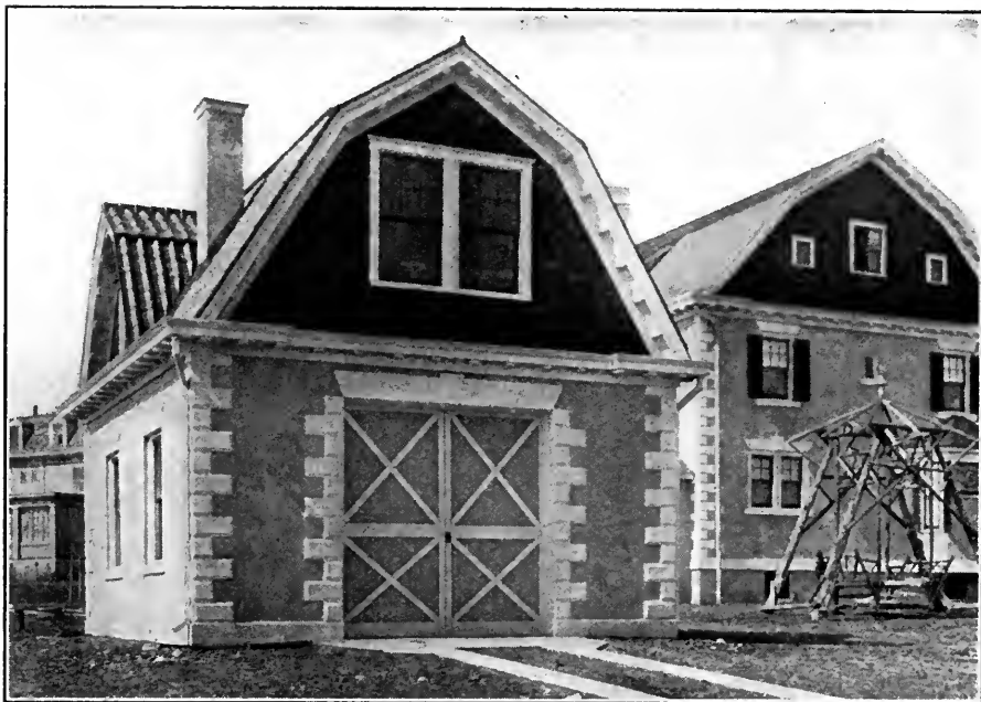
Concrete Block and Stucco Garage, Haworth, N. J.
