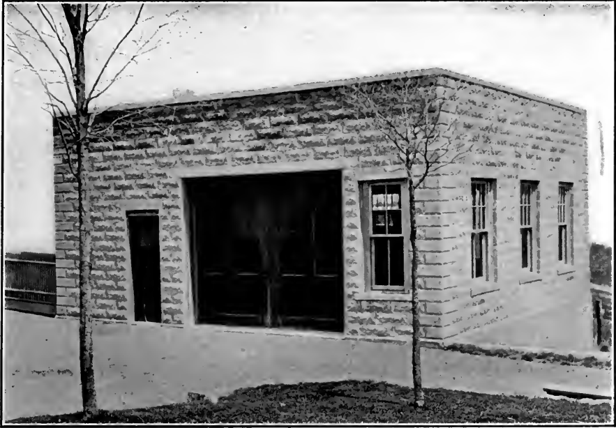
Garage at Scarsdale, N. Y. Concrete Block.
