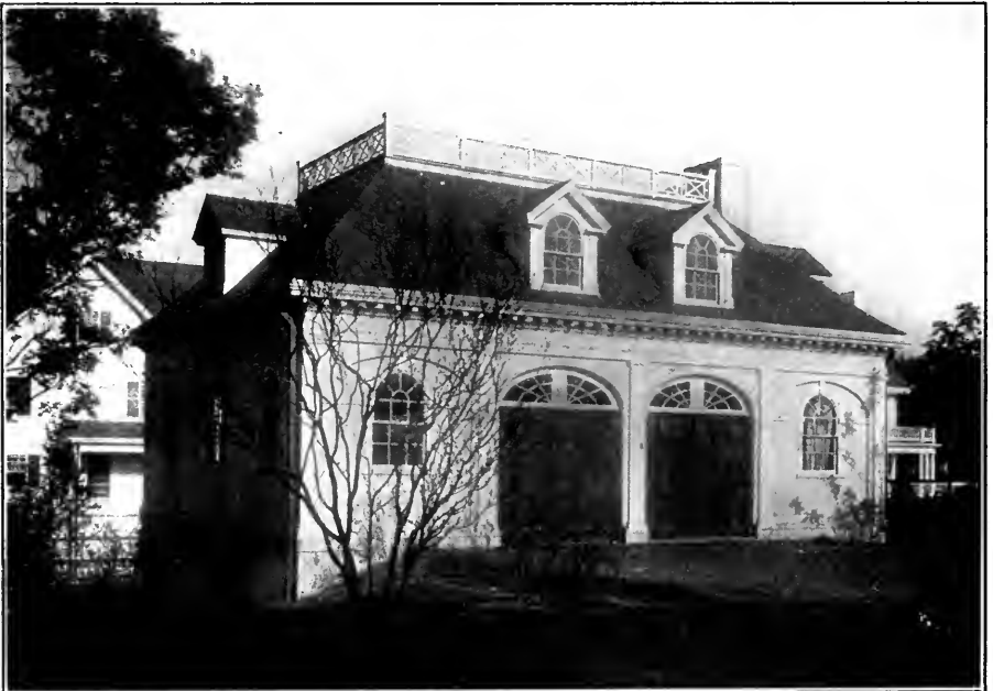
Solid Concrete Garage, Newton, Mass.
