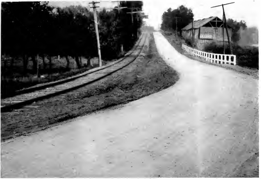
FIG. 6.—CONCRETE ROAD, LAKE SHORE ROAD, KENOSHA, KENOSHA CO., WIS.
