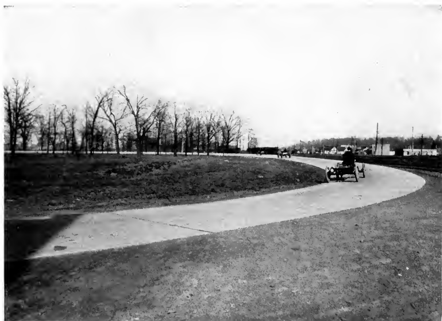
FIG. 5.—CONCRETE AUTOMOBILE TRACK, MOLINE, ILL.
