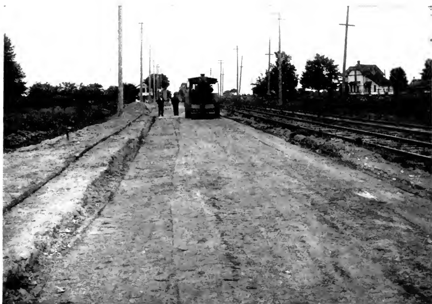
FIG. 44.—PREPARATION OF SUB-BASE.
