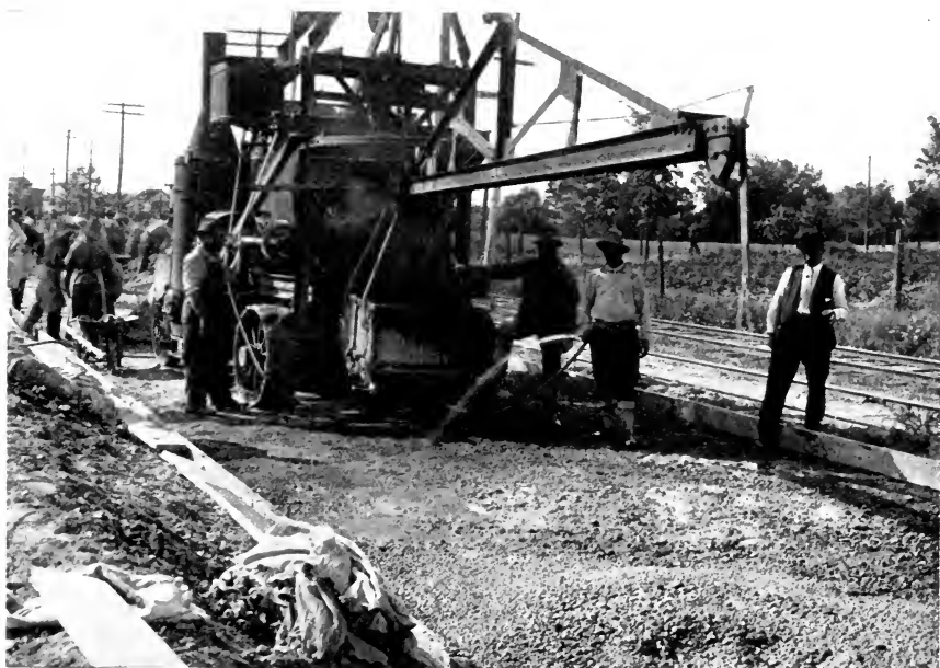
FIG. 45.—WETTING SUB-BASE IMMEDIATELY BEFORE PLACING CONCRETE.
