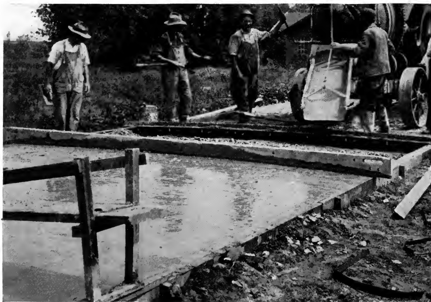
FIG. 48.—CONCRETE ROAD DURING CONSTRUCTION.
