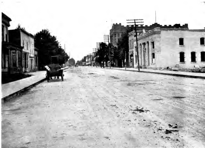
FIG. 23.—SAND BEACH AVE., BAD AXE, MICH. TWO-COURSE CONCRETE.
