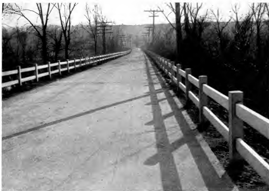
FIG. 2.—LA SALLE-OGLESBY ROAD, ILL. Concrete road subjected to floods which ruined all previous roads.
