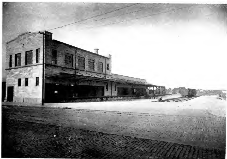
FIG. 29.—CONCRETE PAVEMENT IN FRONT OF C. R. I. & P. RY. STATION, MASON CITY, IA.
