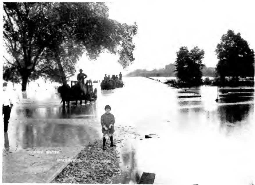
FIG. 20.—HILLSBORO CONCRETE ROADWAY, GREENVILLE, ILL. Flooded but serviceable.
