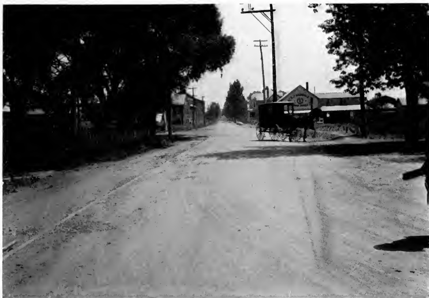
FIG. 3.—CONCRETE ROAD, NAZARETH, NORTHAMPTON CO., PA.
