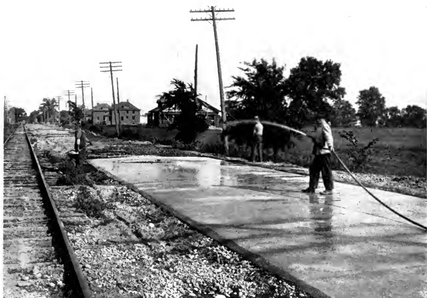
FIG. 49.—PROTECTION OF ROAD. WETTING AND COVERING WITH DIRT.
