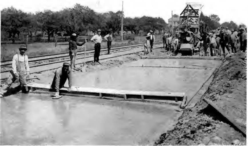
FIG. 9.—METHOD OF CONSTRUCTION ON GRAND RIVER ROAD, WAYNE CO., MICH. BUILT 1911.
