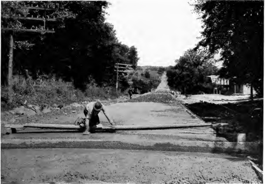
FIG. 54.—JANESVILLE ROAD, MILWAUKEE CO., WIS. Method of constructing one-course concrete pavement.
