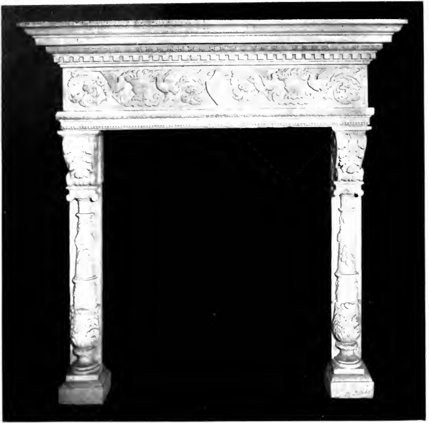
Fig. 31. Elaborate but interesting treatment of concrete.
