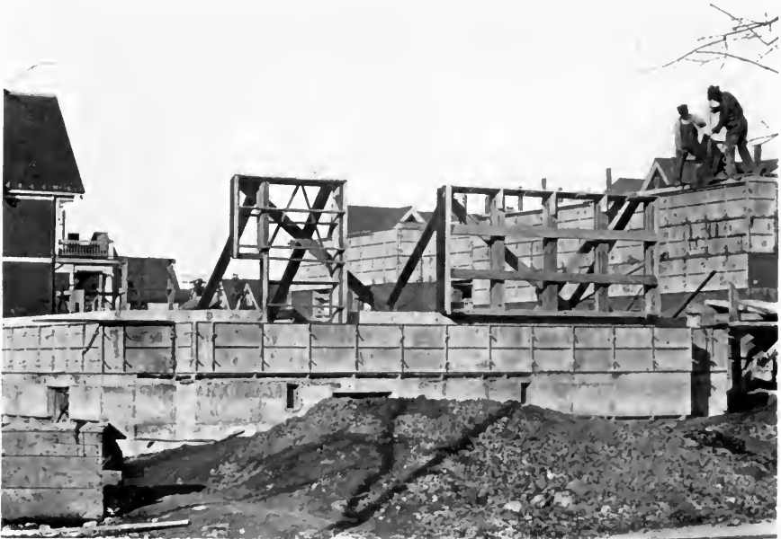
Patented steel forms in use.
