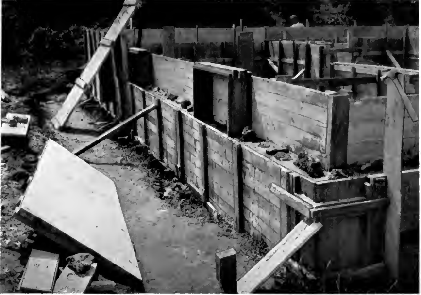
Typical sectional form for concrete wall construction.
