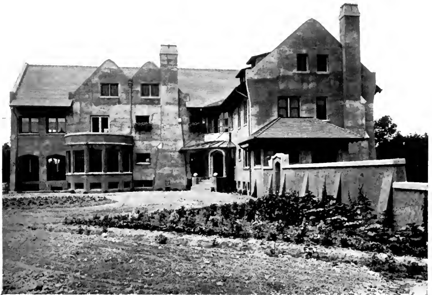
Fig. 3.—A carefully studied design, showing frank treatment of concrete walls and surface finish.
