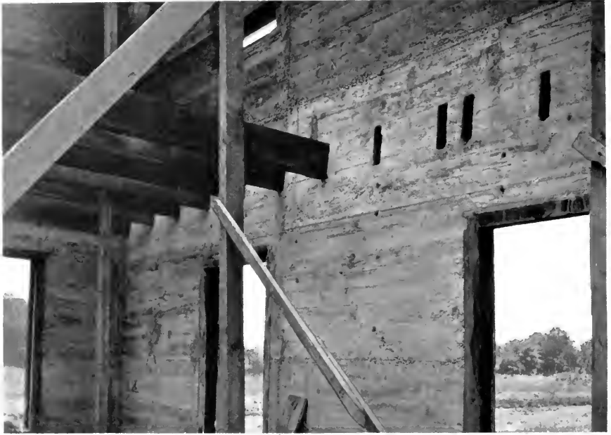
Wall recesses for timber joist.
