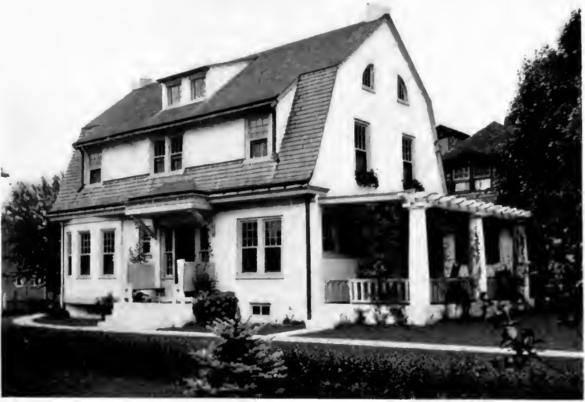
Fig. 14.—A handsome house showing successful use of concrete, but without emphasizing its character.
