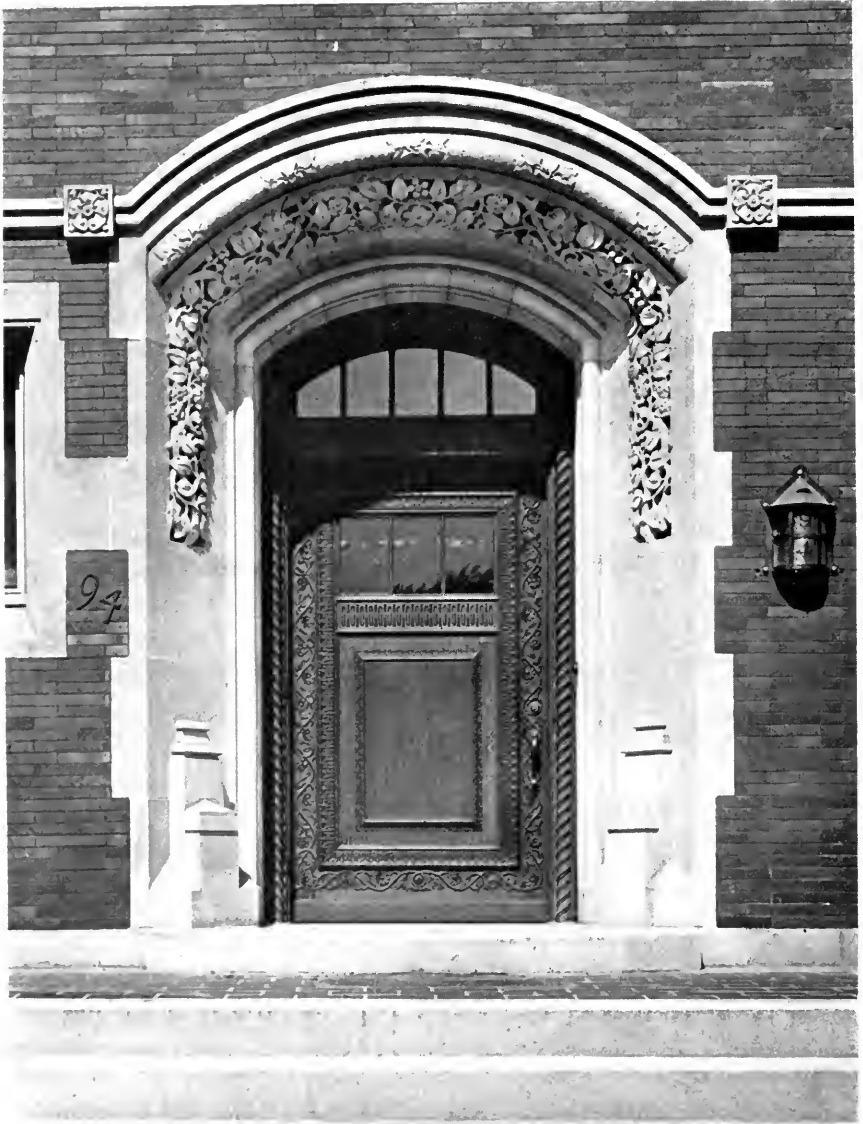
A doorway showing the adaptability of concrete to either plain or ornamental work. Note the great contrast between the elaborate undercut floral decoration and the simple units comprising the structural features.
