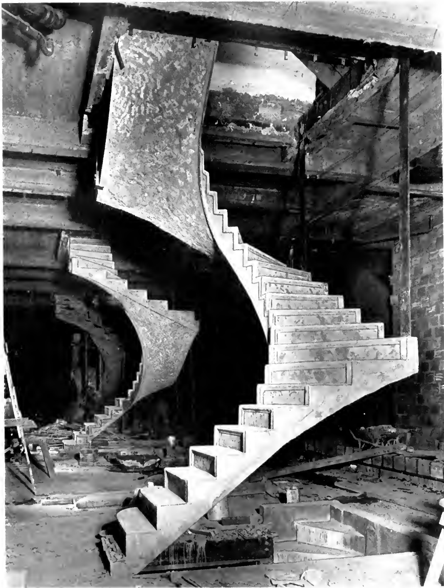
Example of the adaptability and economy of concrete in stairway construction.
