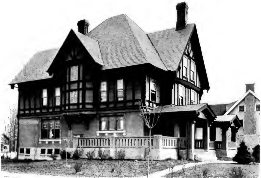
Fig. 6.—Concrete as adapted to the requirements of English half-timber design. Note monolithic corbel or shelf supporting window.
