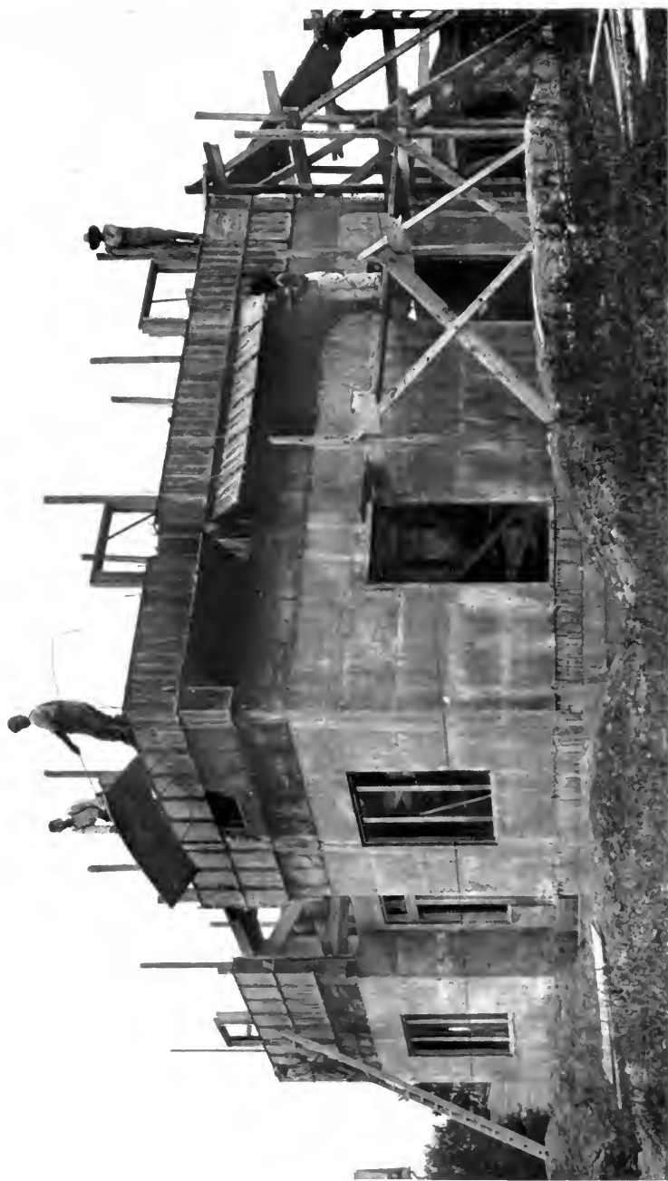
Method of raising and adjusting steel forms by the two-tier process, by Read & Morrill, Brooklyn, N. Y. Forms designed and patented
