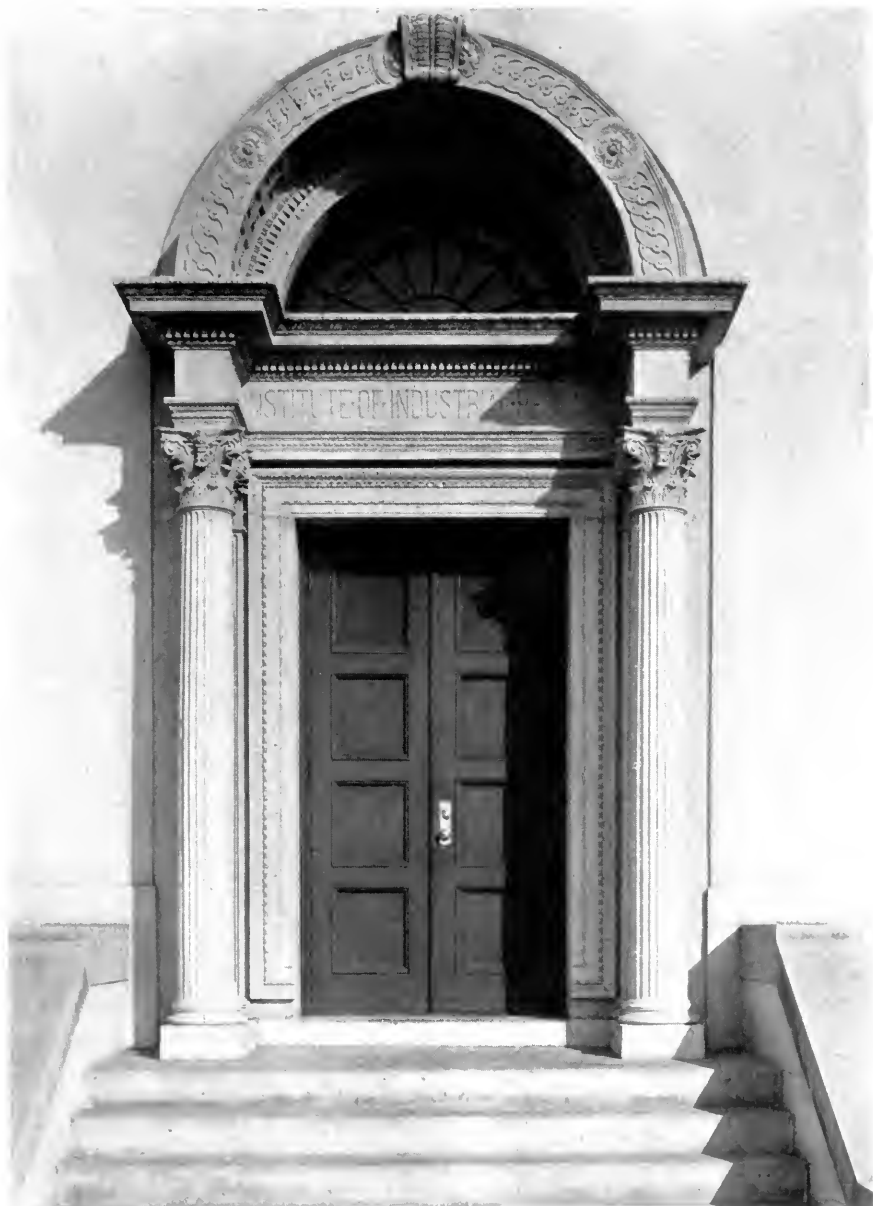
Fig. 16.—Concrete should be translated into simple and original forms as opposed to the elaborate detail shown above.
