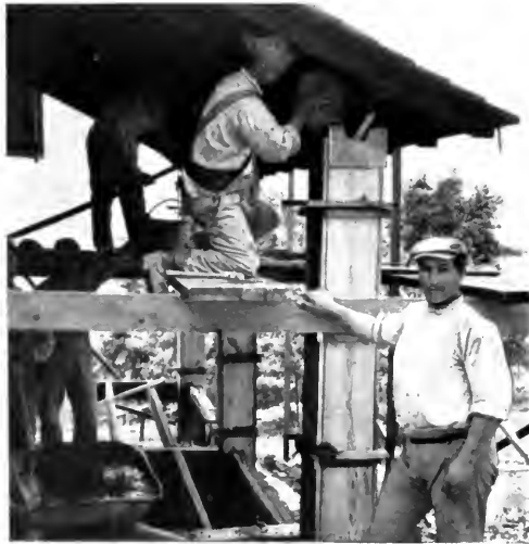
Pouring concrete into a column form.
