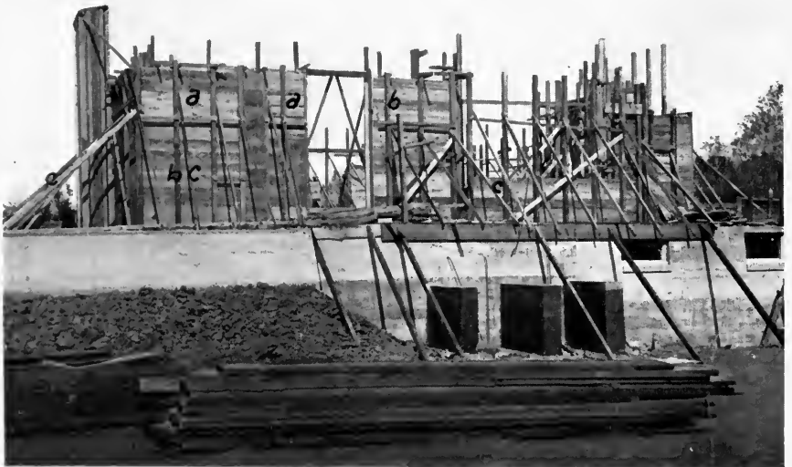
Fig. 63.—Typical example of form work in one-story wall construction.
