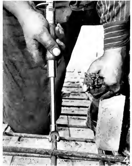
Fig. 77.—“Curry Tyer.” A convenient method for wiring reinforcement together.
