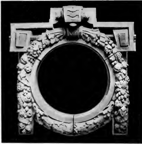
Fig. 23.—A fine example of separately cast concrete detail.
