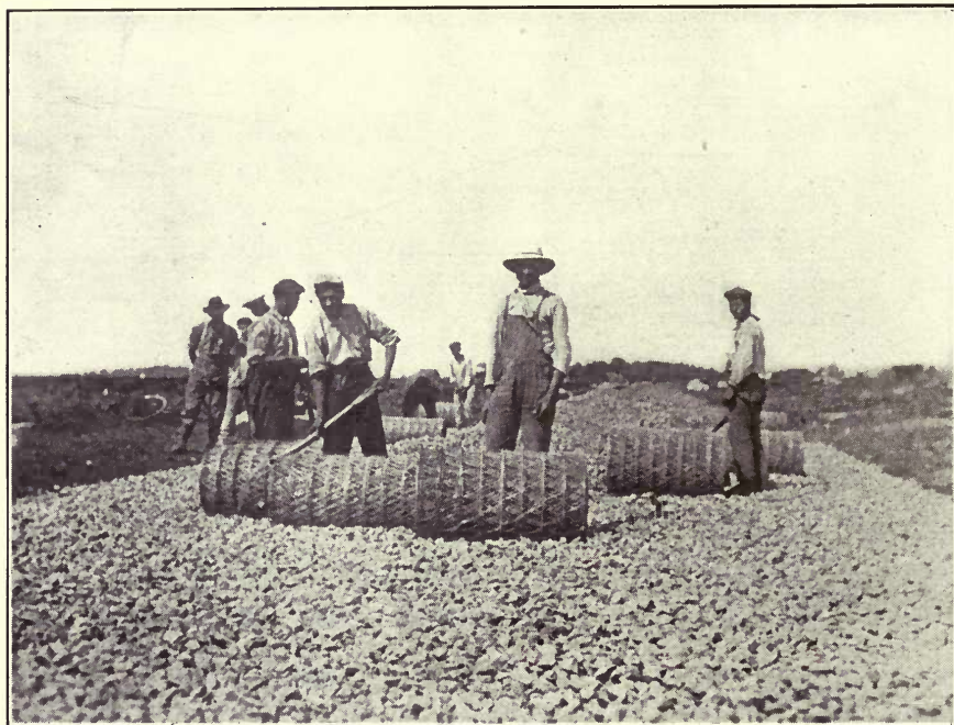
FIG. 19.—CONSTRUCTION OF LONG ISLAND MOTOR PARKWAY.
