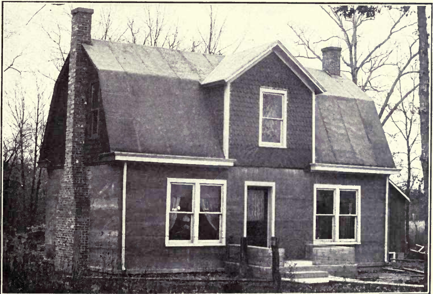
CONCRETE HOUSE NEAR MORTON, ILL.
