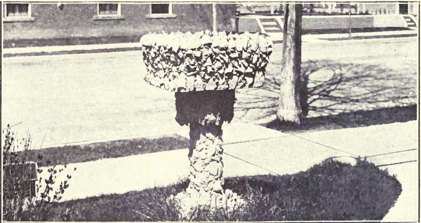
CONCRETE FLOWER BOX AT PATERSON, N. J.
