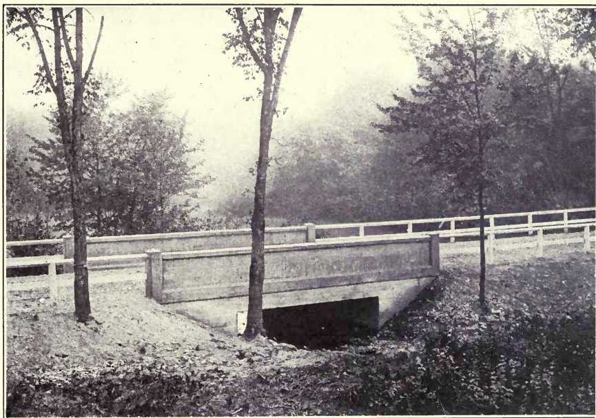
FIG. 42.—CONCRETE BEAM BRIDGE.
