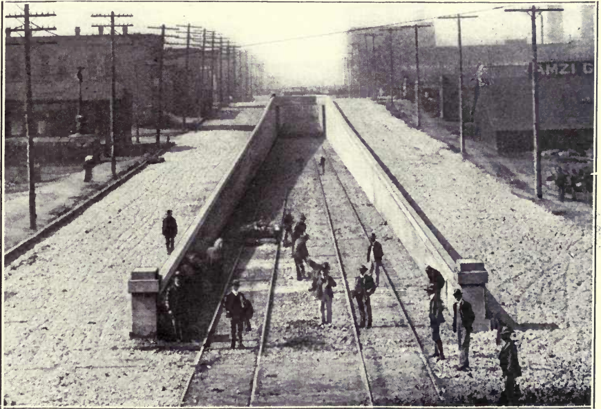
RETAINING WALLS, BIRMINGHAM, ALA.
