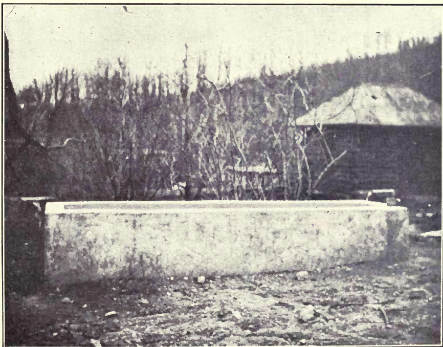
WATERING TROUGH AT BERRY HILL, L. I.
