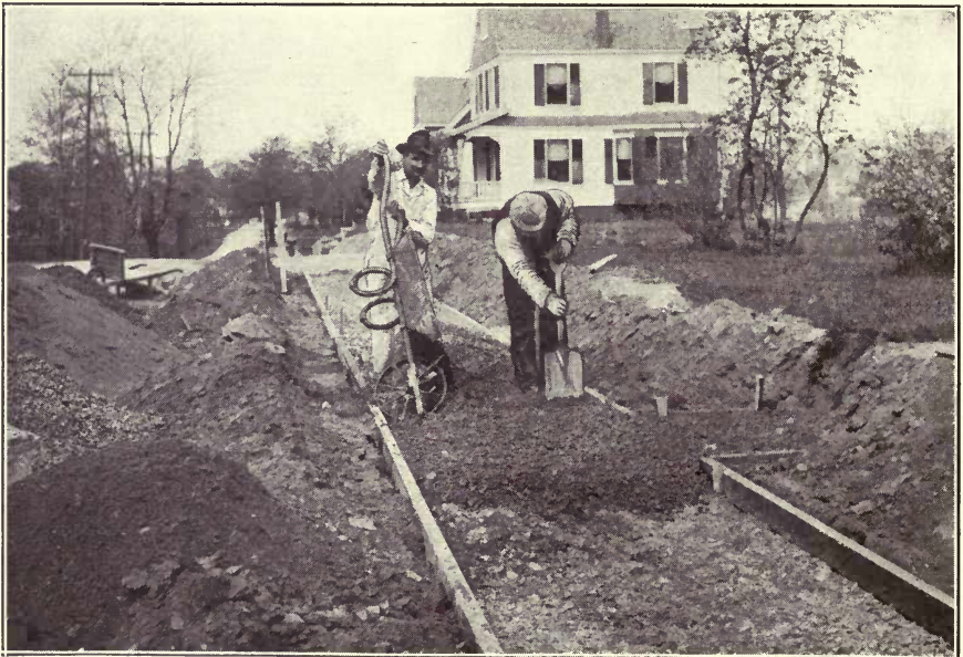
FIG. 7.—PLACING THE CONCRETE BASE.
