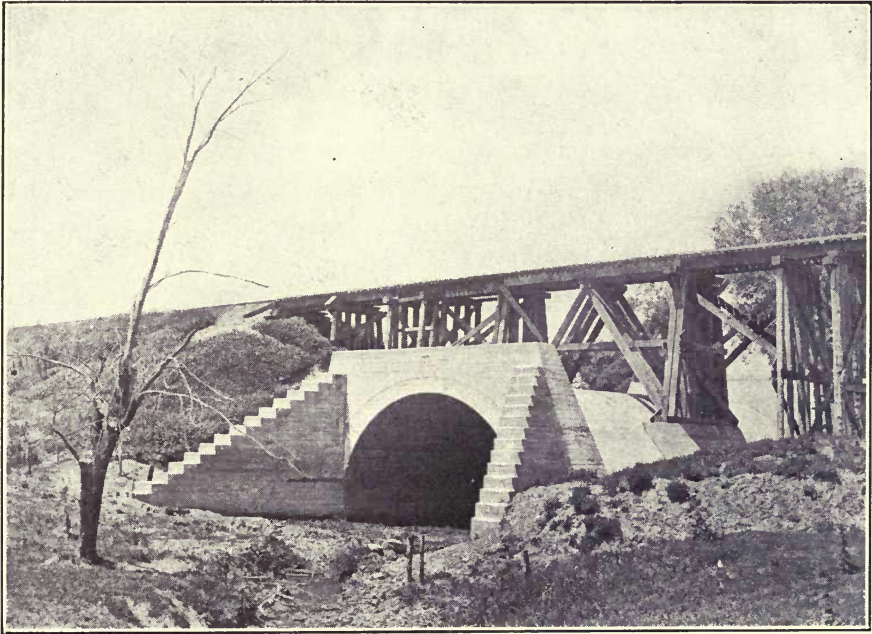
FIG. 45.—THIRTY FOOT CULVERT, C., M. & ST. P. RY.
