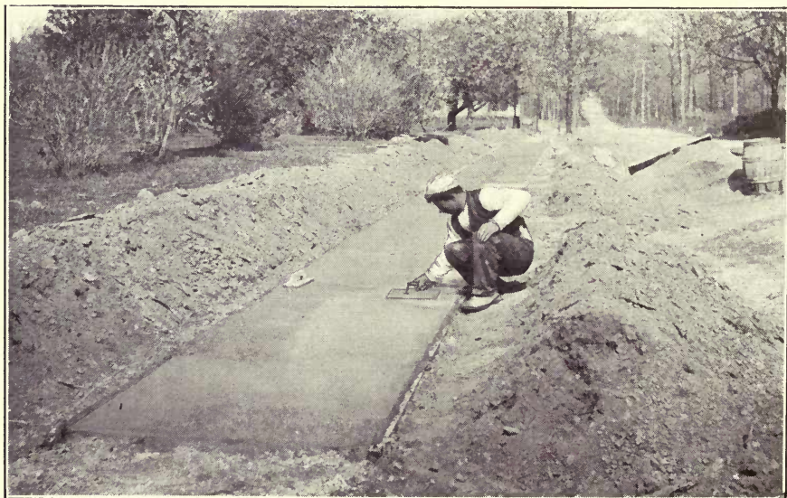
FIG. 9.—TROWELING WEARING SURFACE.
