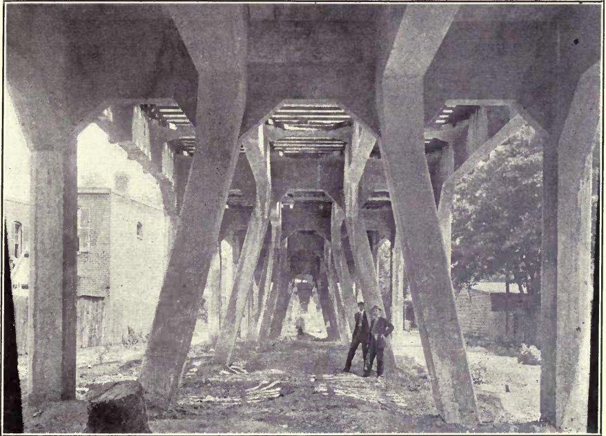
FIG. 19.—VIEW FROM GROUND, RICHMOND VIADUCT.
