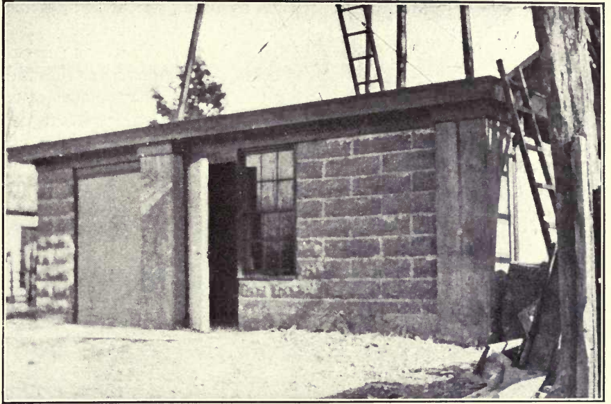
WELL HOUSE WITH HEAVY CONCRETE COLUMNS FOR SUPPORTING STEEL FRAME OF HIGH WATER TANK AT COLUMBIA, MO.
