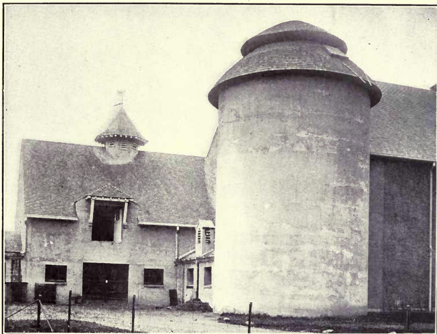
ONE OF THE SILOS AT GEDNEY FARMS, WHITE PLAINS, N. Y.
