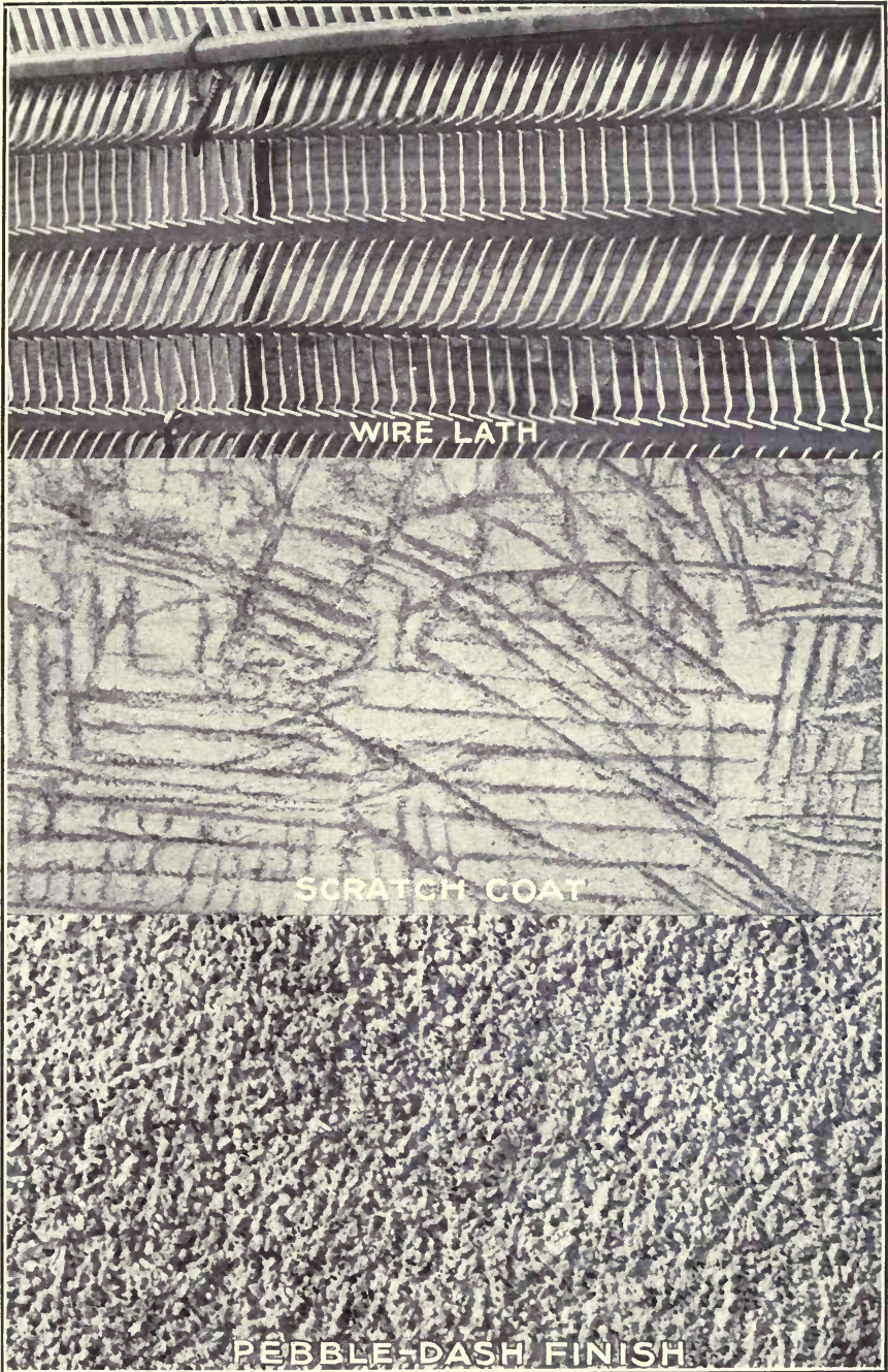
METHOD OF APPLYING PEBBLE DASH FINISH
