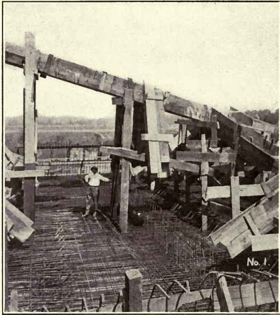
CHUTE FOR DEPOSITING CONCRETE, PAINSVILLE BRIDGE.
