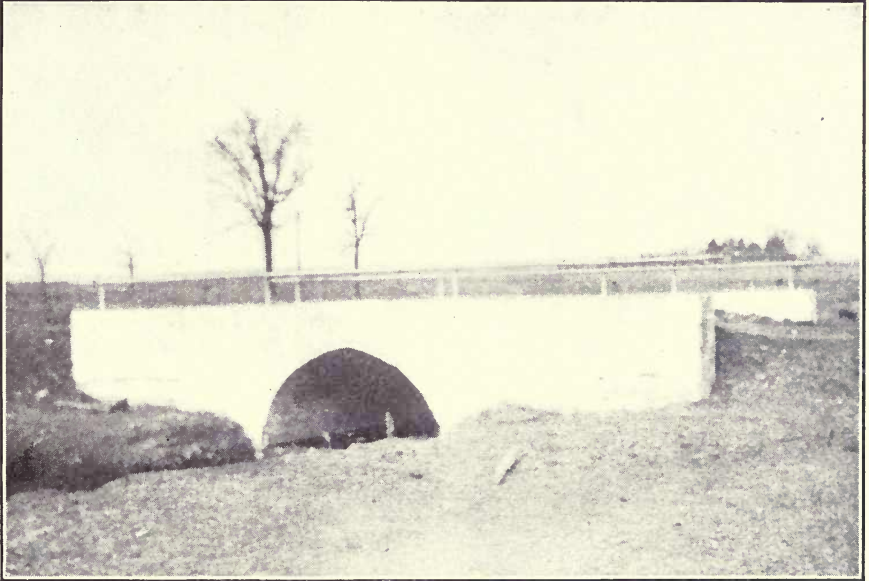
CULVERT AT HARRISTOWN, ILL.
