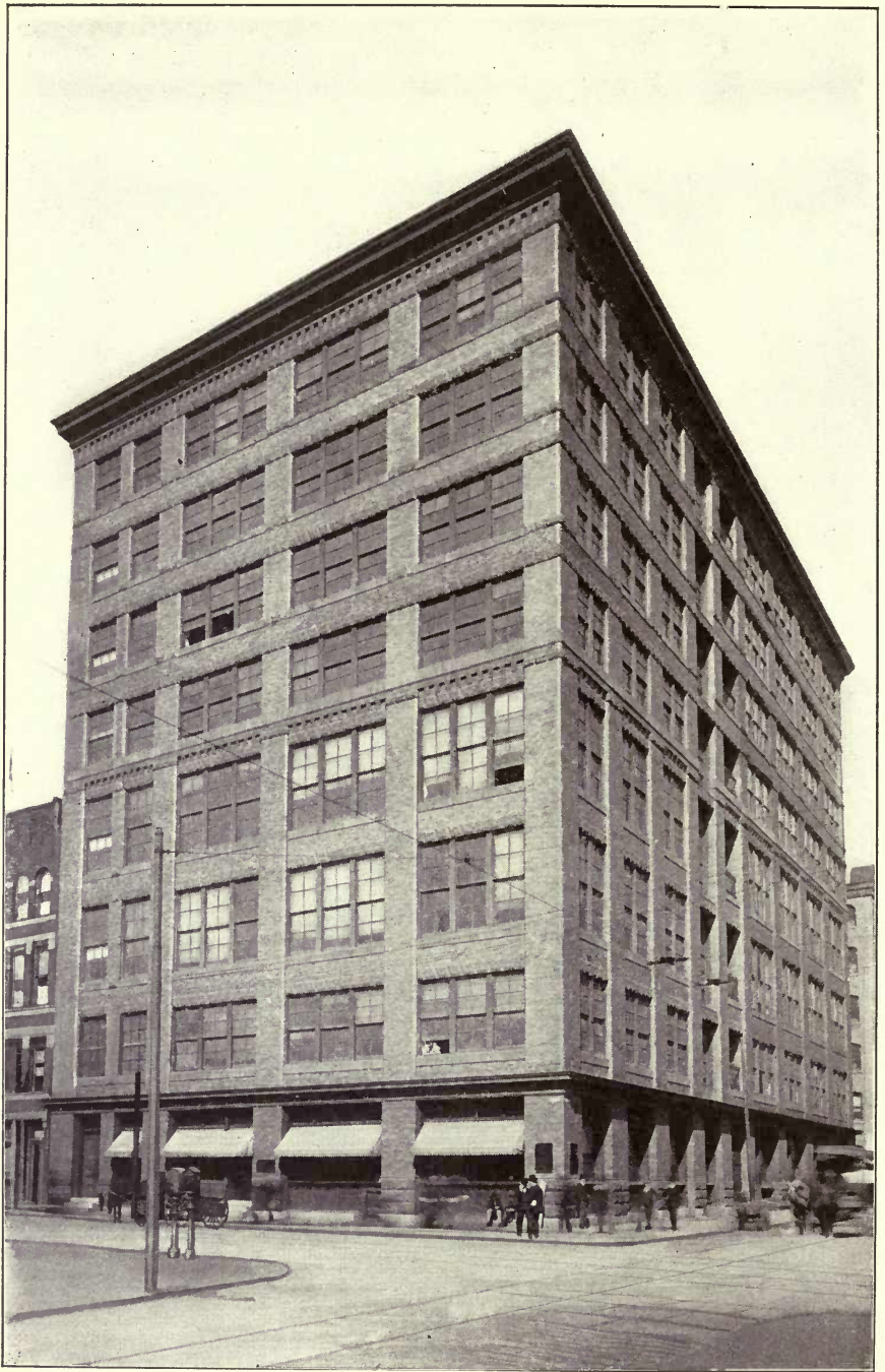
Fig. 14.—The Ketterlinus Building. (See p. 61.)
