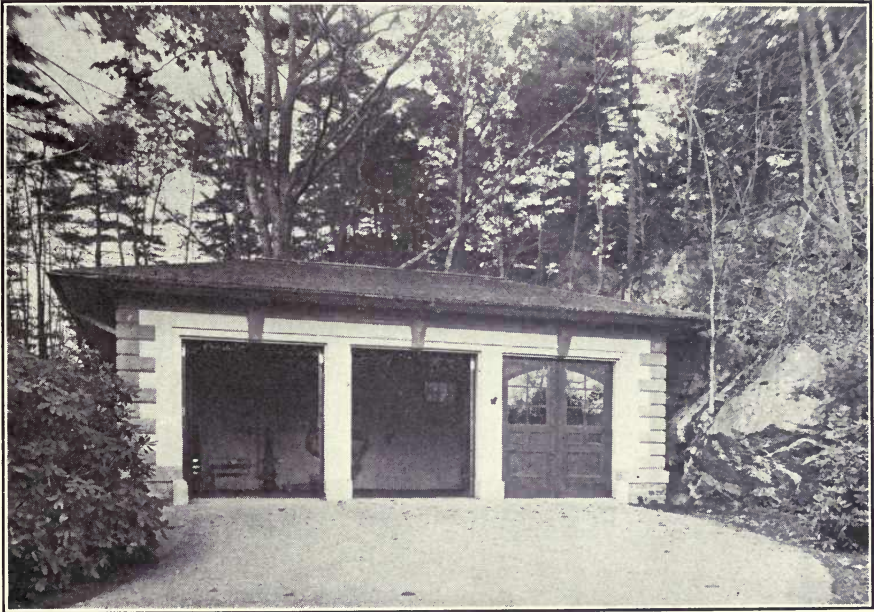
Garage at Beverly Farms, Mass. Solid Concrete.
