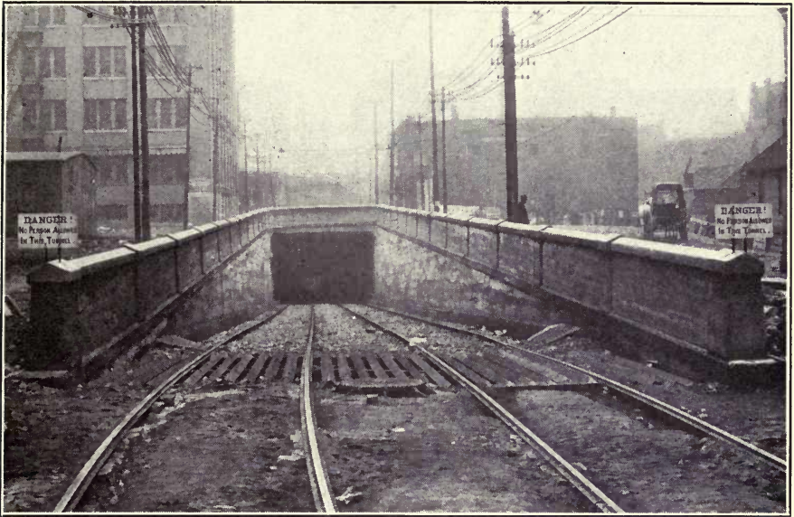
PORTAL 8TH STREET TUNNEL, KANSAS CITY, MO.
