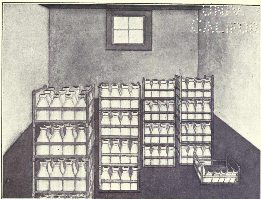
INTERIOR OF CONCRETE ICE BOX AT BROOKSIDE FARMS, NEWBURGH, N. Y.
