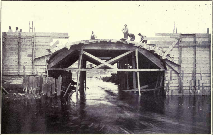
FIG. 57.—CENTERING FOR ARCH IN PLACE.
