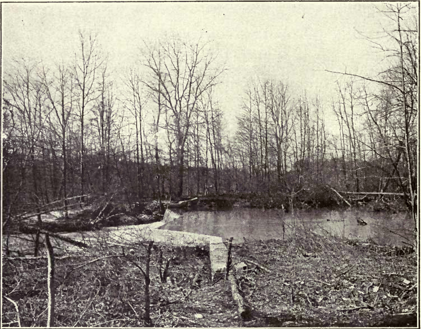
DAM AT ARLINGTON, VA.
