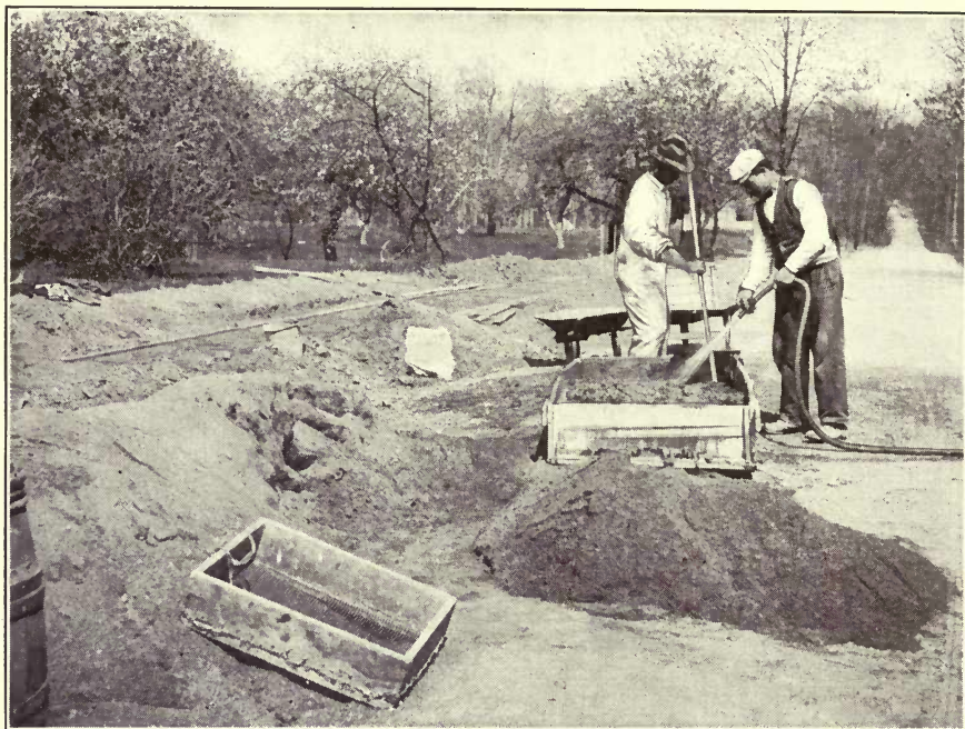
FIG. 8.—MIXING MORTAR FOR WEARING SURFACE.
