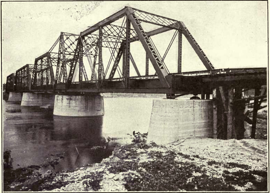
PIERS, GRAND RIVER BRIDGE, PERE MARQUETTE R.R.
