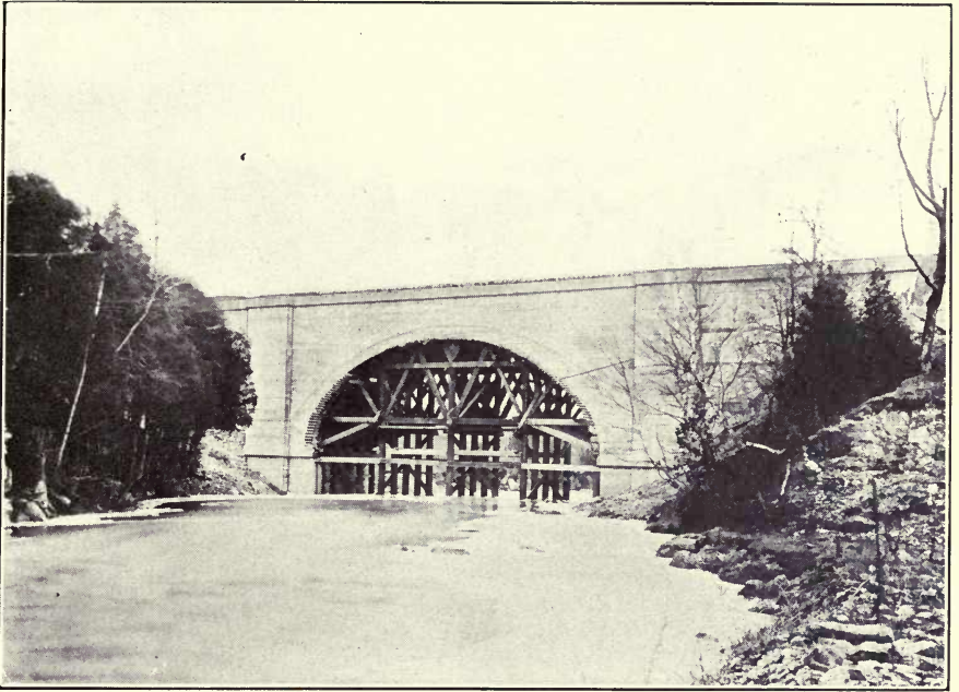
BRIDGE U 44, C., M. & ST. P. RY.
