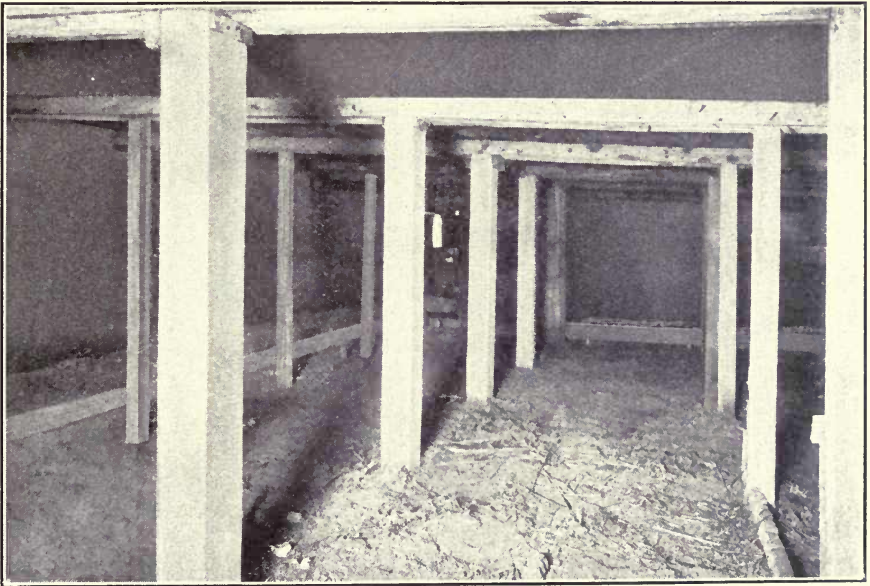
INTERIOR OF MUSHROOM CELLAR AT WESTWOOD, N. J.
