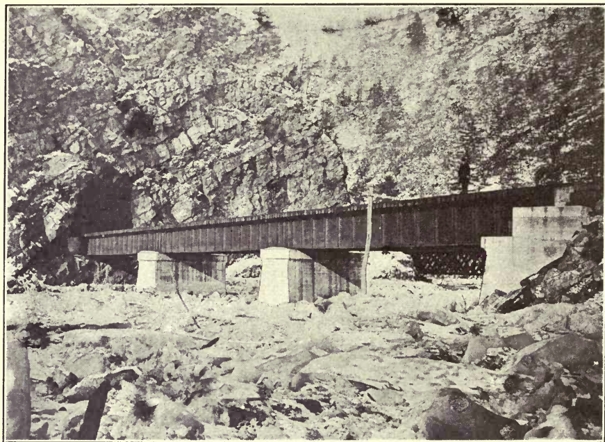
FIG. 49.—CONCRETE PIERS DURING ICE JAM, C. R. R. OF N. J.
