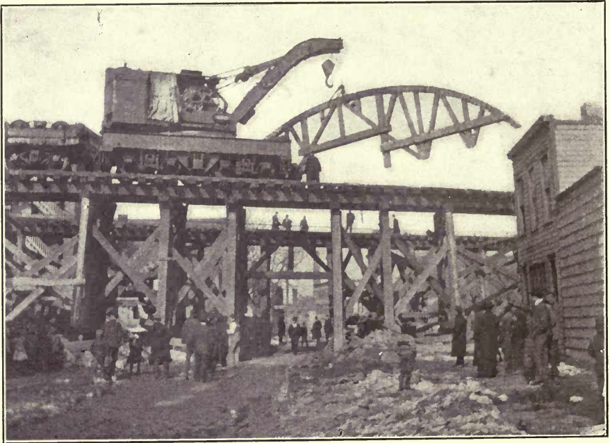
FIG. 7.—SETTING ARCH CENTERS.
