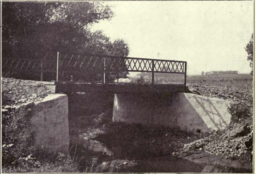
BRIDGE NEAR WASCO, ILL.
