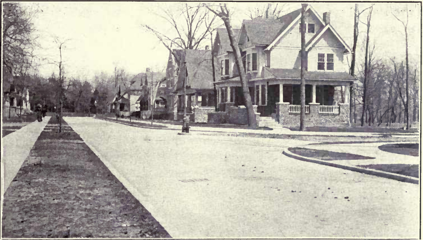
FIG. 14.—CONCRETE ROAD AT FLUSHING, L. I., N. Y
