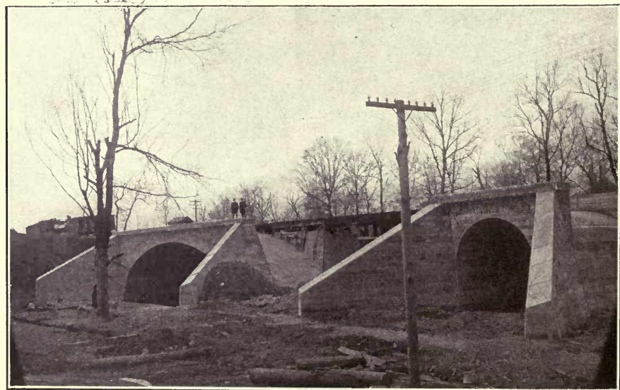
FIG. 47.—DOUBLE ARCH CULVERTS, ILL. CENTRAL R. R.
