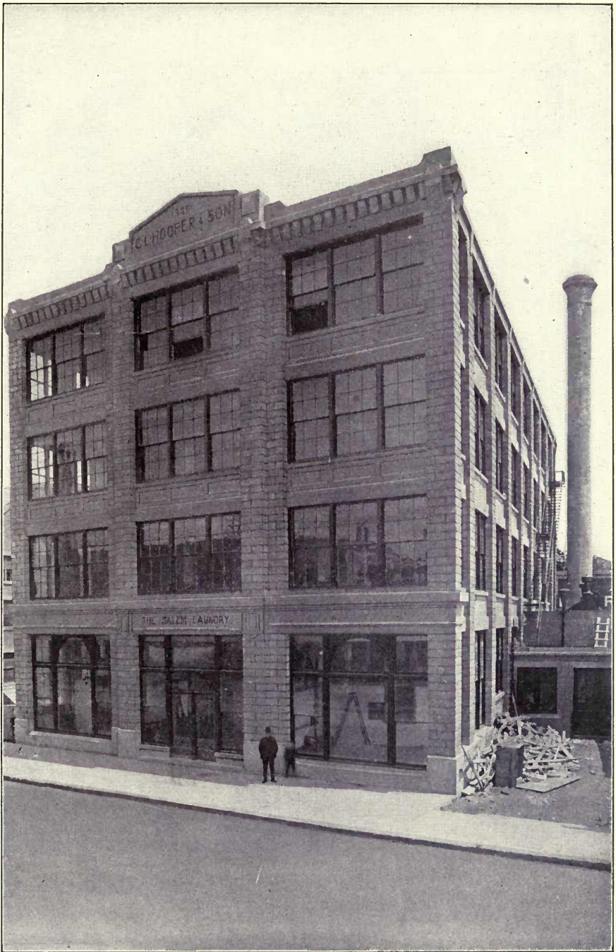
Fig. 125.—Concrete Block Walls, Salem Laundry. (See p. 195.)
