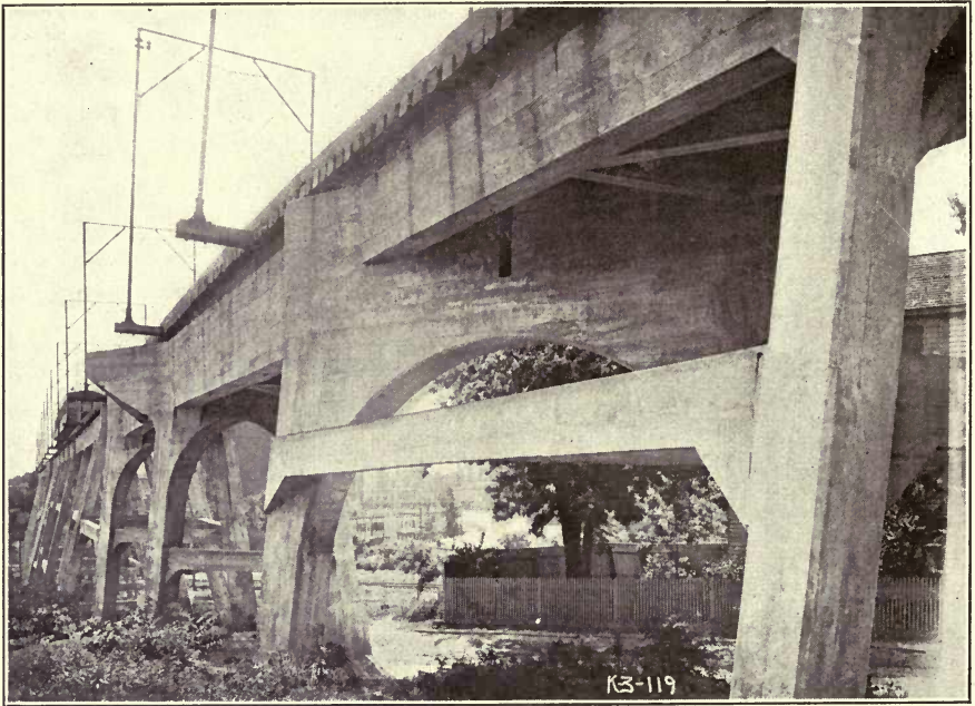
FIG. 18.—VIEW AT CURVE, RICHMOND VIADUCT.
