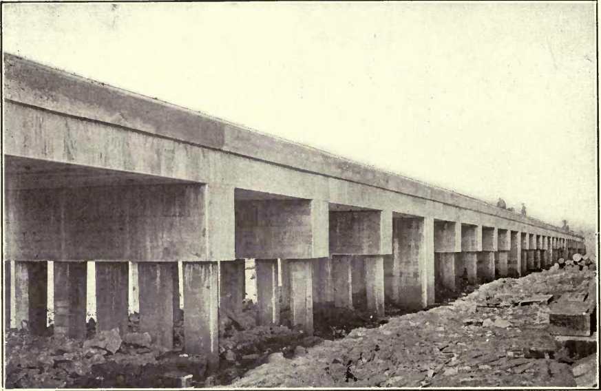
PILE TRESTLE OVER SALT RIVER, C. B. & Q. R. R.
