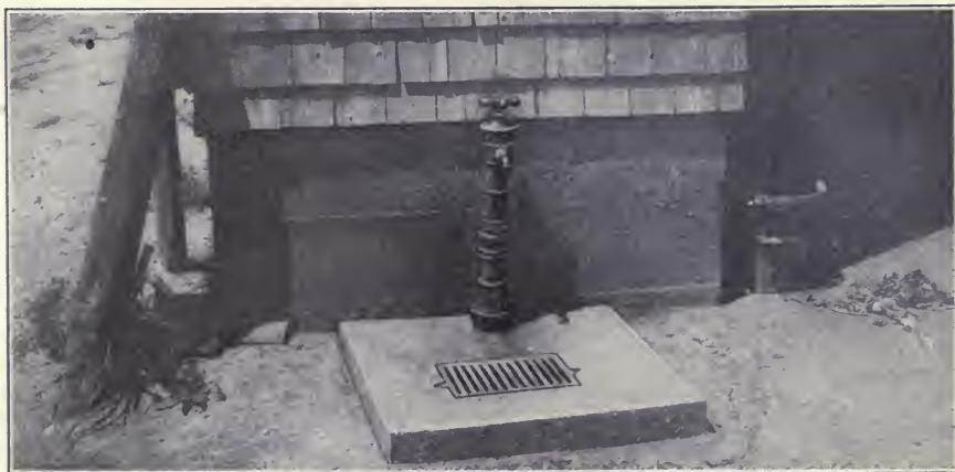
Concrete Hydrant Sink
