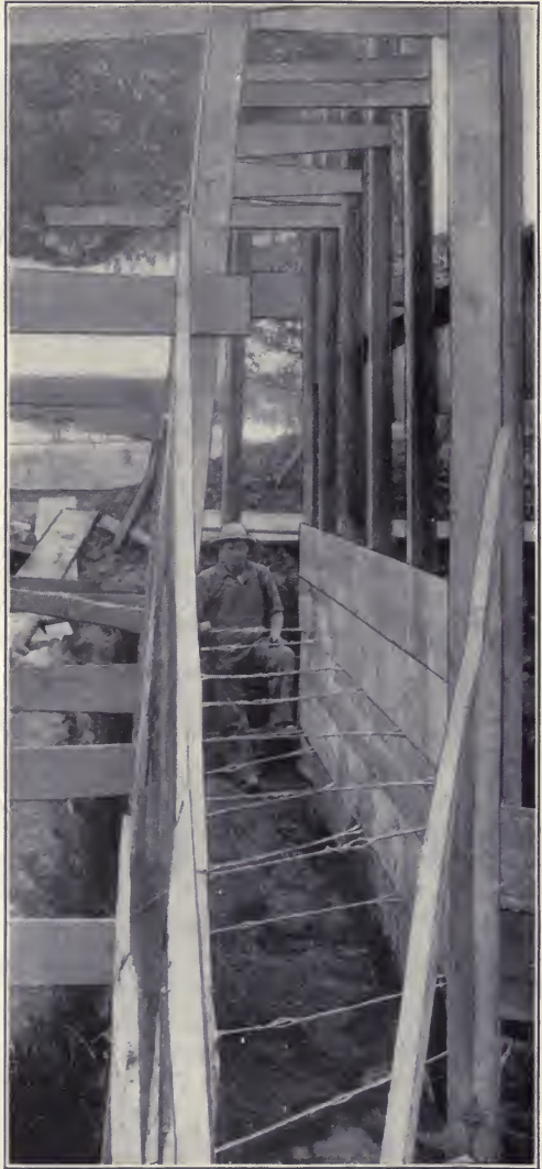
Wiring Forms Prevents Bulging.
