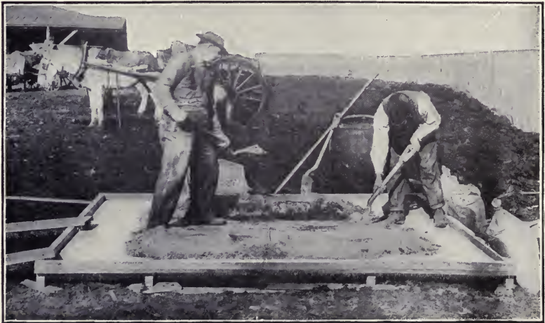
Fig. 5.—First Turning, Sand and Cement.
