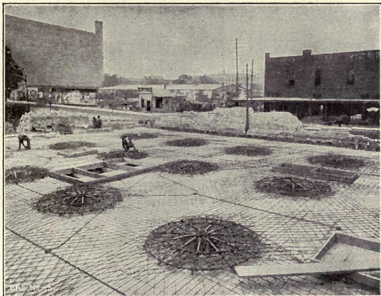
Fig. 315.—View of Floor, Mushroom System of Construction.
