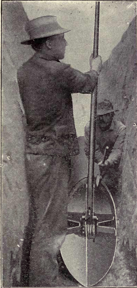
Fig. 510.—The Ransome Concrete Pipe Mold.
