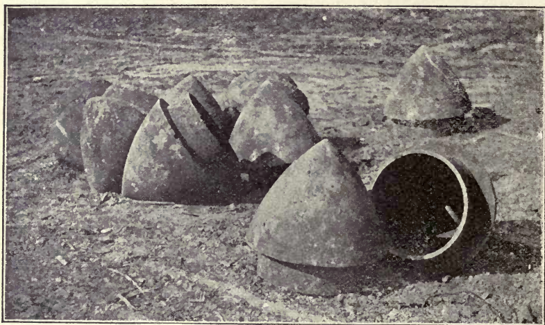
Fig. 243.—Cast Iron Points for Simplex Piles.
