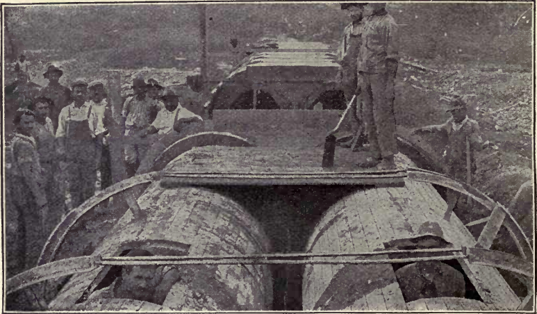
Fig. 482.—Forms for Double Conduit, Cedar Grove Reservoir.
