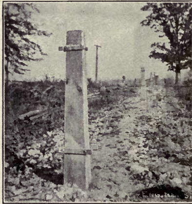
Fig. 561.—Mould for Line Post.
