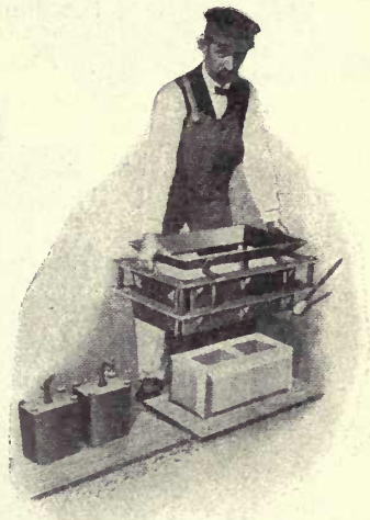
Fig. 712.—Moving the Mould Instead of the Block.
