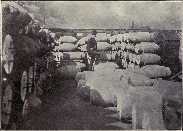
Fig. 242.—Concrete Points for Simplex Piles.
