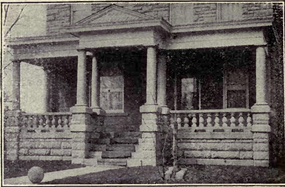
Fig. 694.—Example of Porch Work in Concrete Blocks.
