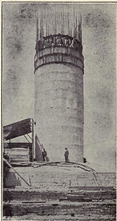
Fig. 543.—View Showing Forms for Weber Chimney.
