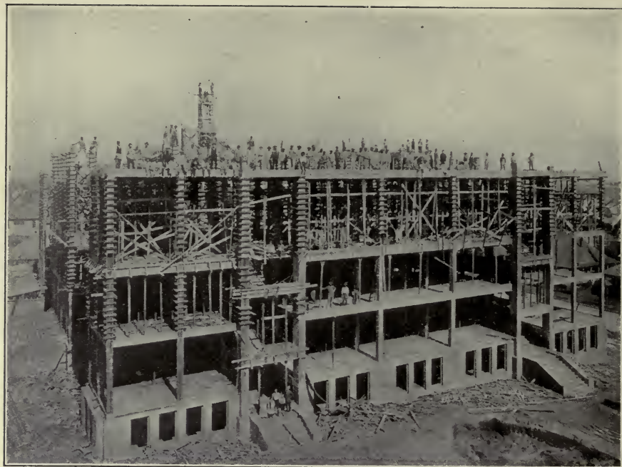
FIG. 9.—HIGH SCHOOL, FORT WORTH, TEXAS. CONCRETE FLOORS AND SKELETON.
