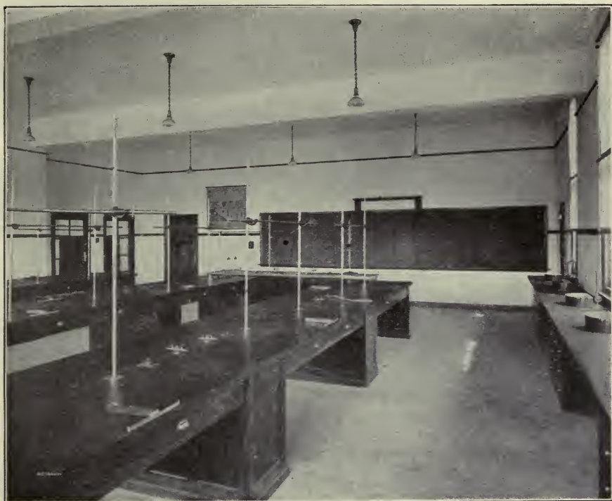
FIG. 4.—PHYSICAL LABORATORY, NORFOLK HIGH SCHOOL. NOTE SANITARY CONCRETE FLOOR AND ABSENCE OF WOODWORK WITH THE EXCEPTION OF DESKS.
