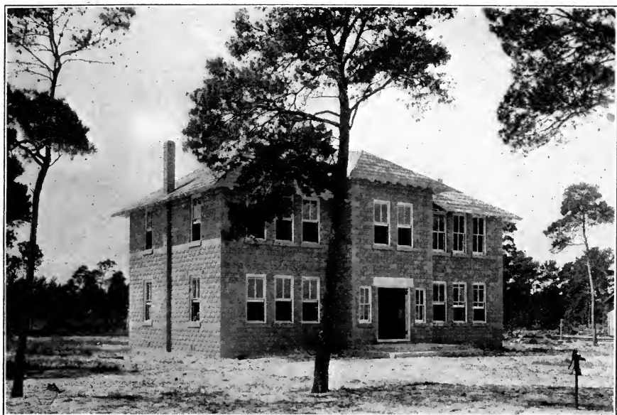
FIG. 10.—CONCRETE BLOCK SCHOOL HOUSE, STUART, FLORIDA.
