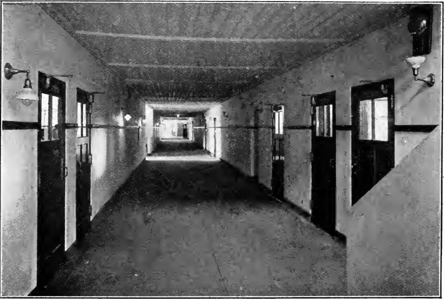
FIG. 3.—CORRIDOR IN NORFOLK HIGH SCHOOL. NO OPPORTUNITY AFFORDED FOR SPREAD OF FIRE.
