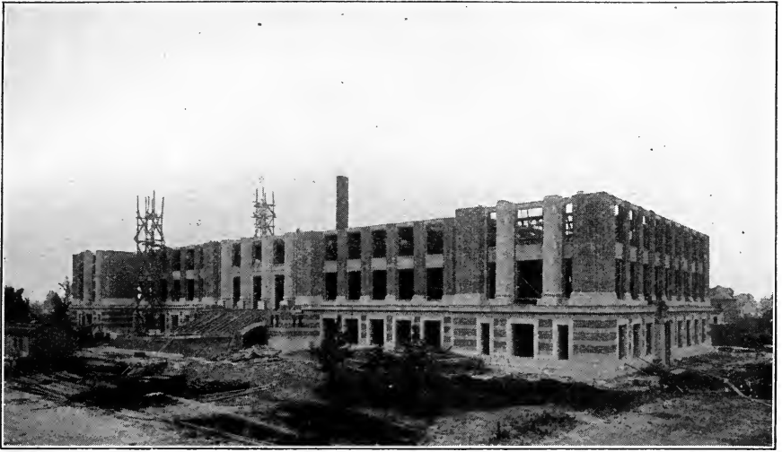
FIG. 8.—NORFOLK HIGH SCHOOL UNDER CONSTRUCTION. REINFORCED CONCRETE SKELETON AND FLOORS WITH BRICK VENEER.
