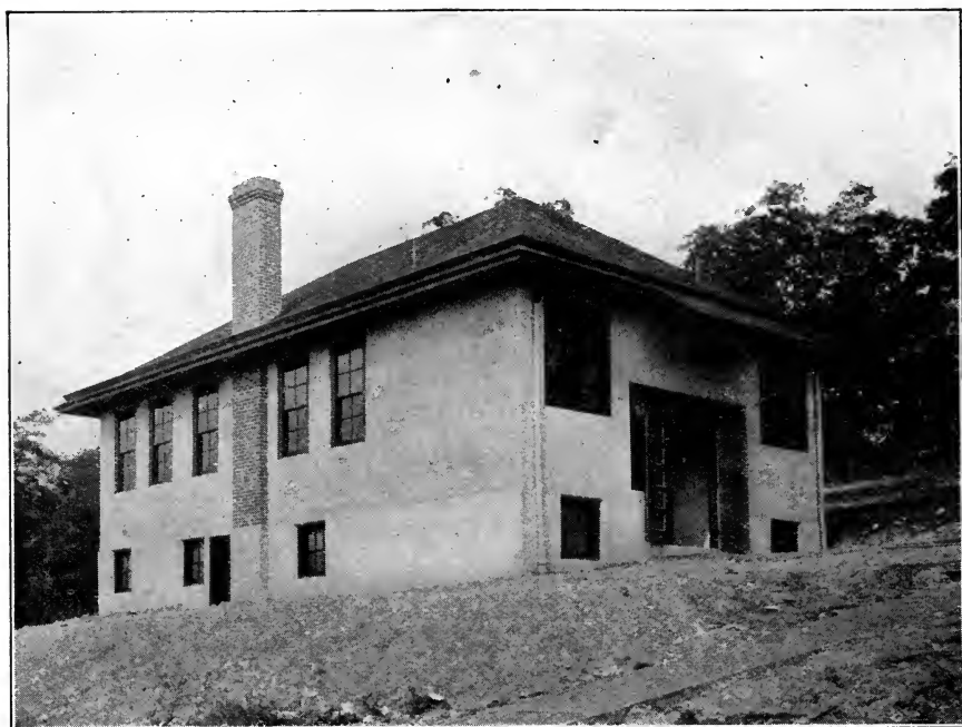
FIG. 7.—ROSLYN FARMS SCHOOL, CARNEGIE, PA. SPLENDID EXAMPLE OF SMALL CONCRETE SCHOOL HOUSE—COST $3,000 COMPLETE.
