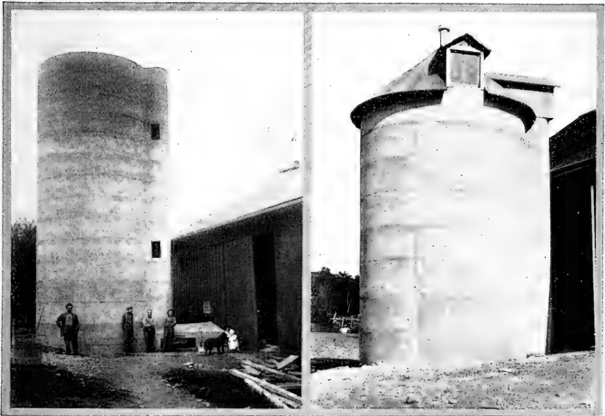
Fifty-foot Concrete Silo put up for Ben. Searls near Picketts, Wisconsin, by George W. Western. Limberg molds used.
