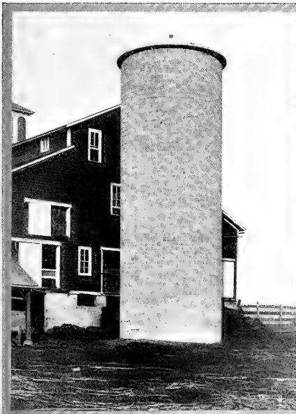
Excellent concrete block silo, built in Iowa by Anchor Concrete Stone Co., Rock Rapids.
