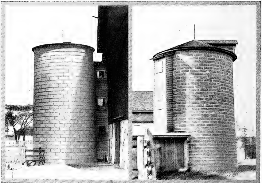
A Michigan Concrete Block silo—homemade—on farm of W. Stoll, Lansing, Michigan.
