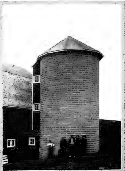
Concrete Block Silo in Minnesota, on G. W. Long's farm at Detroit. Courtesy of Holmes Stone and Lumber Co., Detroit, Minnesota.
