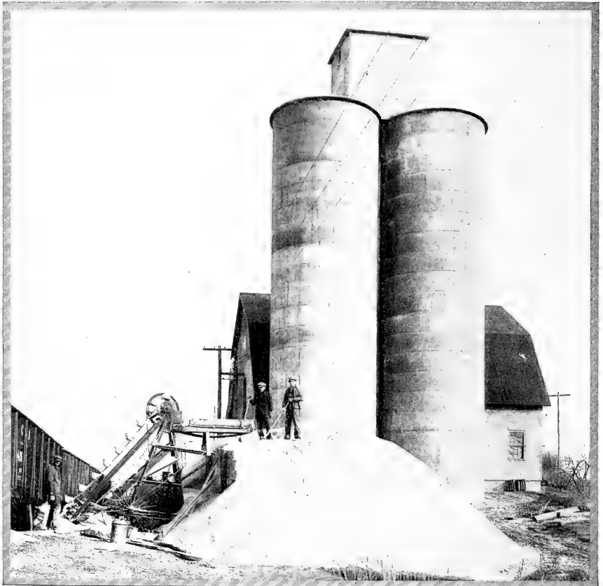
Reinforced Concrete Grain Tanks, 16 feet by 65 feet inside dimensions. Built by Ed. Kuharske, Rockford, Illinois, for Spencer Otis, Sr., Barrington, Illinois. Car unloader shown on side.
