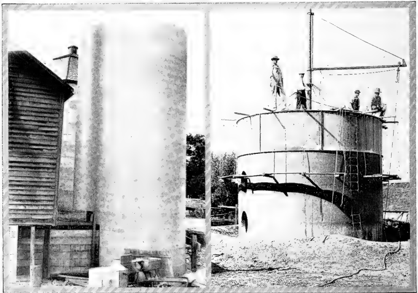
Two Concrete Silos with Concrete Chutes built in Wisconsin with W. A. Limberg's patented molds.
