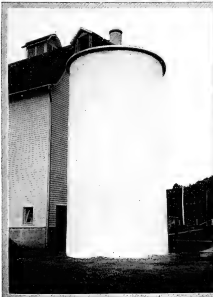
Monolithic Silo 14 feet 3 inches by 40 feet, holding over 200 tons; built by G. A. Ford of Oswego, N. Y., for county.
