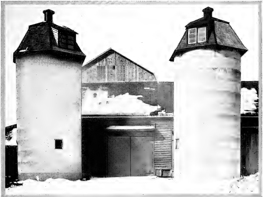
Twin Silos, 14 feet by 40 feet, built for W. Swart of Plymouth, Wisconsin, by W. H. Limberg, silo contractor and inventor of the Limberg Concrete Silo Molds.
