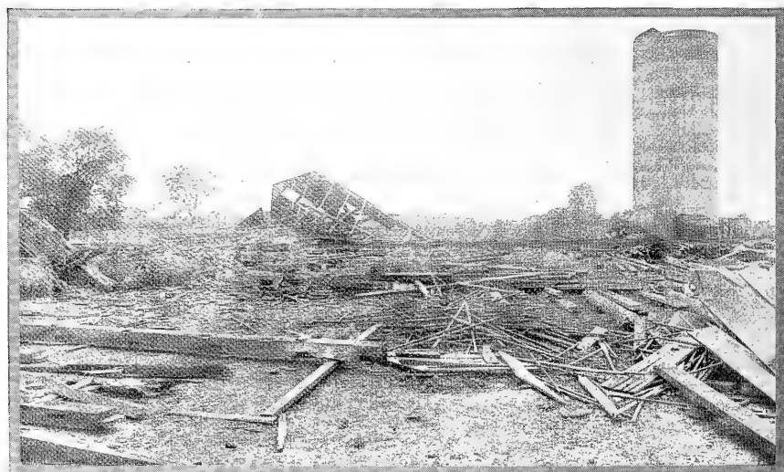
After Cyclone of July 26, 1913, at Frankfort, Kentucky. Eighty-one large barns were blown down. This Polk System concrete silo was undamaged, nor were other concrete silos in the vicinity harmed. "They are not built of pieces and they cannot go to pieces."
