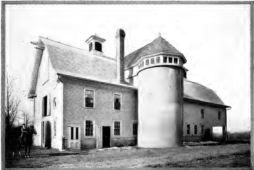
Concrete Silo at Home for the Aged, Washington, D. C.
