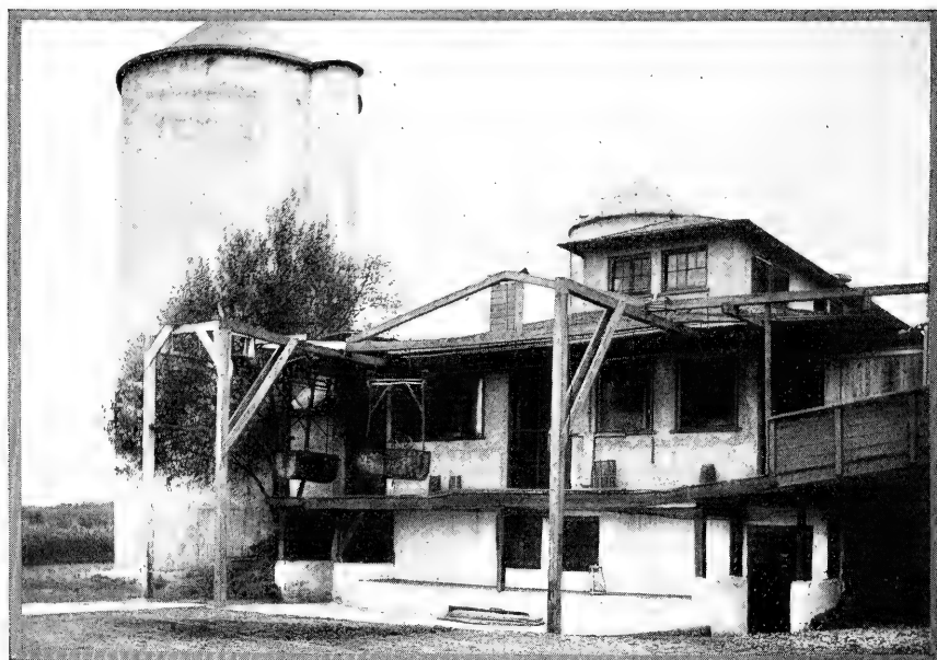
Arcady Certified Milk Barn, Lake Forest, Illinois, showing litter carriers and two of six concrete silos.
