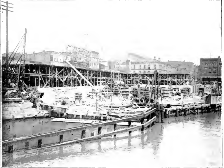
Aug. 1st, Showing Seawall and Adjacent Footings Incomplete.
