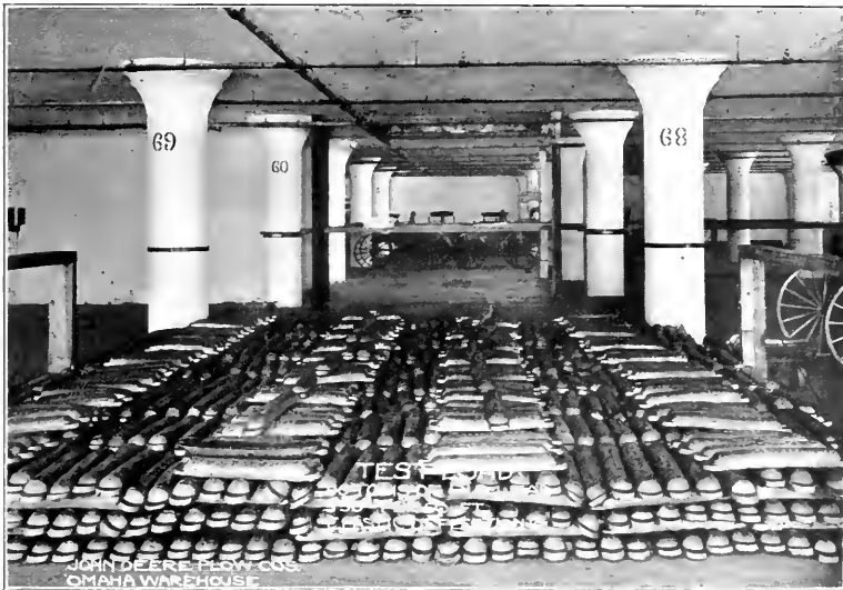
Fig. 18. Test of John Deere Plow Company Building, Omaha, Neb. 550 pounds per square foot.
