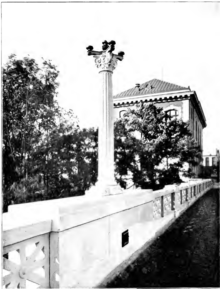
Fig. 97. Cast Stone Railing, bridge at Fergus Falls, Minn. John Lauritzen, Contractor. C. A. P. Turner, Engineer.
