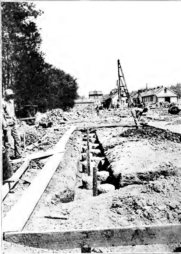
Fig. 91. A Trench Filled with Concrete Piles.
