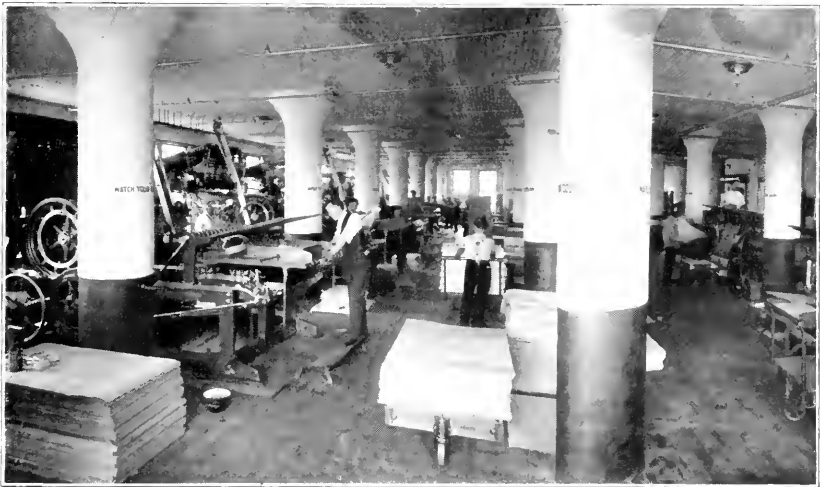
Fig. 10. View showing Ceiling made with Corrugated Steel Forms, Con. P. Curran Building, St. Louis, Mo.
