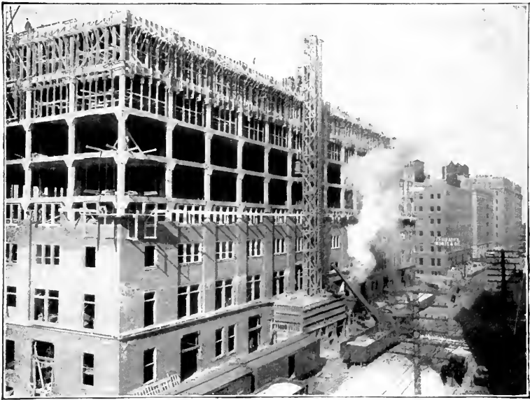
Fig. 2. Mixing Plant and Hopper, John Deere Plow Company Building, Omaha.
