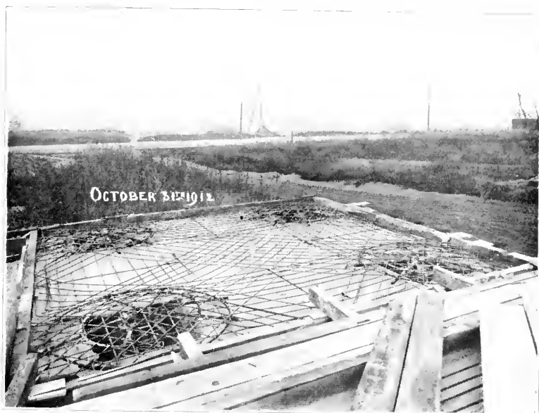
Fig. 65. Reinforcement of Mushroom Slab
