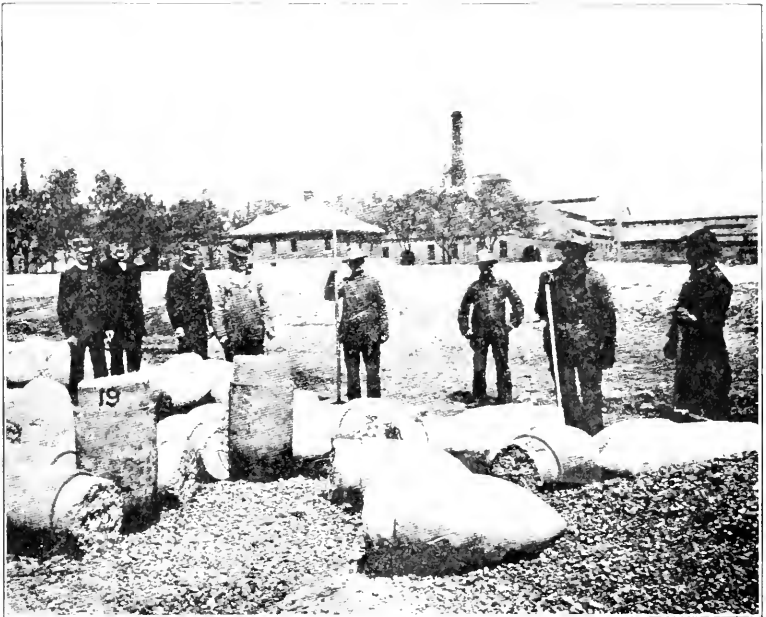
Fig. 87. Concrete Points for Simplex Piles.
