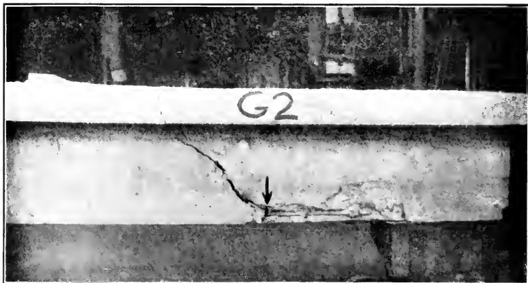
Fig. 31. View Showing Beam Failure by Diagonal Tension near the End.
