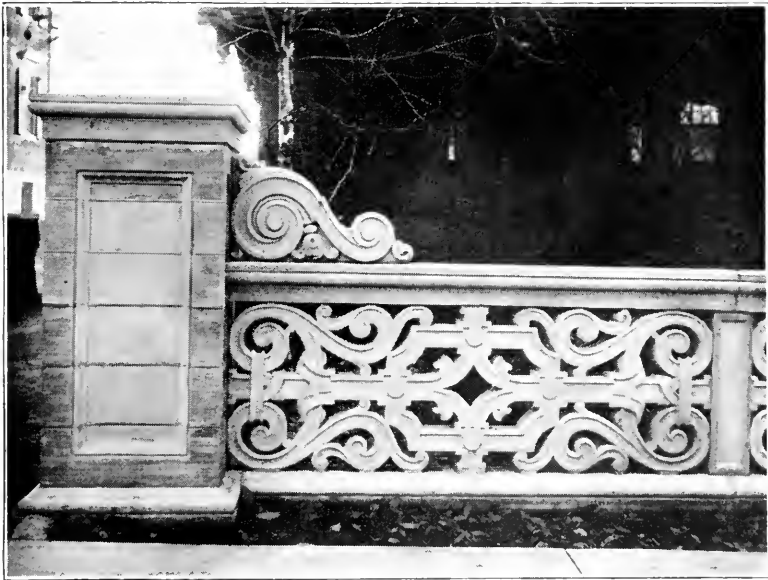
Fig. 98. Ornamental Cast Stone Railing.
