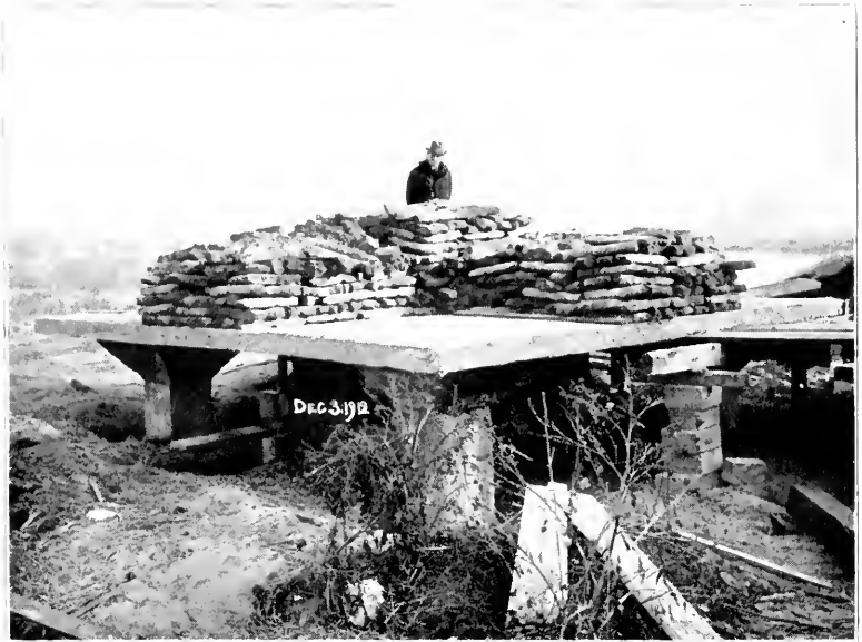
Fig. 67. Mushroom Slab, Load 4.
