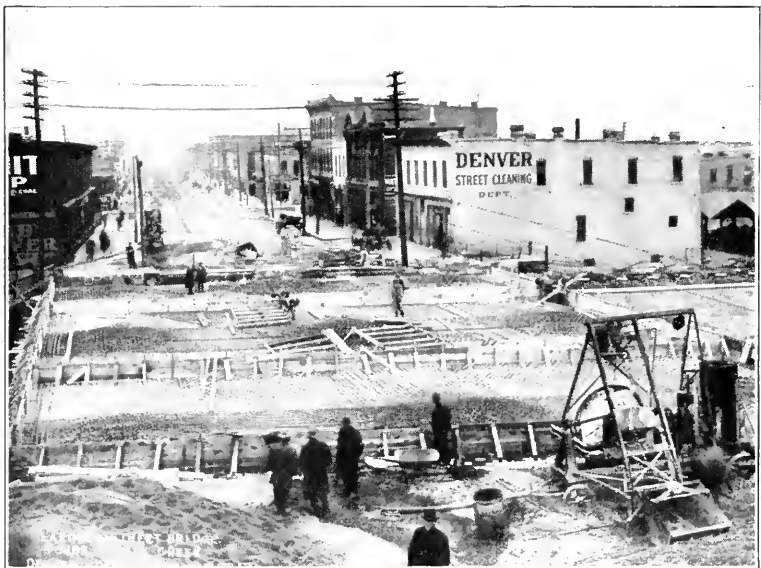
VIEW OF REINFORCING STEEL
