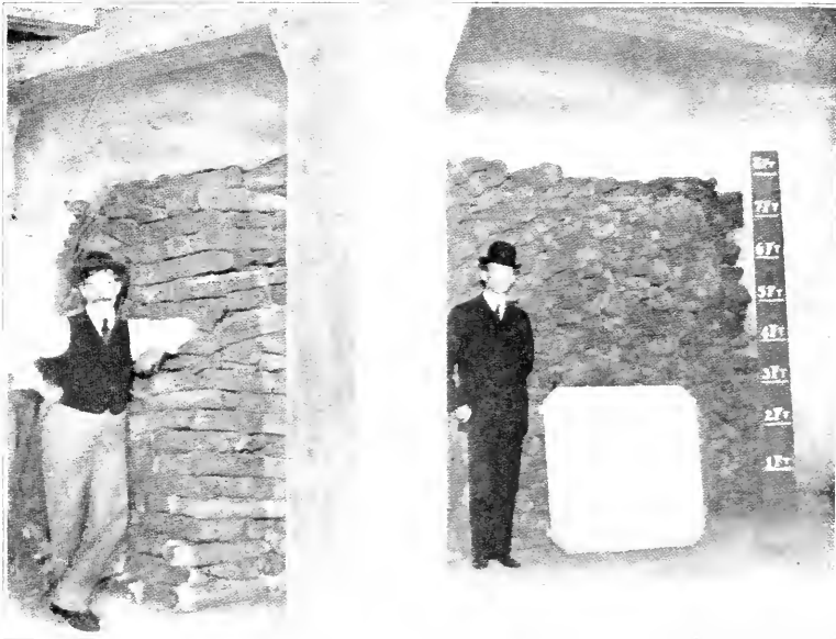
Fig. 41. Test in which Arch Action occurs from Main Beam to Main Beam, giving a Misleading indication as to the Strength of the Floor.
