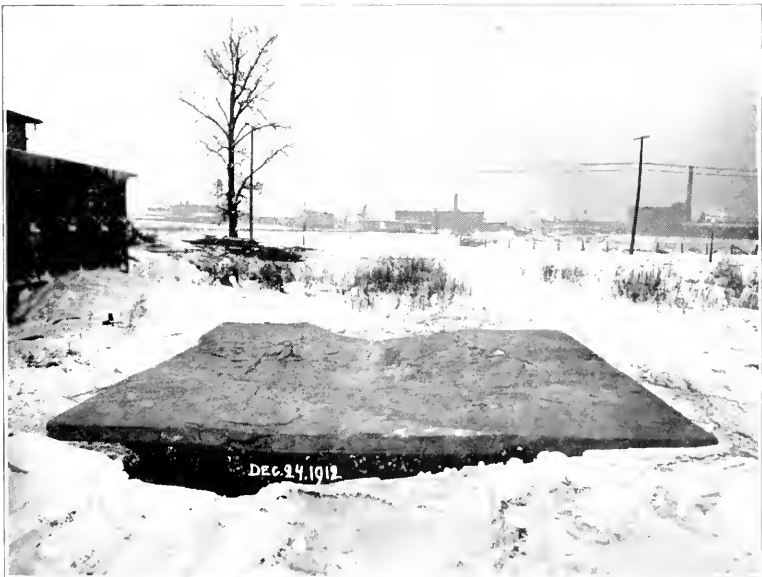
Fig. 72. Failure of Mushroom Slab. Load Removed.
