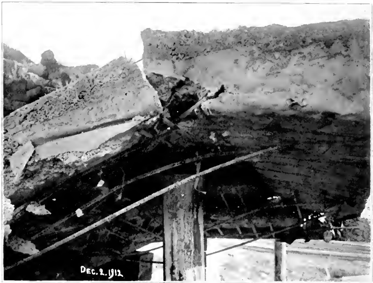
Fig. 64 Collapse of Norcross Slab
