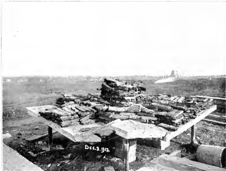
Fig. 63. Collapse of Norcross Slab
