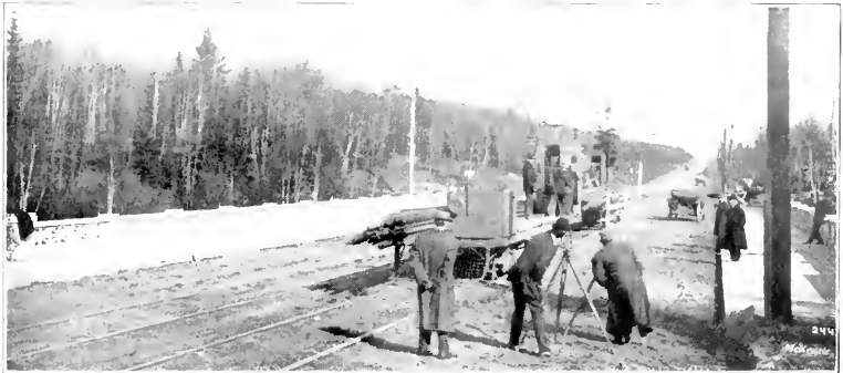
Test of Tischers Creek Bridge with 30 ton construction cars, each loaded with 20 tons of rails Deflection less than one twenty thousandth part of the span
