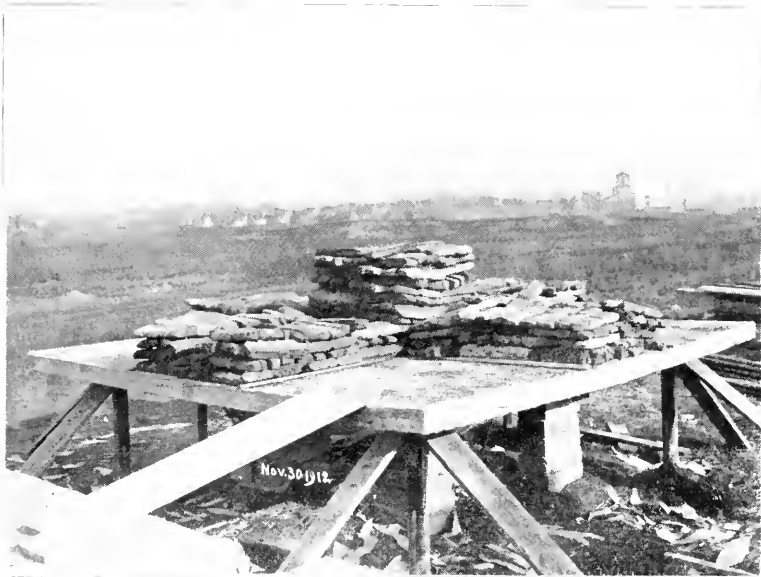
Fig. 61. Norcross Slab Carrying Load 3
