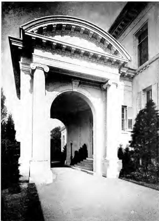
Detail of Guggenheim Residence, Elberon, N. J.
