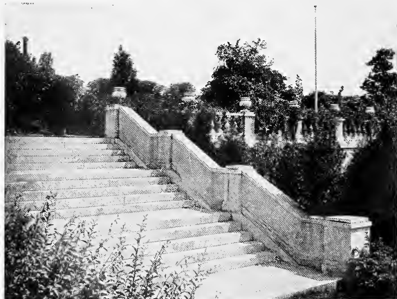
"A high degree of skill is required in casting concrete for steps, sills, copings, balustrades and the like, employed as exterior members in place of stone"
