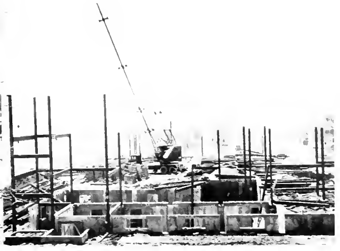
The photographer on April 4 caught the crane swinging the first shipment of steel into place on the foundation. Dimly outlined in the background are the faculty houses on Mount Joy Street.
