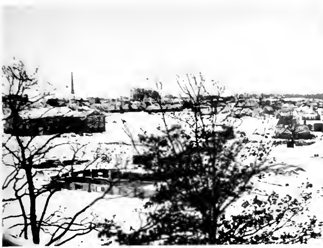
The big snow of the winter on March 17 partially covered the foundation ready for delayed steel. The new Church of the Brethren stands almost completed just beyond the edge of the campus.
