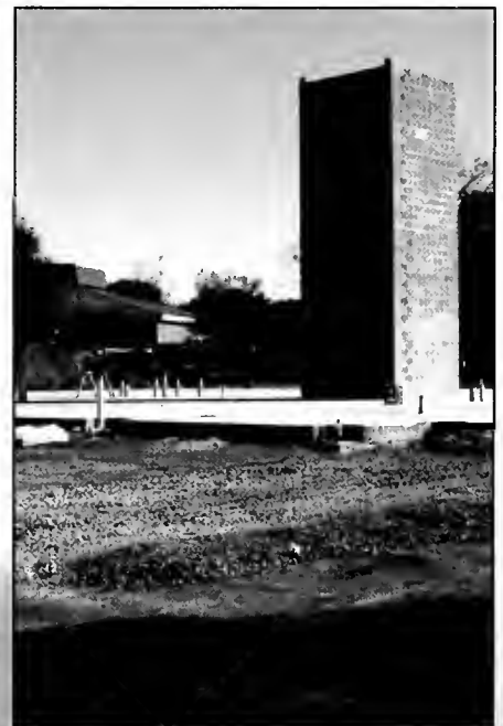
Above: In Early November, the foundation for the building was complete.
