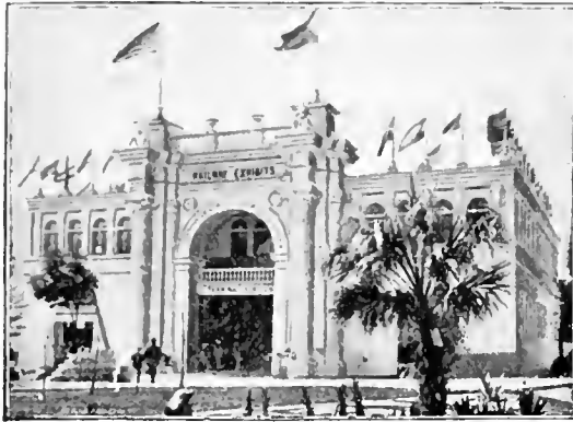
TERMINAL STATION, TENNESSEE CENTENNIAL.
