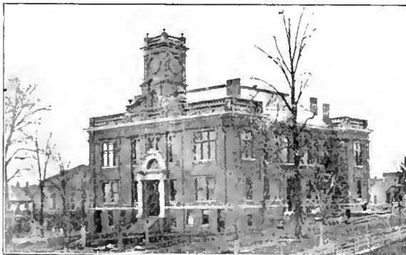
COURT HOUSE, GLASGOW, KY.
