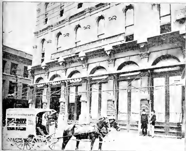
Entrance to store and offices. Entrance to VETERAN office. METHODIST PUBLISHING HOUSE, N. E. CORNER PUBLIC SQUARE.
