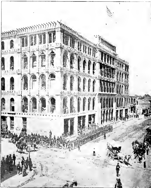
THE MAXWELL HOUSE AT THE TIME OF THE DISASTER.
