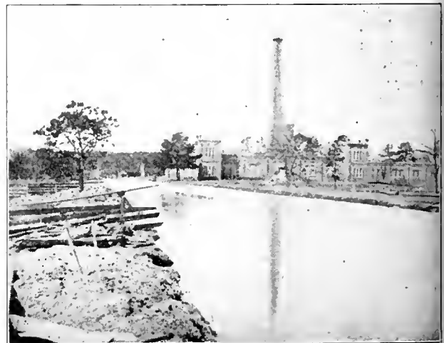
CHIMNEY OF OLD POWDER MILL, AUGUSTA, GA.
