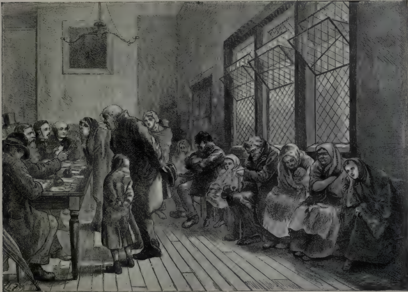
DISTRESS IN THE NORTH.
