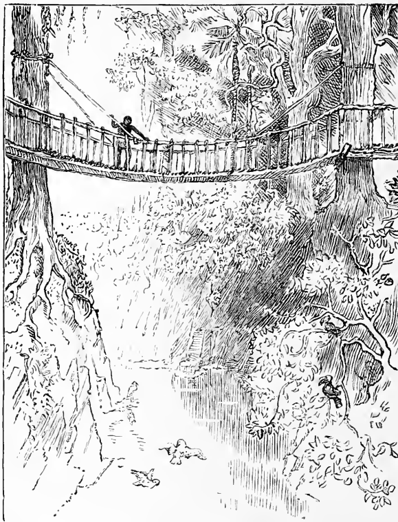
A SUSPENSION BRIDGE.
