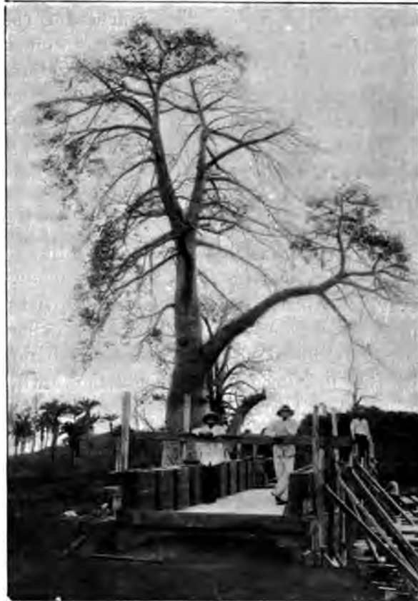
BRIDGE AT BOMA.
