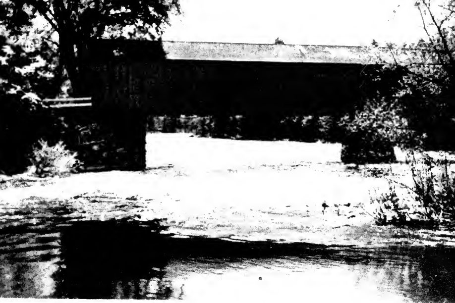
HART'S BRIDGE, WEST CORNWALL
