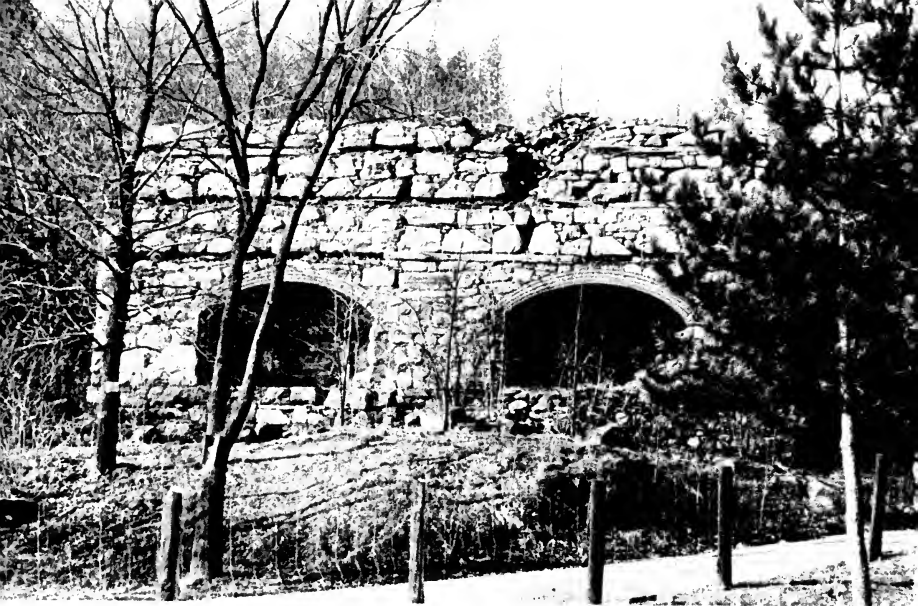
CEMENT KILN, WOODBRIDGE
