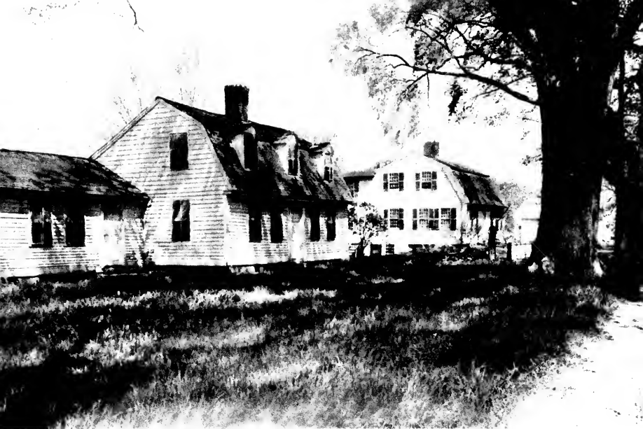
GAMBREL ROOFS, PLAINFIELD
