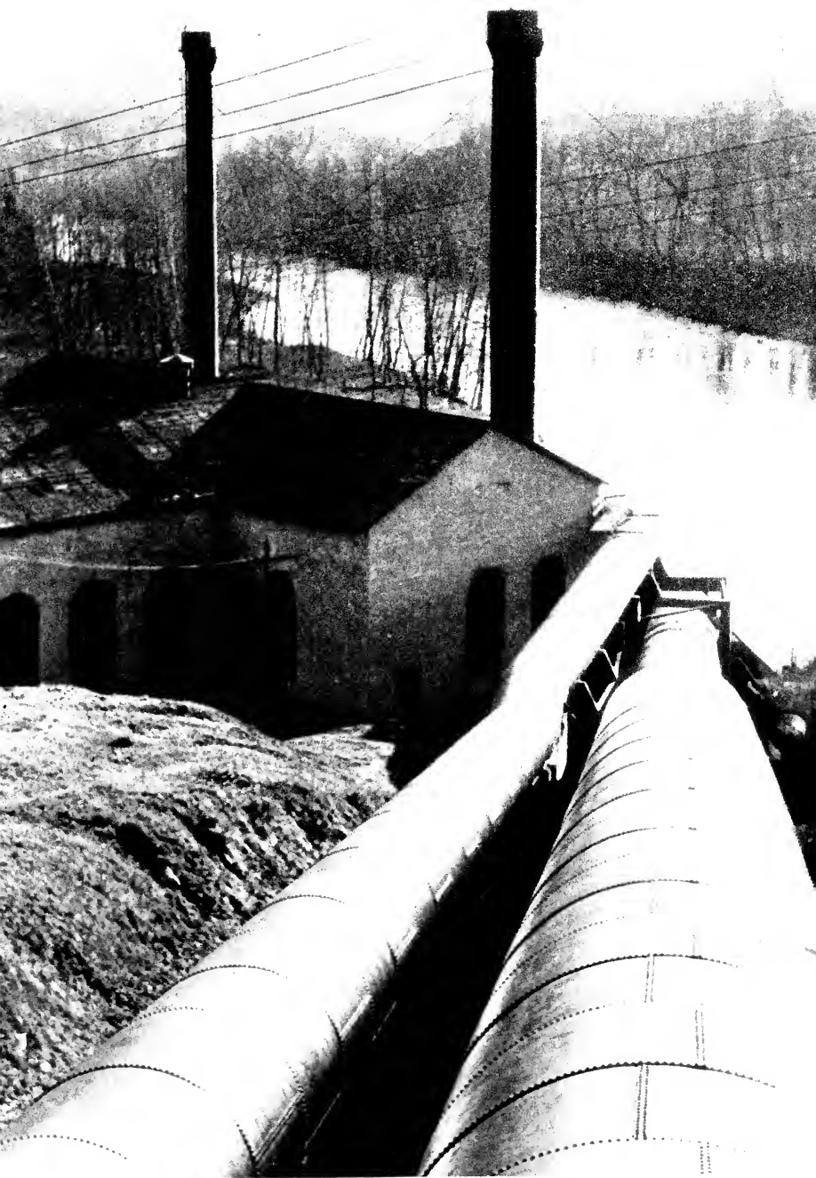
HYDROELECTRIC PLANT, BULLS BRIDGE
