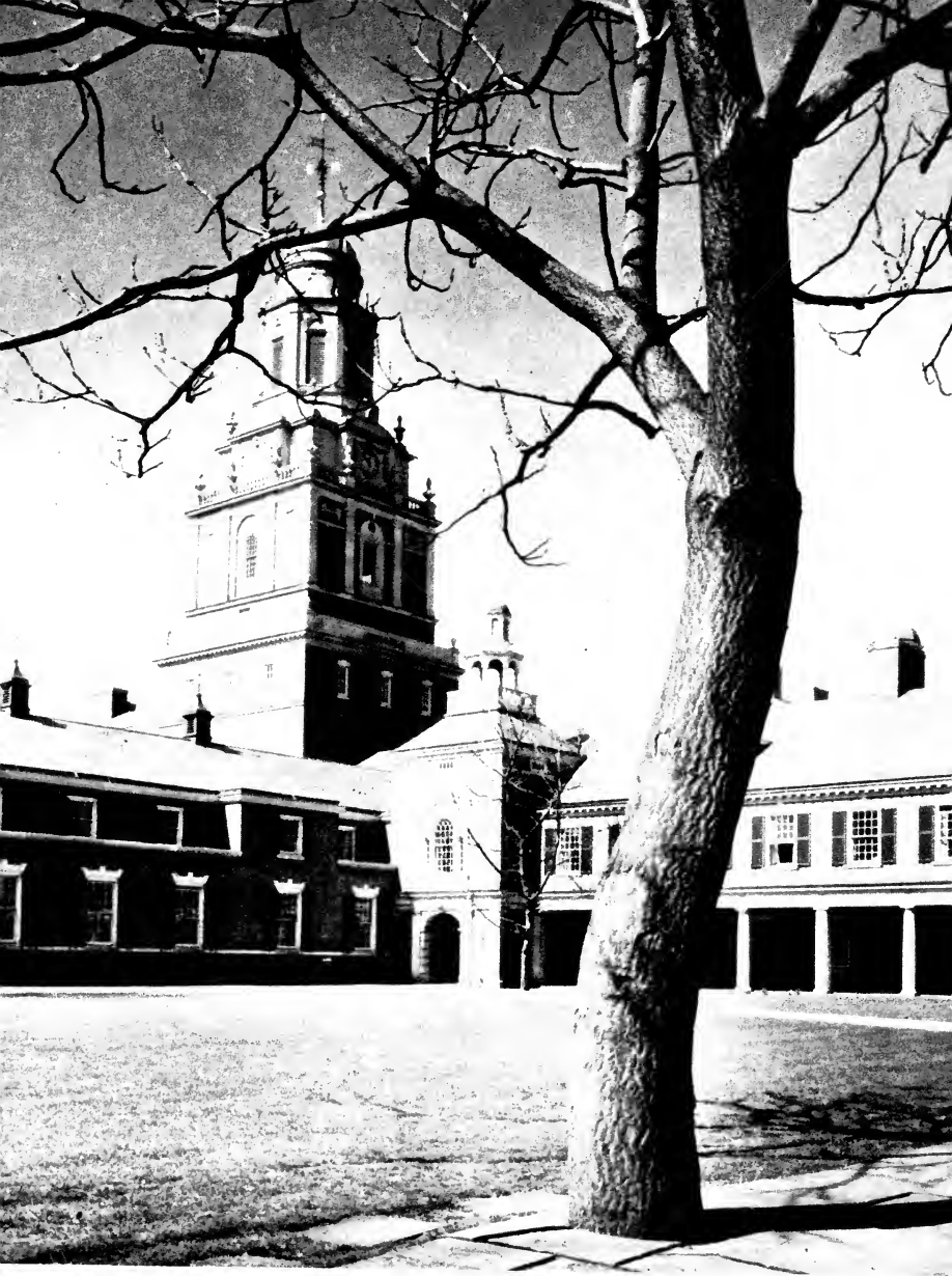
DAVENPORT COURT AND PIERSON TOWER, YALE UNIVERSITY
