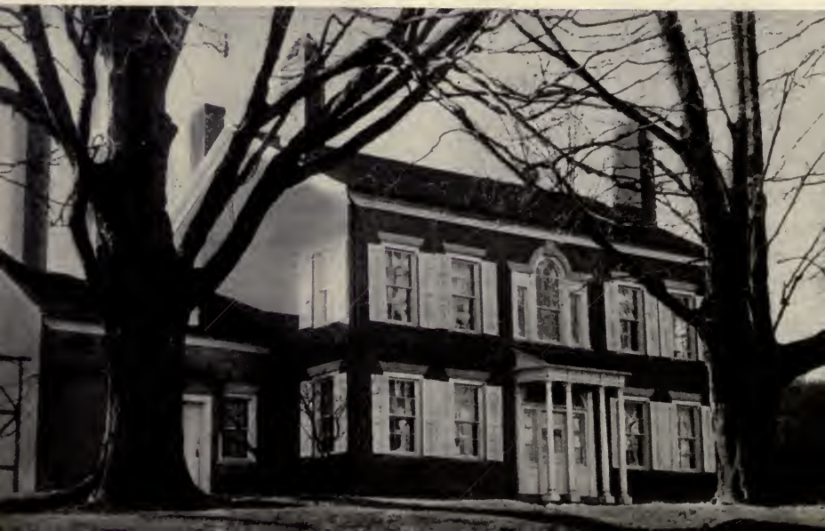
NOBLE HOUSE, NEW MILFORD
