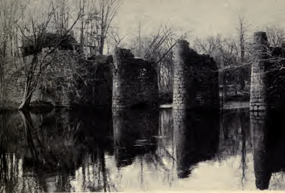
CANAL PIERS, FARMINGTON
